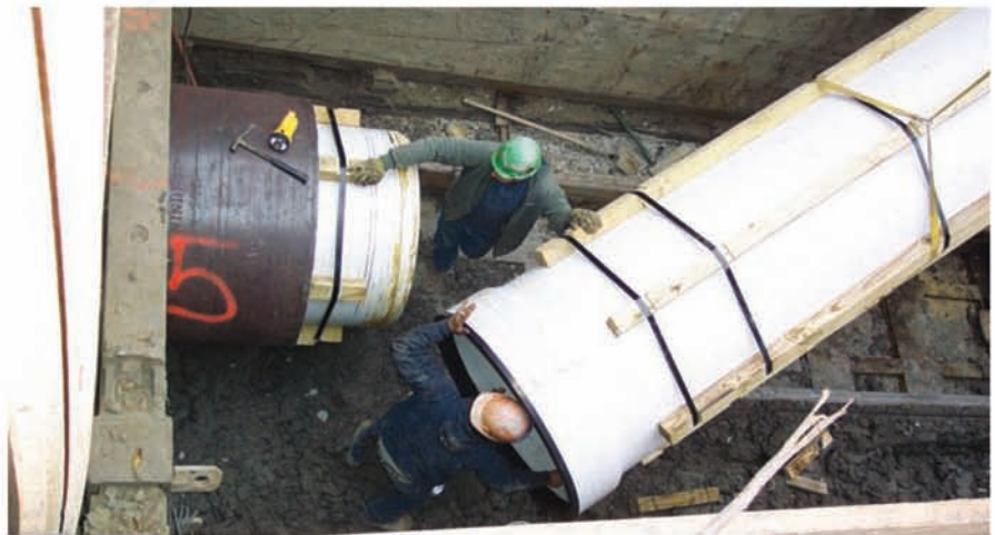
Vylon pipes being connected and inserted into casing pipe for river crossing.
