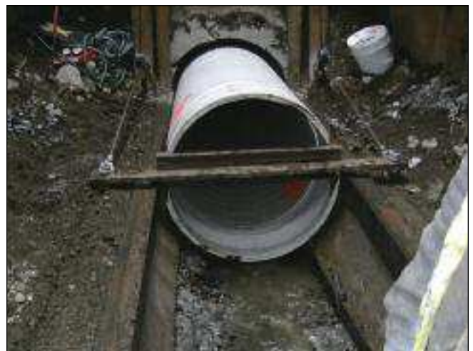
PVC Vylon pipe being installed
