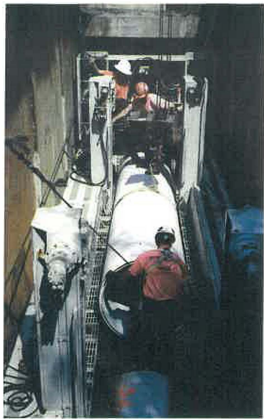
A special sliplining push unit with power for up to 200 tons thrust is employed on the project.
