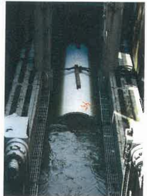
The sewer flows continue uninterrupted at 20 to 80 percent flow capacity during the sliplining process.
