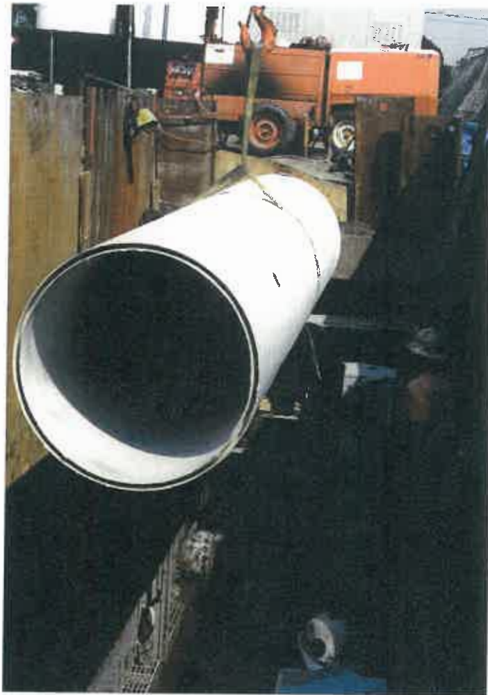
The District 5 Trunk Rehab Project uses 15-ft segments of the 36-in. closed profile-wall PVC sliplining pipe.
