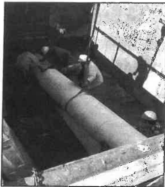
Joint is lined up for quick coupling and insertion.
