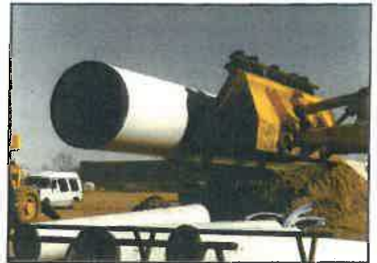
Lightweight, 15-ft. long Vylon Slipline joints are easily handled and staged for insertion.
