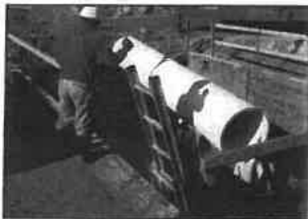
Slipline lowered into shored insertion pit.
