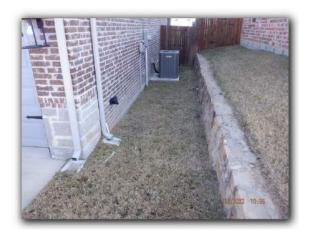
**Notice:** Proper drainage is needed to help prevent water from standing or ponding next to the foundation. There should be a minimum of 4-inches of height from the ground up to the masonry veneer, and a minimum of 6-inches of height from the ground up to any siding material; and there should be a positive slope away from the structure. Corrective measures may be required if water stands within 10-feet of the foundation for more than 24-hours.
