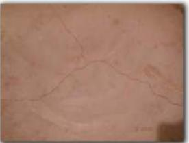
• Stress cracks were observed on the interior of the basement concrete foundation wall in one or more areas; some appear to have been patched or sealed. Recommend further evaluation by a specialist to determine the overall structural condition and concern for possible water intrusion; in need of repair.
