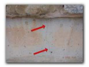
• Cracks were observed in the basement concrete floor of the foundation in several (various) areas; many appear to be greater than common or typical.
