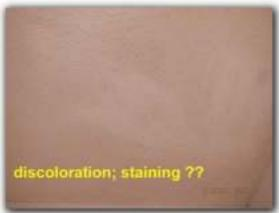
• Water staining and/or leaking was observed on the basement ceiling (insulation) in the small hidden room behind the moveable bookcase at the bottom of the stairs. The cause and remedy should be further evaluated and corrected as necessary.
