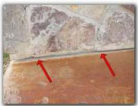
• Visible evidence of previous water intrusion was observed in several areas down in the basement area. Unable to determine the cause and whether the water intrusion came from the exterior, from plumbing related issues, or both. The cause and remedy should be investigated and corrected as necessary.
