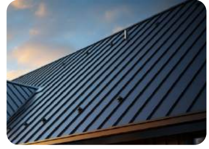
STANDING SEAM METAL ROOF EST: $3,500
