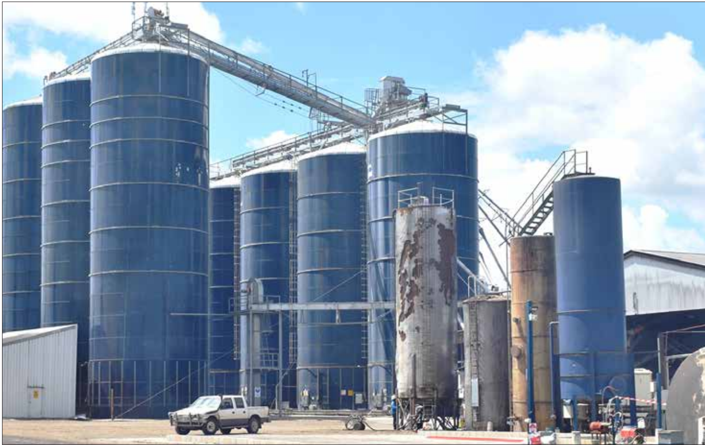
Harvestore silos, heart of the feeding system at Sandalwood, produce high moisture grain which is 20 per cent more digestible than normal grain.
