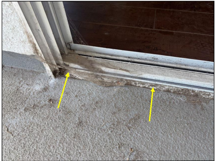
The slider door threshold at the #207 terrace is lower than the surface of the terrace in various places.
