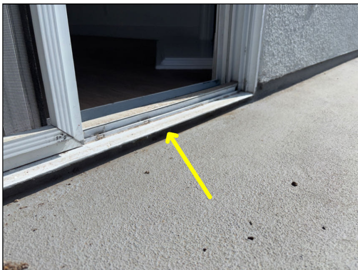
The slider door threshold at the #206 terrace is shown in this image. This is an example of a slider door threshold installed at the proper elevation above the exterior walking surface.
