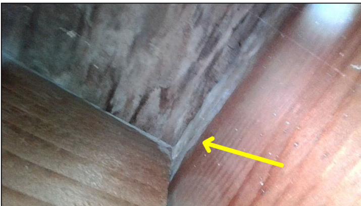
Organic growth was observed at the #203 balcony framing with the baroscope camera.
