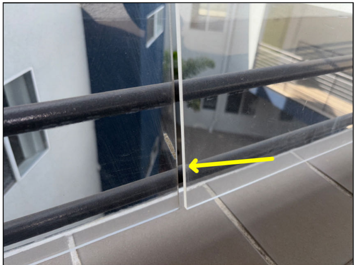
A cracked plastic barrier was noted at the walkway adjacent to #301.
