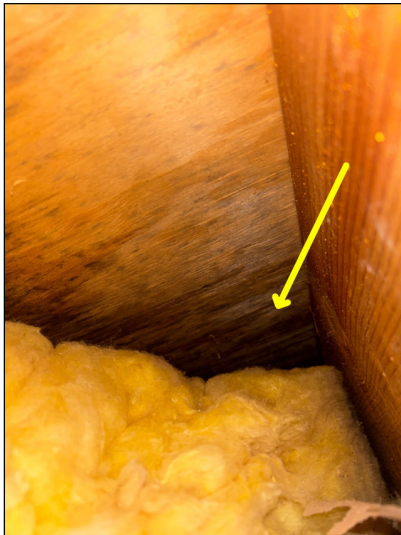
Dry water stains were not noted at the #207 framing where visible at #100.
