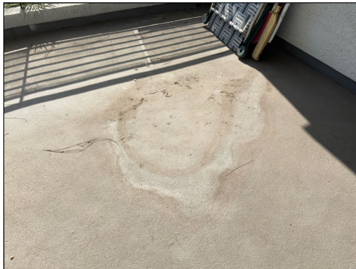
Poor drainage was noted at the surface of the terrace.
