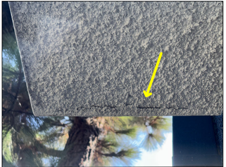
Cracked stucco was noted at the edge of #303 balcony soffit.
