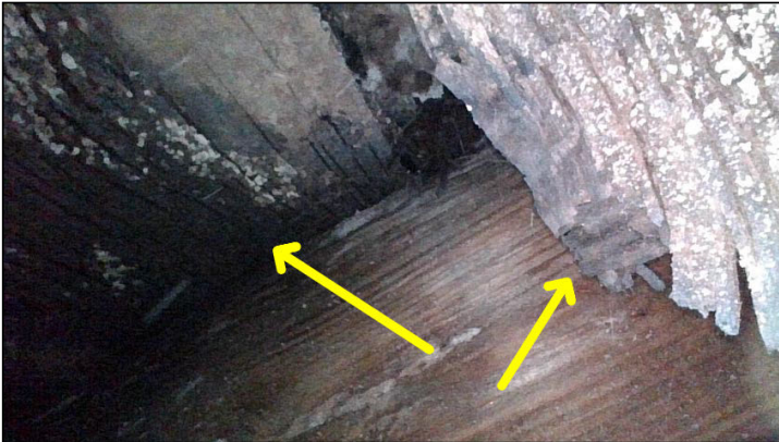
Moisture damage and possible insect damage were observed at the #303 balcony framing with the borescope camera.
