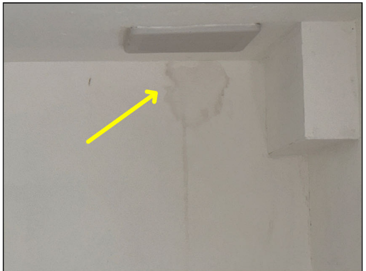
Dry water stains were noted at the #100 ceiling and wall below the #207 terrace.
