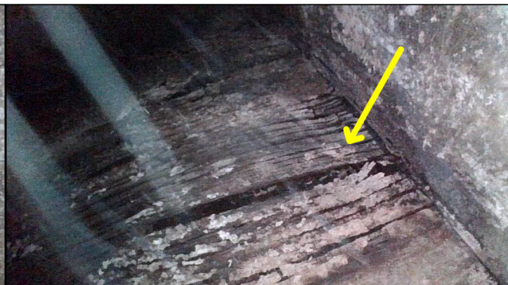
Moisture damage and possible insect damage were observed at the #303 balcony framing with the borescope camera.
