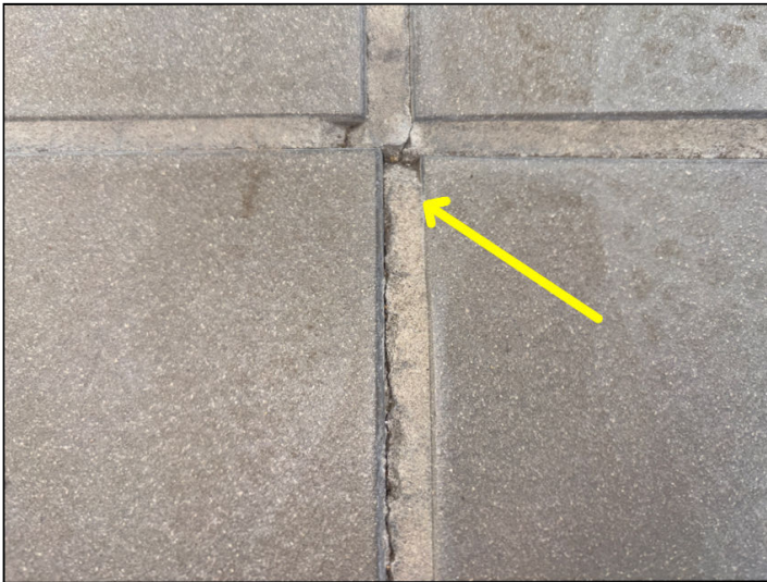
Cracked and missing grout was noted at the walkway surface in various places.
