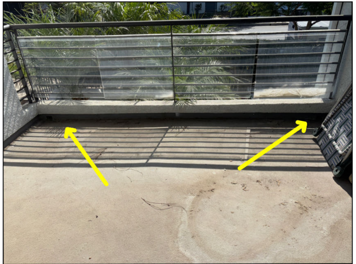
The size and quantity of the #207 terrace drains is not to current standards.
