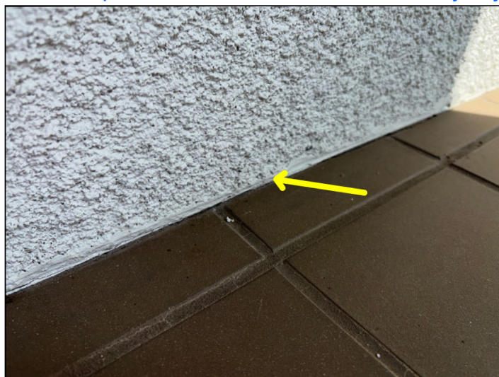
The stucco weep screed is blocked by the tile walkway surface at many places.
