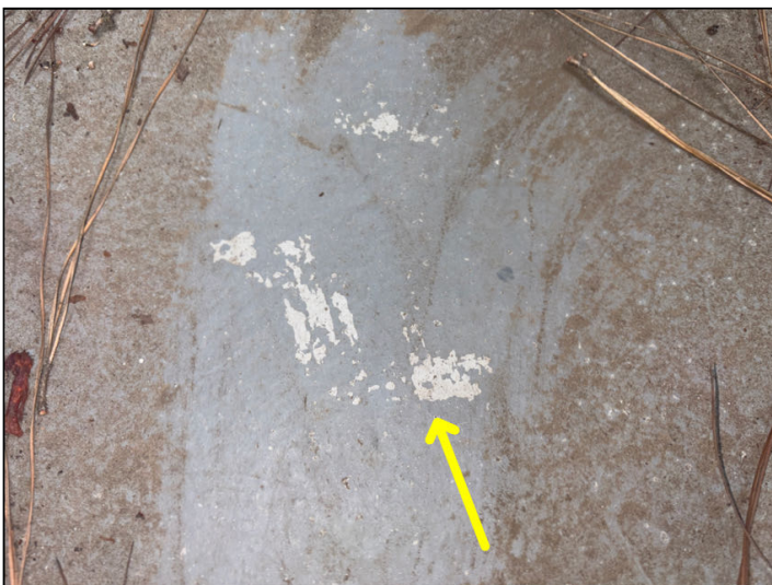
Worn waterproof coating was noted at the #203 and the #303 balcony surfaces.
