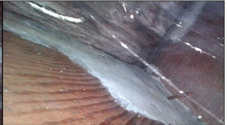
Organic growth was observed at the #203 balcony framing with the baroscope camera.
