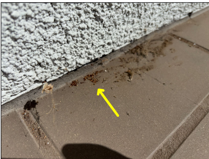
Possible insect droppings were noted at the surface of the walkway in various places adjacent to the exterior walls.
