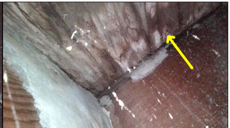
Moisture damage and possible insect damage were observed at the #203 balcony framing with the borescope camera.
