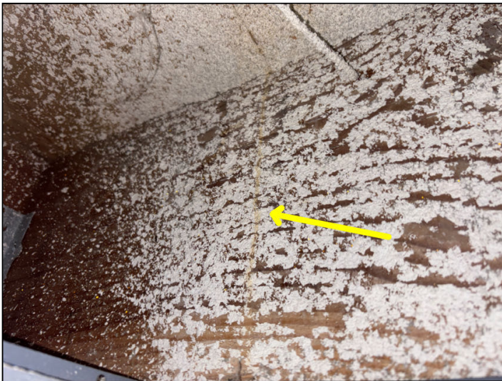
Dry water stains were observed at the walkway framing through plumbing accesses adjacent to #202 and #203.
