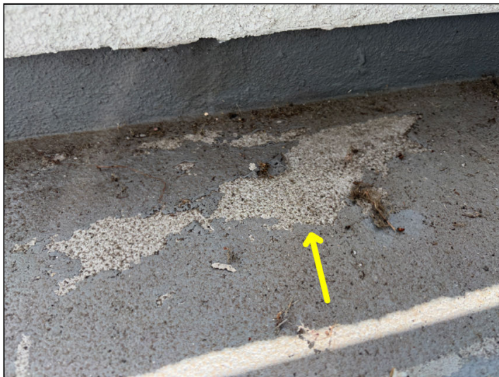
Damaged waterproof coating was noted at the surface of the terrace.
