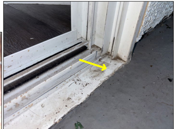
The #203 slider door threshold slopes at the corner of the door.
