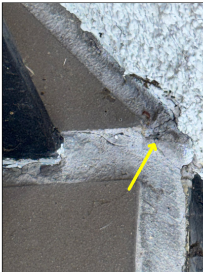
Cracked and missing grout was noted at the walkway surface in various places.
