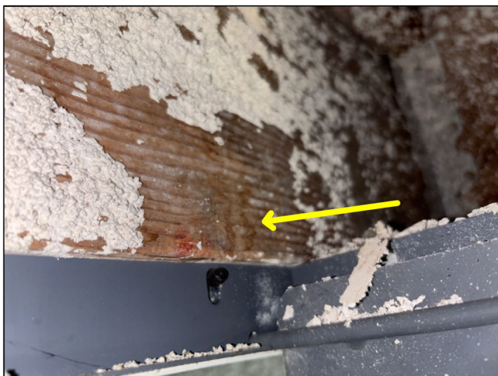
Dry water stains were observed at the walkway framing through plumbing accesses adjacent to #202 and #203.
