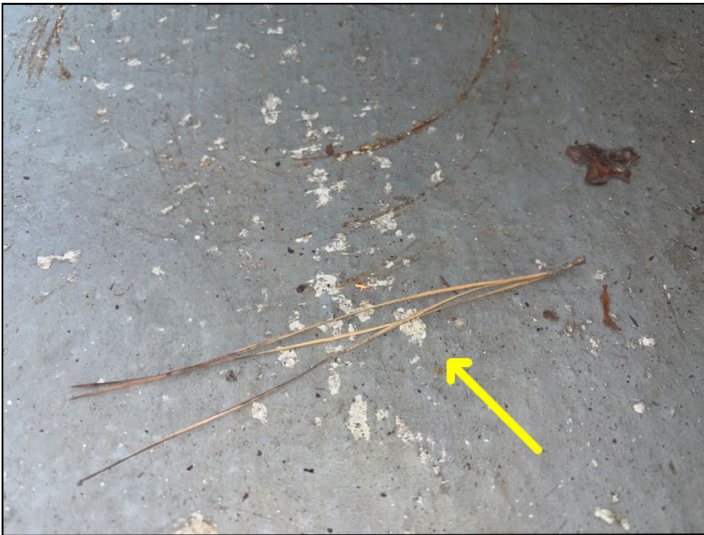
Worn waterproof coating was noted at the #203 and the #303 balcony surfaces.
