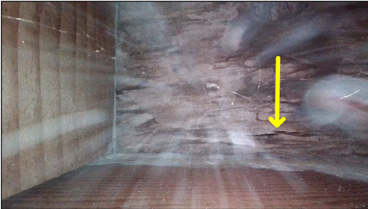
Moisture damage and possible insect damage were observed at the #203 balcony framing with the borescope camera.
