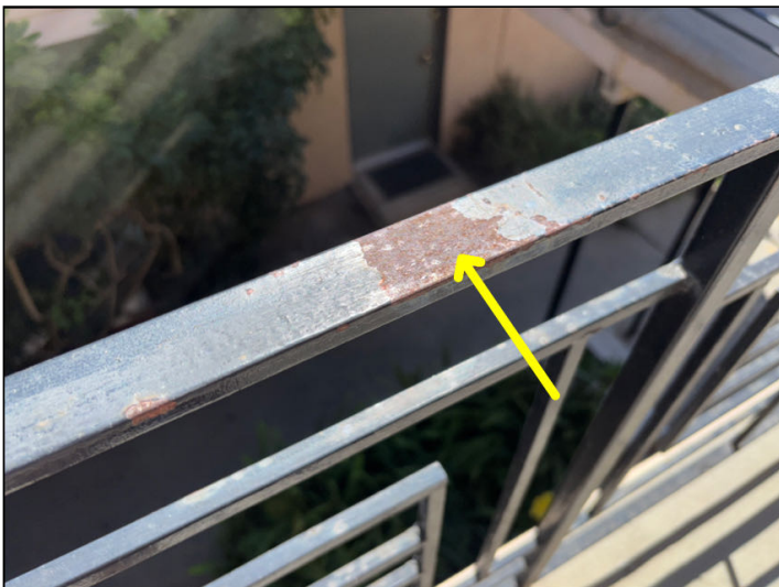
Rust was noted at the walkway guardrails in various places.
