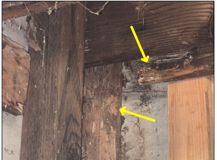
Moisture damage and possible insect damage were noted in many places at the terrace framing.
