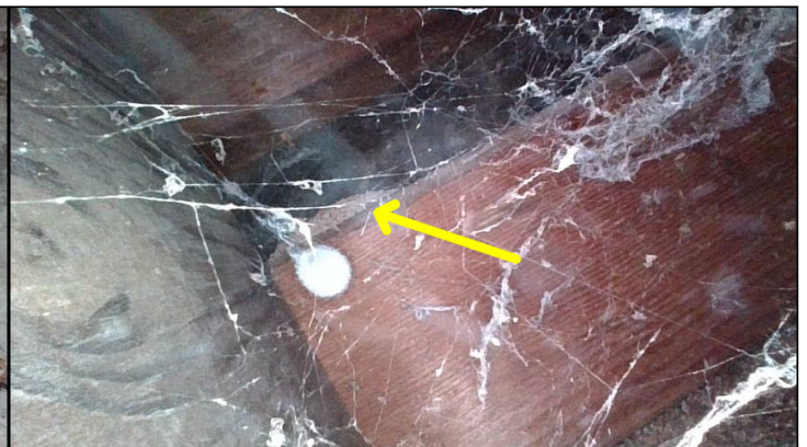
Possible insect droppings were observed in the walkway soffits at many places with the borescope camera.
