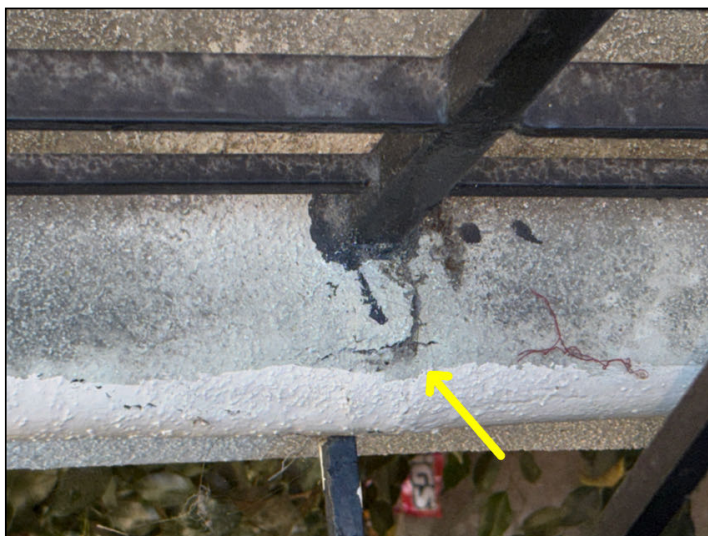
Cracked and uplifted walkway surface material was noted adjacent to #25 and between #29 and #30 at the edge of the walkway.
