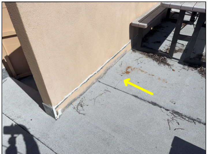
A soft area was noted at the terrace surface adjacent to the stairs.
