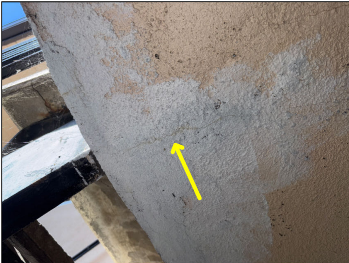
Cracks and slight water stains were noted at the stair landing soffit adjacent to #28.
