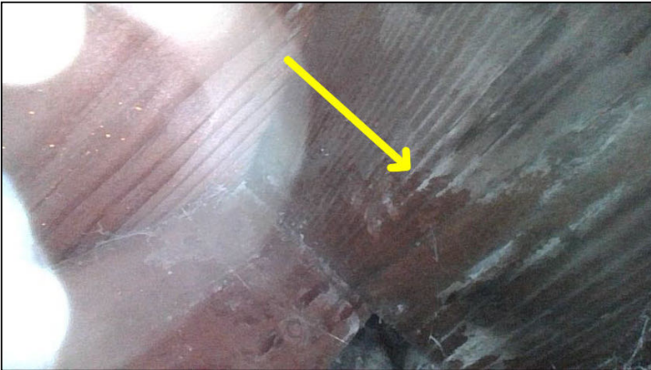
Dry water stains were observed at the walkway framing with the borescope camera in various places including adjacent to #25 and #29.
