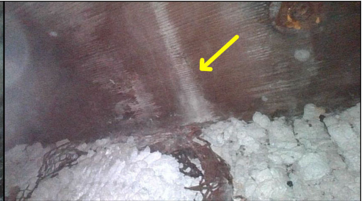
Dry water stains were observed at the walkway framing with the borescope camera in various places including adjacent to #25 and #29.
