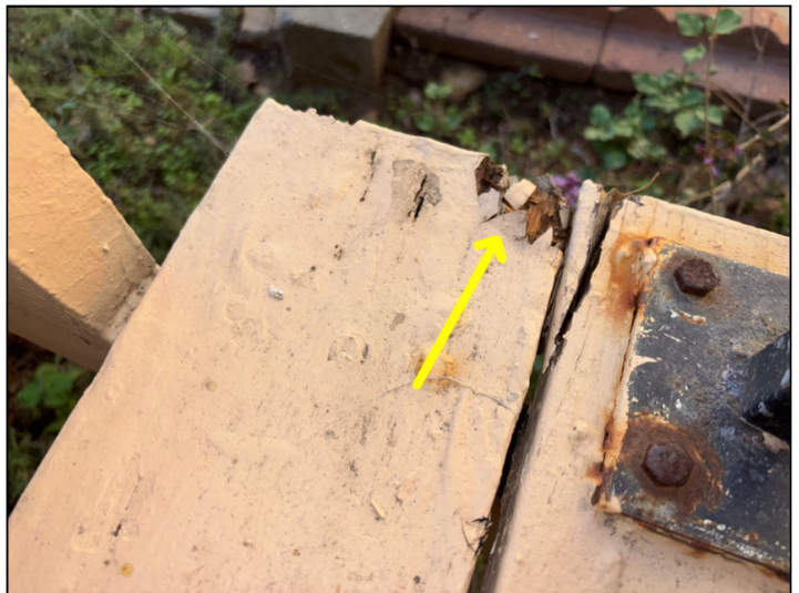
Extensive moisture damage and possible insect damage were noted at the terrace stairs.
