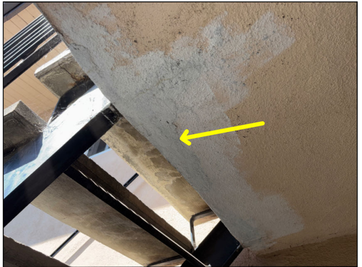
Patching was noted at the stair landing soffit adjacent to #28.
