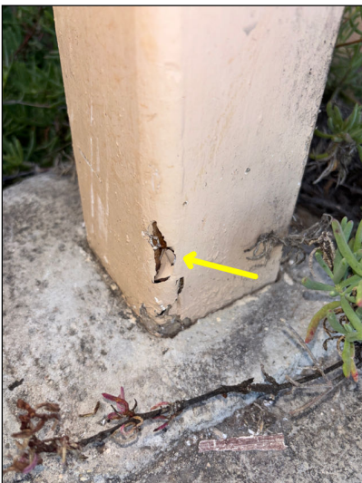
Extensive moisture damage and possible insect damage were noted at the terrace stairs.
