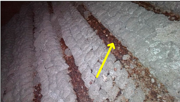
Corroded stucco lathe was observed with the borescope camera adjacent to #6.
