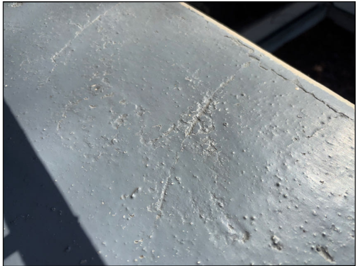
Worn, deteriorated, and cracked waterproof coating was noted at the #33 and #35 balcony surfaces in many places.
