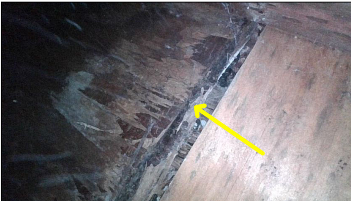
Moisture damage and possible insect damage were observed in various places at the walkway sheathing with the borescope camera adjacent to #29.
