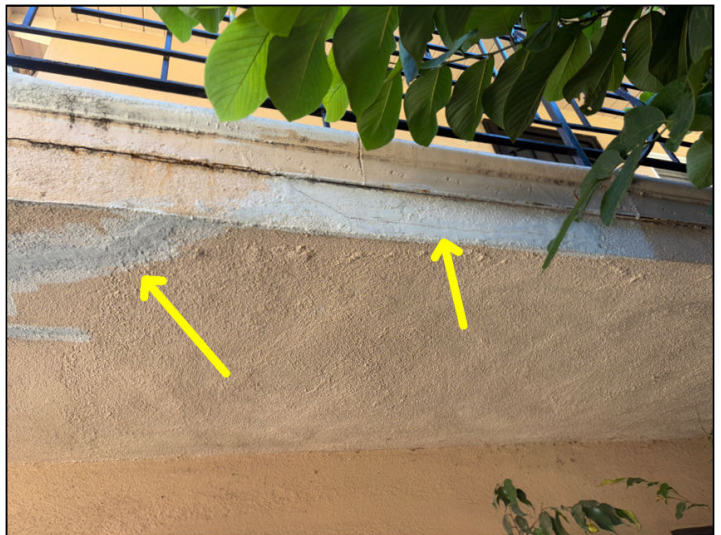
Patching was noted at the walkway soffit adjacent to #29.
