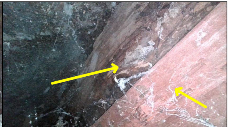
Damaged wood was observed next to newer wood in many places with the borescope camera.
