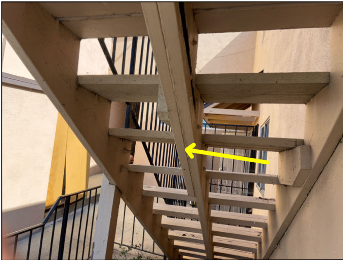
Temporary repairs were noted at the terrace stairs.
