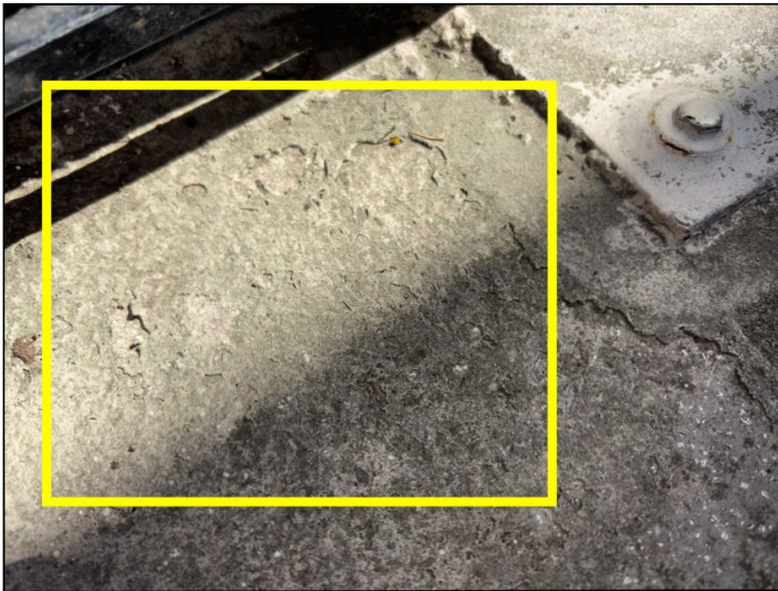
Deteriorated waterproof coating was noted at the walkway surface adjacent to the stairs and #29 in many places.
