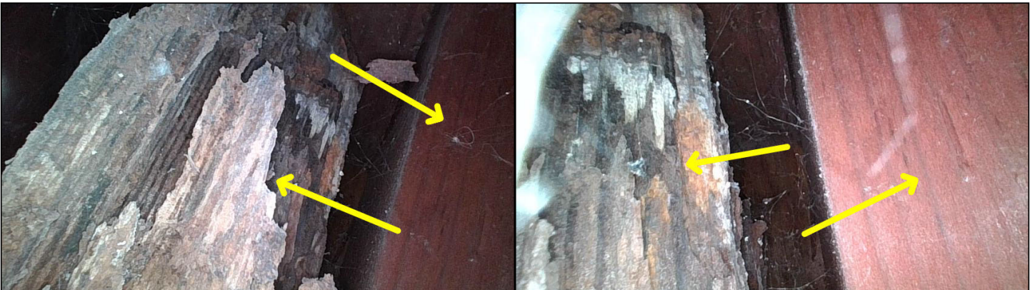
Damaged wood was observed next to newer wood in many places with the borescope camera. Damaged wood was observed next to newer wood in many places with the borescope camera.
