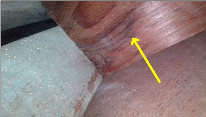
Dry water stains were observed at the #35 balcony framing with the borescope camera.
