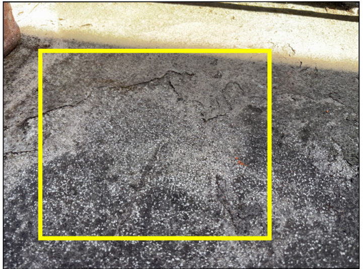
Deteriorated waterproof coating was noted at the walkway surface adjacent to the stairs and #29 in many places.
