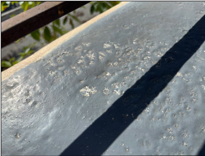
Worn, deteriorated, and cracked waterproof coating was noted at the #33 and #35 balcony surfaces in many places.
