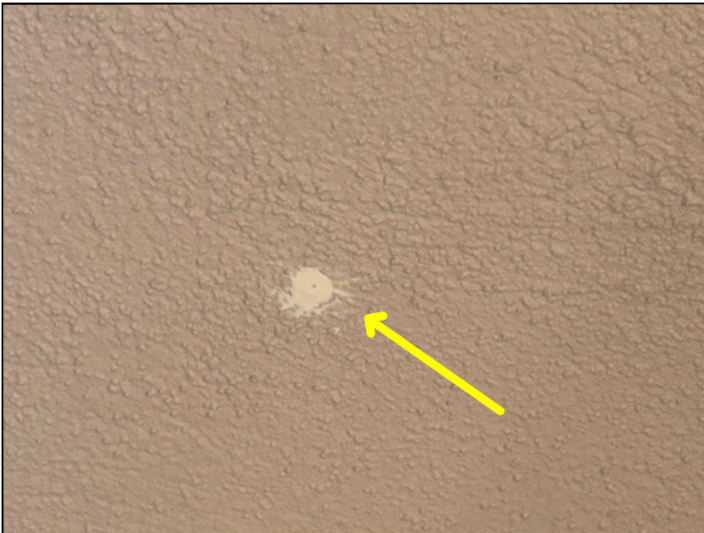
Holes were drilled in the balcony and walkway soffits that were inspected at the time of the inspection to observe the related framing components using a borescope camera.
