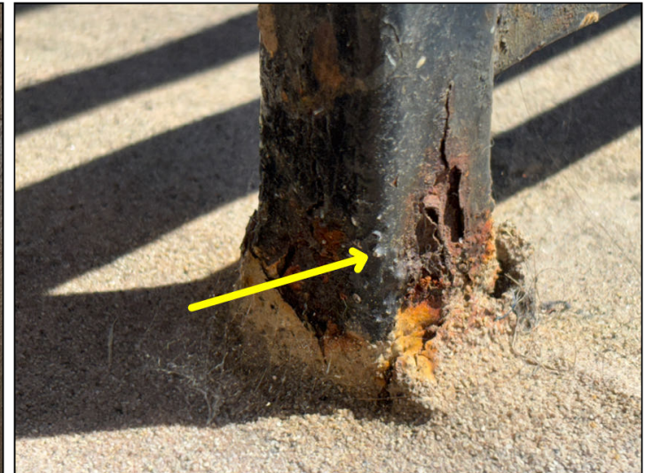
Corrosion was noted at the stair railing post adjacent to #28.
