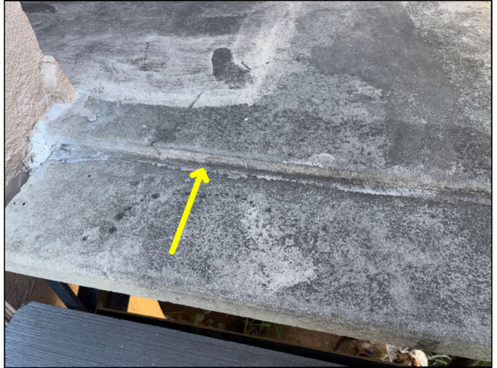
A trip hazard was noted at the edge of the walkway adjacent to the stairs and #29.
