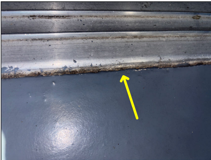
A gap was noted between the balcony surface and the slider door threshold at #33.
