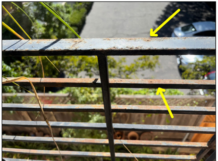
Rust was noted at the balcony guardrails in various places.
