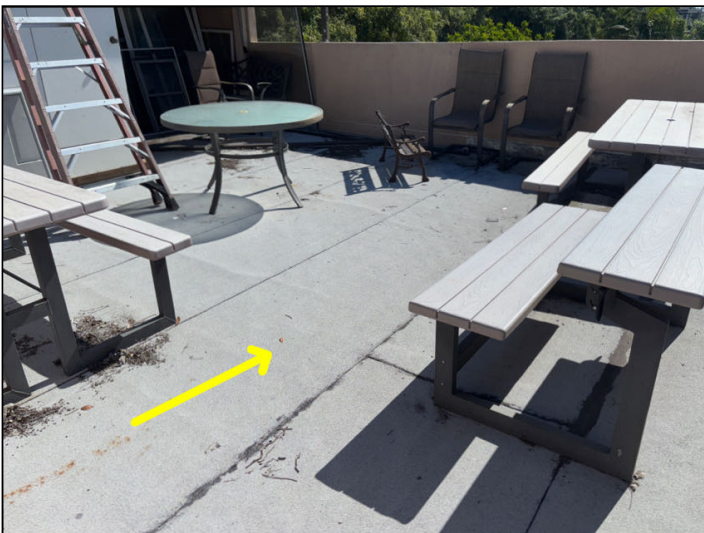
The surface of the terrace is rolled composition roof material.
