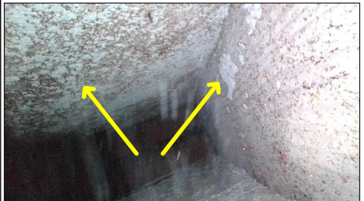
The #31 balcony framing within the soffit was mostly not visible with the borescope camera due to stucco overspray.
