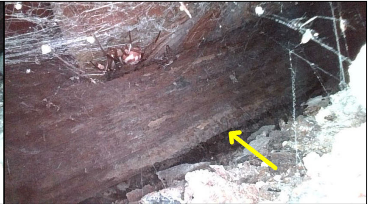
Moisture damage and possible insect damage were observed in various places at the walkway framing with the borescope camera adjacent to #29.
