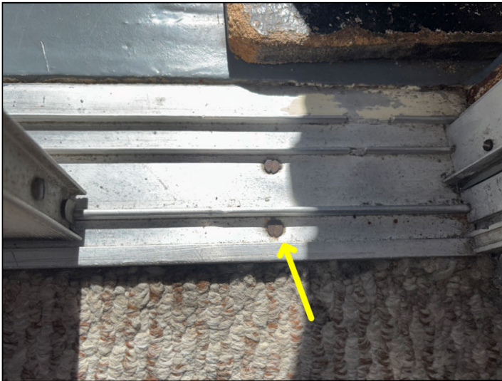
Fasteners have been installed through the #33 balcony slider door threshold.
