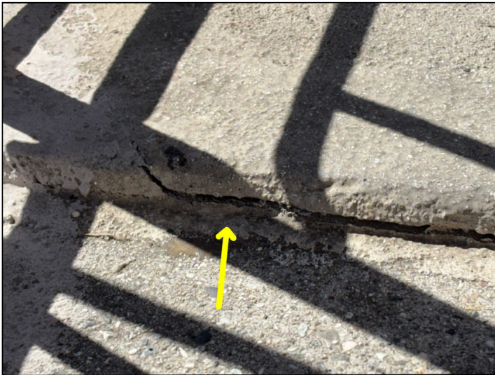
A crack with uplifted material was noted at the walkway adjacent to the #25 stairs.
