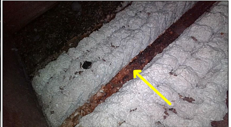
Corroded stucco lathe was observed with the borescope camera adjacent to #6.
