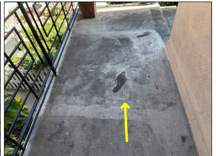
Patching was noted at the walkway surface in many places.
