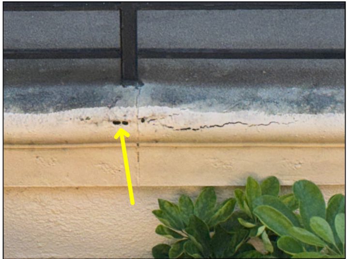
Open cracks were noted at the edge of the walkway between #29 and #30 and adjacent to #25.
