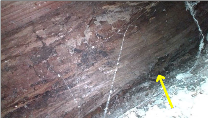
Moisture damage and possible insect damage were observed in various places at the walkway framing with the borescope camera adjacent to #29.
