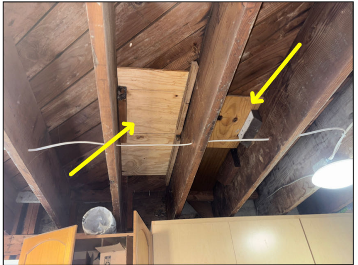
Temporary repairs were noted at the terrace framing.
