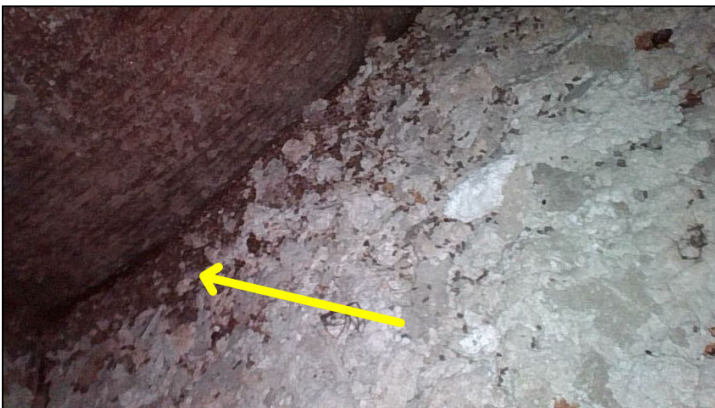
Possible insect droppings were observed in the walkway soffits at many places with the borescope camera.
