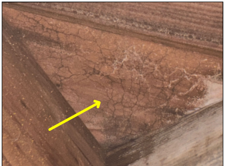
Organic growth was noted at the terrace framing in many places.
