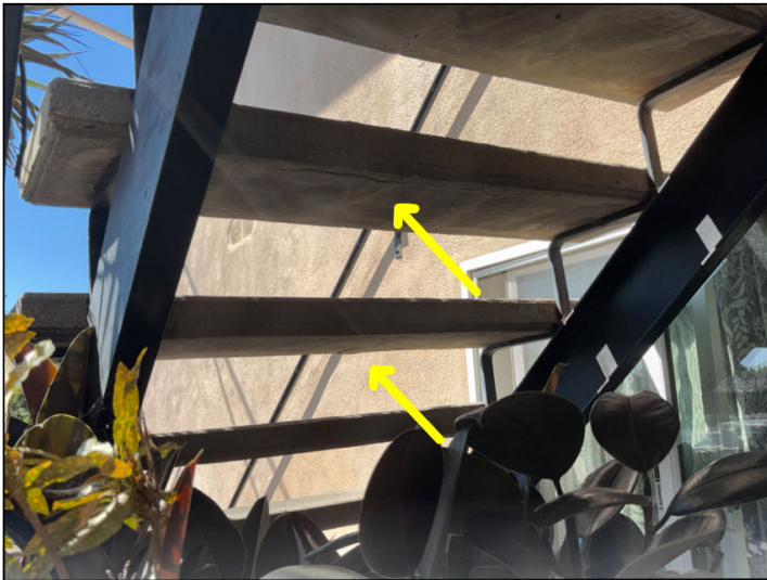
Cracked concrete was noted at the #28 stair treads in various places.
