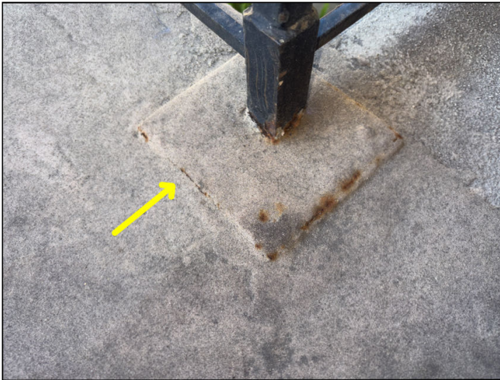
Cracked waterproof coating and rust stains were noted at the walkway surface adjacent to a guardrail post and #30.
