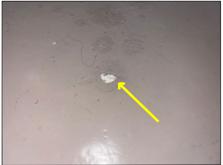
Chipped waterproof coating was noted at the #31 balcony surface.
