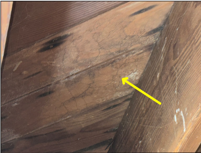
Organic growth was noted at the terrace framing in many places.
