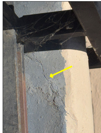
A crack was noted at an area that was patched at the #33 balcony adjacent to a railing post.
