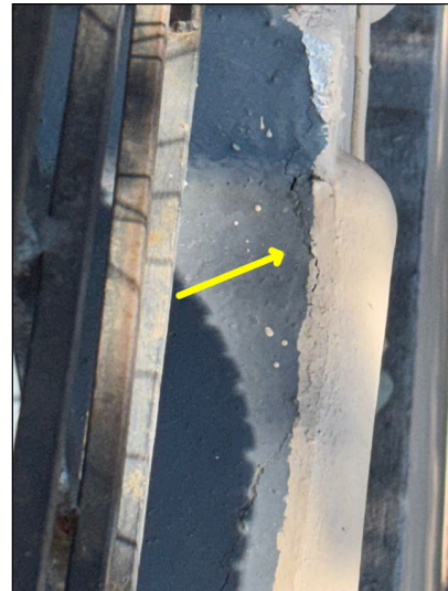
The material at the surface of the balcony is cracked in various places at the #31, #33, and #35 balconies.
