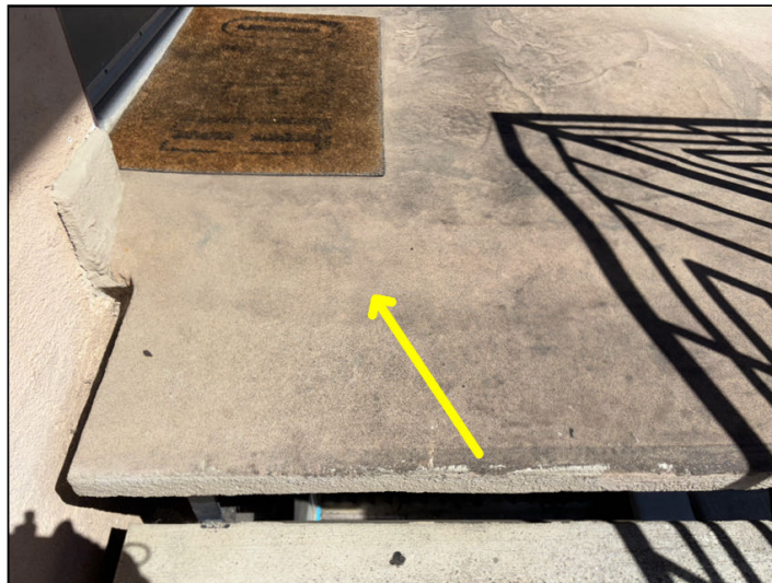
The walkway surface is uneven at the upper stair landing adjacent to #28.
