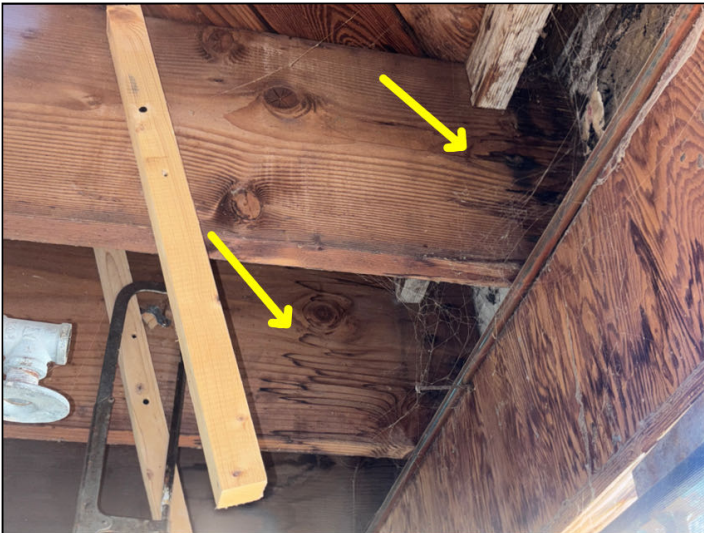
Dry water stains were noted at the terrace framing in many places.
