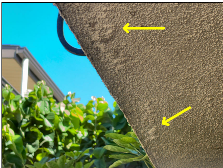
Bubbled paint and efflorescence were noted at the ends of the walkway soffit adjacent to #29 and #30.
