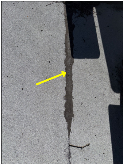
Patching was noted at the rolled composition terrace surface.
