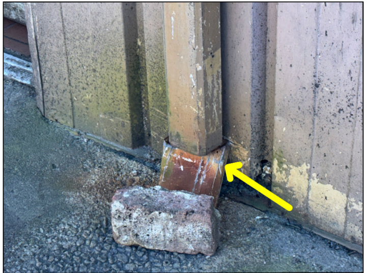
A damaged downspout termination was noted at the rear of 12308.
