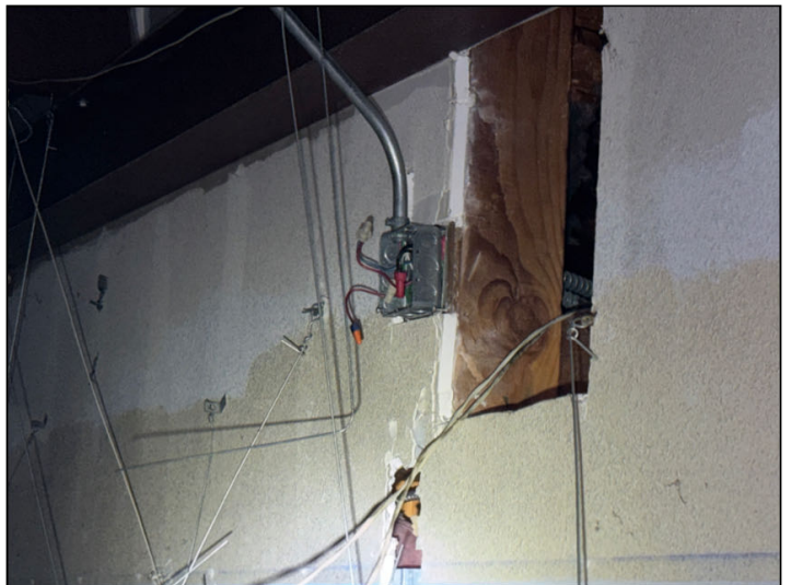
An open junction box was noted in the attic over the side exterior door of unit 12300.
