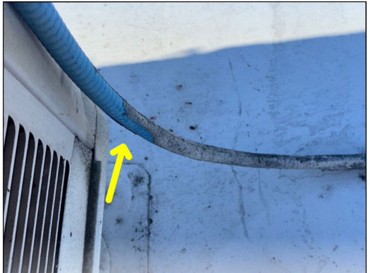
Deteriorated conduits were noted in various places on the roof of 12308.
