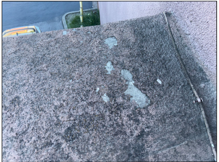
Peeling paint and deteriorated stucco was noted in many places at the horizontal surfaces of the parapet walls.
