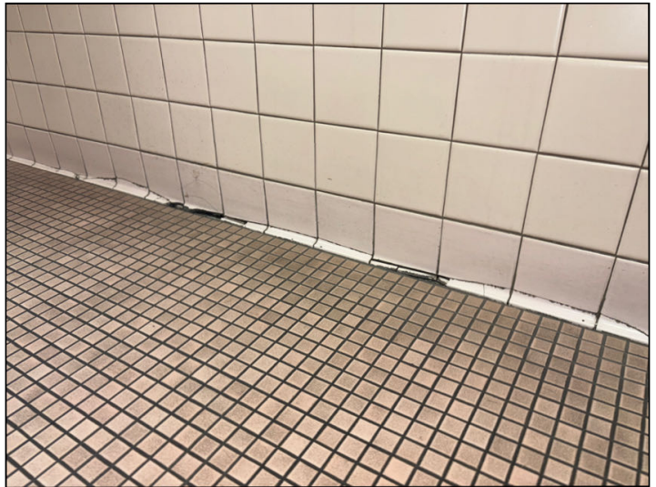
Cracked and damaged tiles were noted at many places where the walls meet the floors in the men's common restroom.
