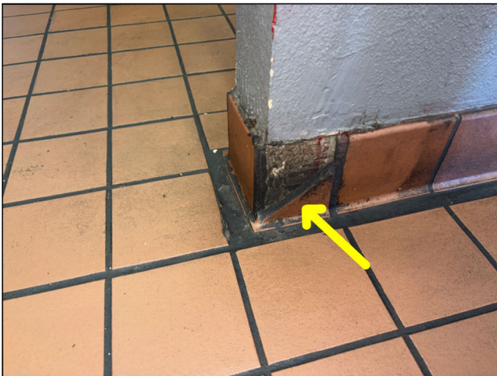
Damaged base tile was noted between the register and the kitchen at the front of 12308.
