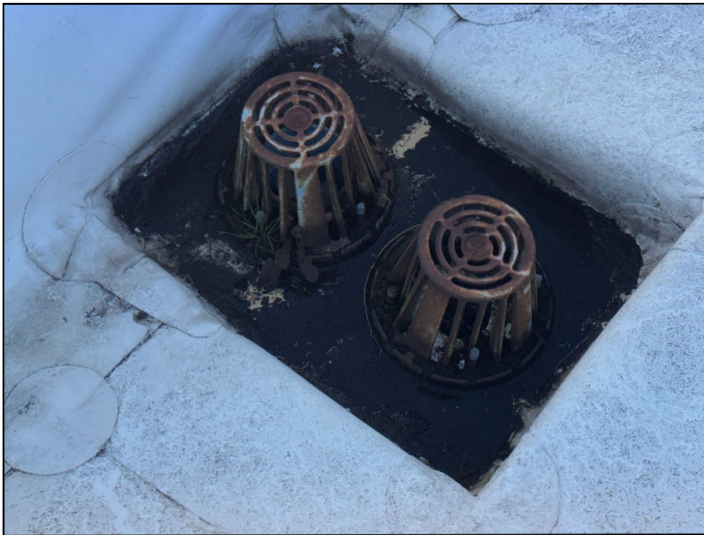
Recommend removing tree debris from the roof drains to help maintain proper drainage.
