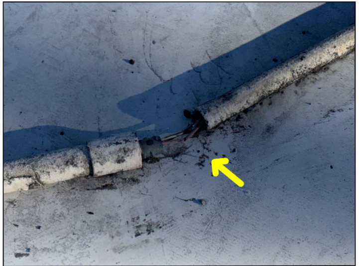
A detached conduit was noted on the roof of 12308.
