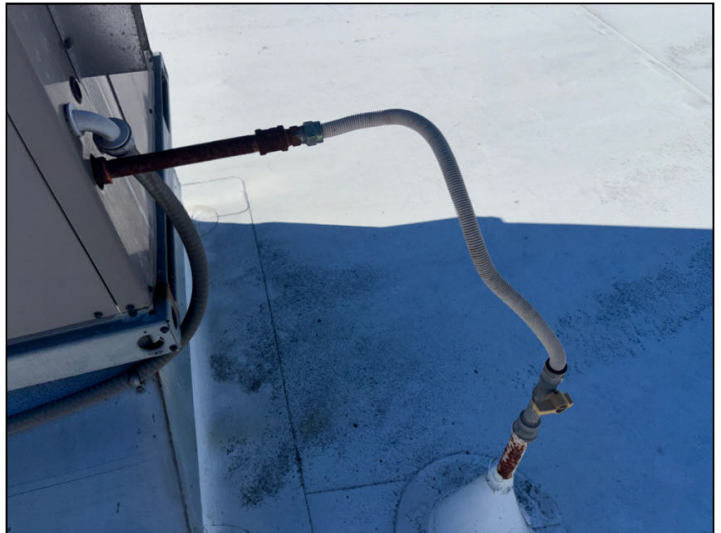
Rusted gas pipes and worn CSST gas connectors were noted in various places on the roof.
