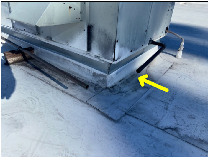
The condensate drain line for the package unit on the roof at 12324 is disconnected.
