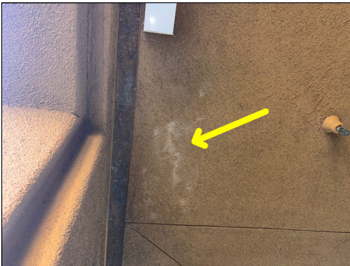
Efflorescence was noted at the underside of the eaves adjacent to the common restrooms.
