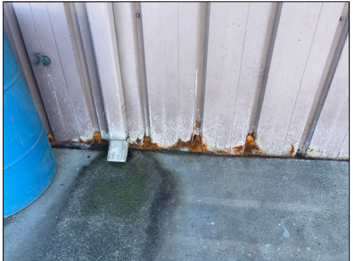
corrosion was noted in various places at the base of the rear exterior metal siding.
