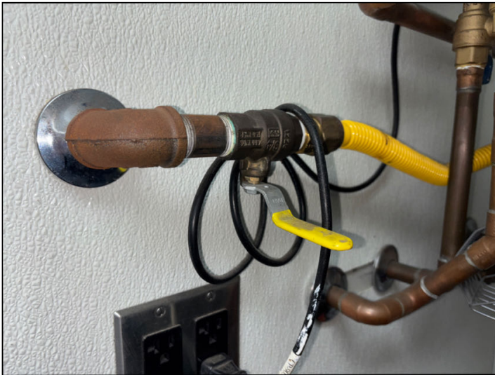
Gas supply was off to the water heater in 12300 at the time of inspection. This water heater was not operated.
