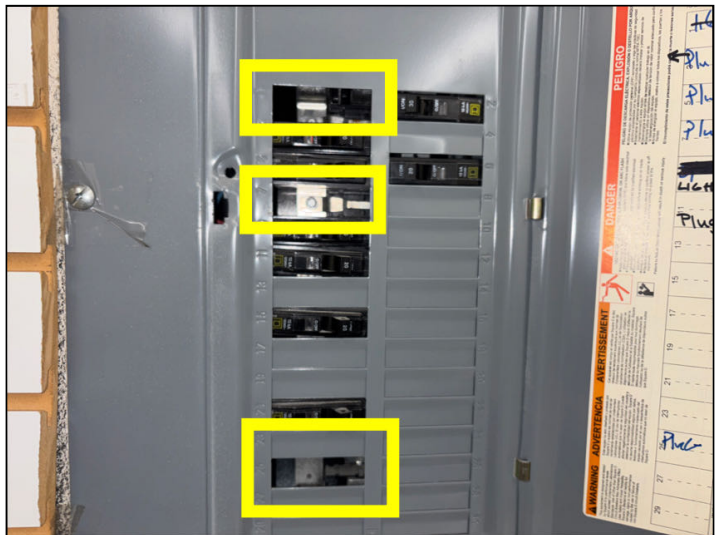
Missing filler plates were noted at the subpanel in 12320.
