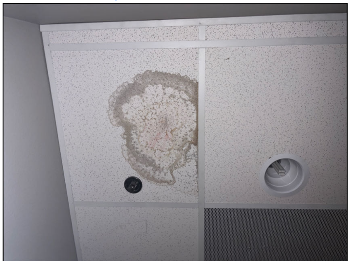
A stained ceiling tile and evidence of water intrusion were noted at the work station in unit 12326. The restroom ventilation duct penetrates the roof above this stain.
