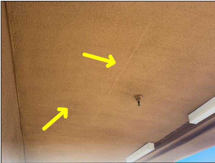
Patched cracks were noted in many places at the stucco trim and eave details.
