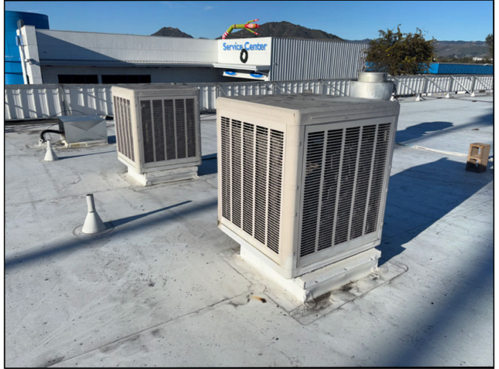
There are two evaporative coolers on the roof of 12308.
