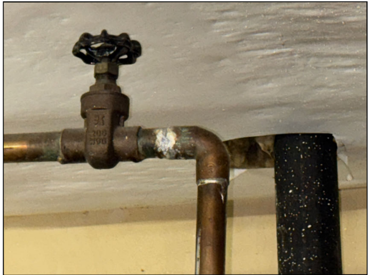
Mineral deposits and evidence of leakage were noted at a supply pipe over the restroom in 12310.
