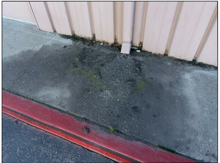
Deteriorated concrete was noted in various places adjacent to downspout terminations at the rear exterior of the building.
