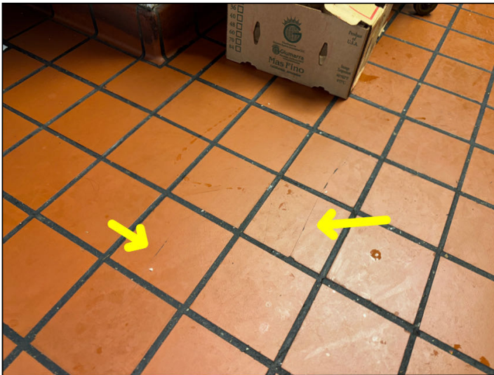
Various cracked floor tiles were noted in the kitchen of 12304.
