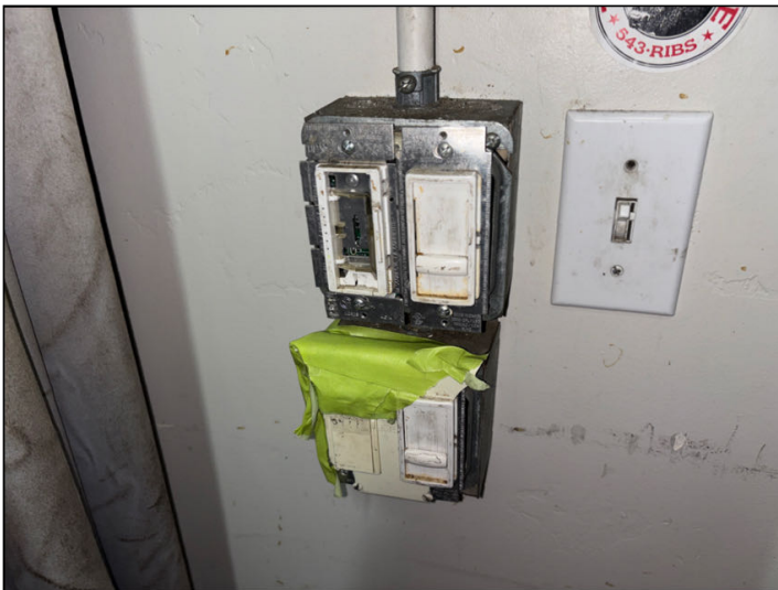
Damaged switches and switch cover plates were noted at the rear storage area of 12306.
