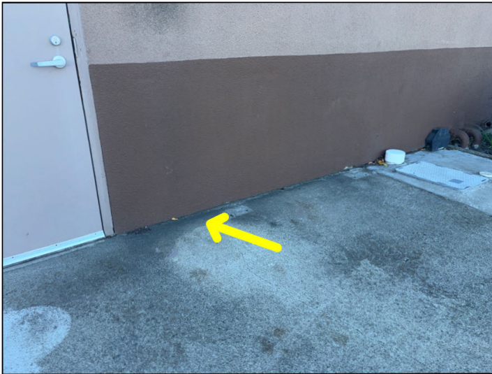
The stucco weep screed is blocked by paving at various places. This can cause moisture problems.
