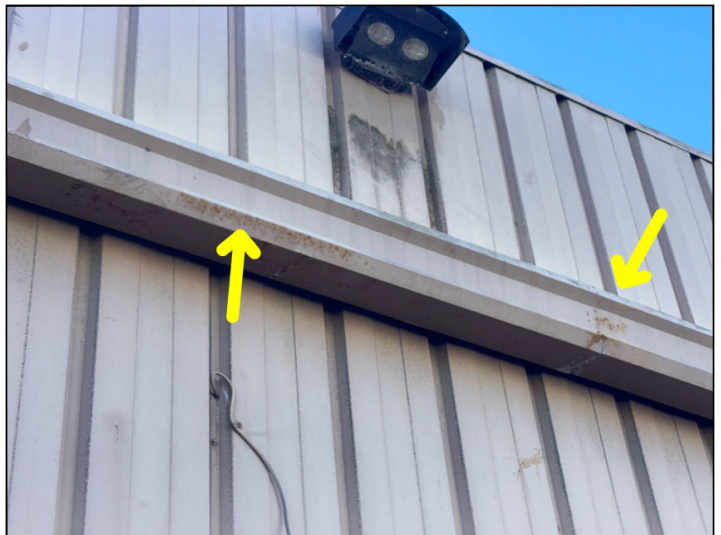
Corrosion was noted at the gutter in various places at the rear of 12320 and 12322.
