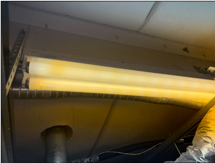
Recommend a proper light cage be installed around the light fixture in the attic over the 12326 restroom.
