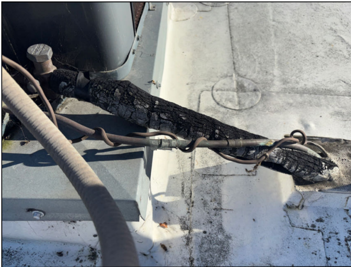
Deteriorated refrigerant line installation was noted adjacent to the split system condenser on the roof of 12300.
