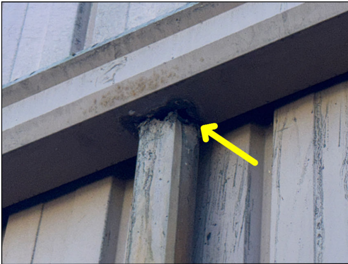
Corrosion was noted where a downspout is connected to the gutter at the rear of 12308.
