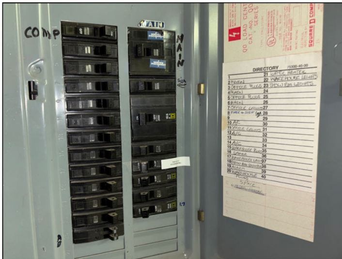
Incomplete breaker identification labeling was noted at the subpanel in the rear of 12310.
