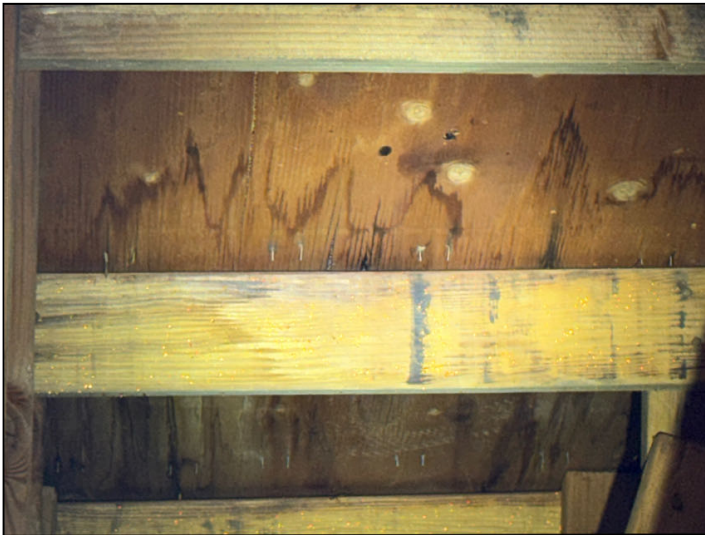
Moisture stains were noted in the attic of the stucco arch detail over 12338. The stains were dry at the time of the inspection.
