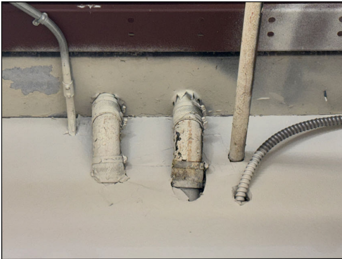
Corrosion and evidence of leakage were noted at the cast iron drain pipes where visible adjacent to the ceiling of 12340.
