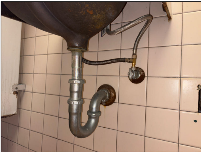
Corrosion was noted at various components below the men and women's restroom sinks.
