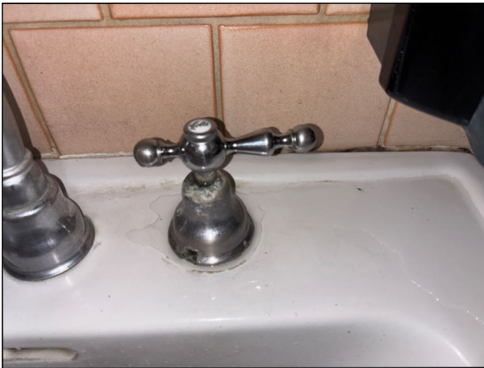
An active leak was noted at the cold water faucet in the restroom of 12306.
