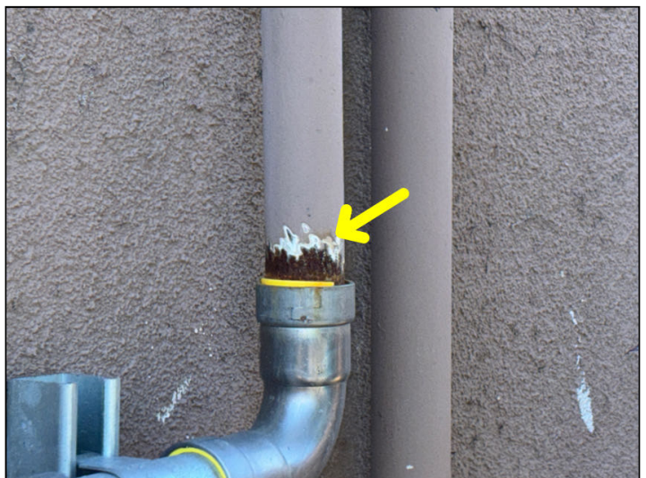
Corrosion was noted at a gas pipe adjacent to the gas meter area.
