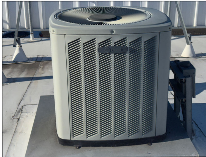
There is a split system condenser on the roof of 12326.
