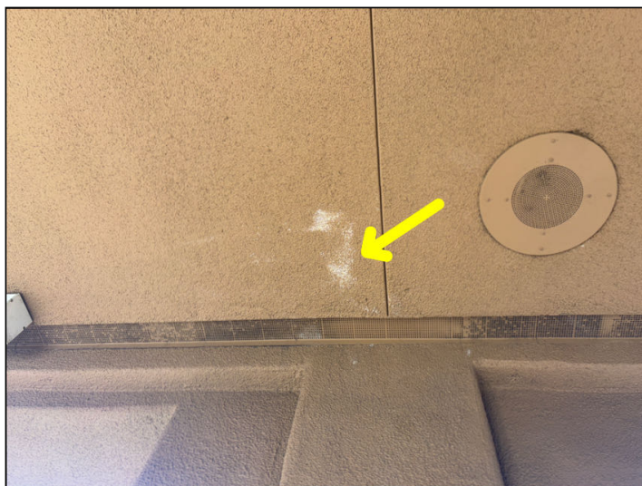
Efflorescence was noted at the underside of the eaves adjacent to 12308. This is an indication that water intrusion may have occurred from above.
