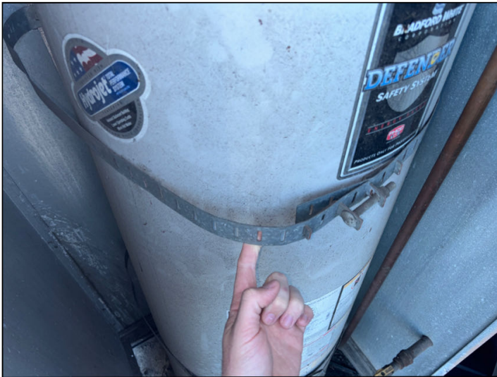
Loose seismic bracing was noted at the water heater at the rear exterior of 12304/06.
