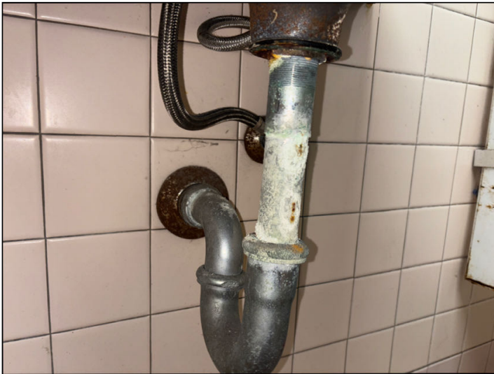
Heavy mineralization was noted at the drain lines below the men's common restroom sinks.
