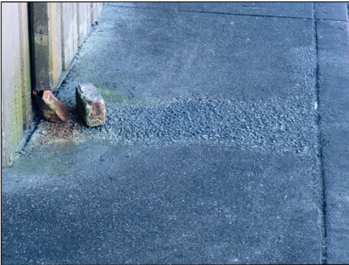
Deteriorated concrete was noted in various places adjacent to downspout terminations at the rear exterior of the building.
