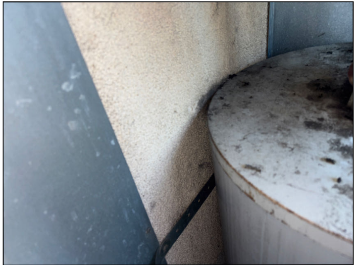
Recommend installing blocking between the water heater and the wall at the rear exterior of 12304/06.
