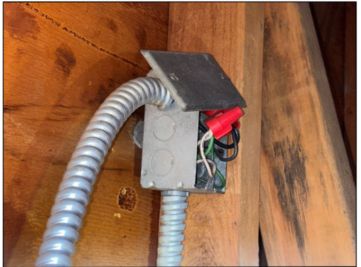
Open junction boxes were noted at various places in the stucco arch detail attic spaces.
