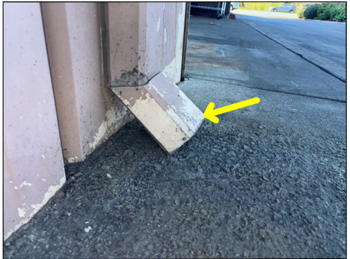
Recommend extending downspouts away from the building to help prevent water intrusion and foundation movement.
