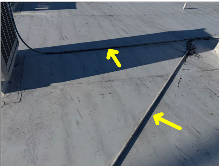
Unsecured conduits were noted in various places on the roof of 12308.
