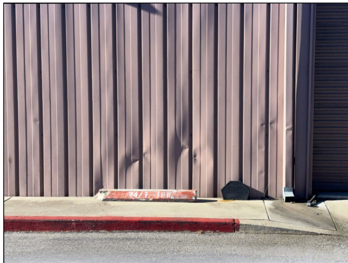
Damaged metal siding was noted at the rear of 12334.
