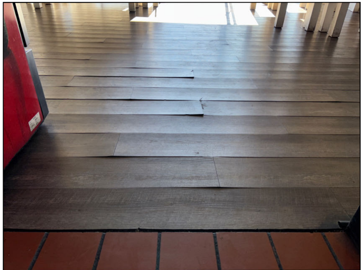
Damaged and uplifted vinyl planks were noted at many places in 12304.
