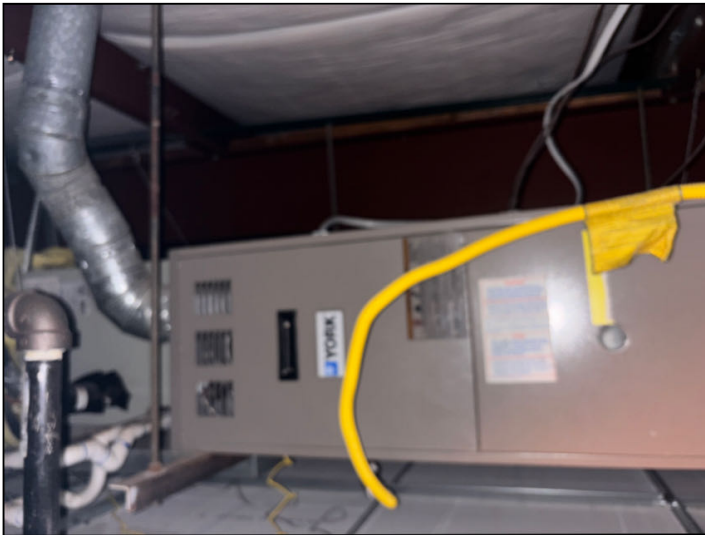
There is a split heating and cooling unit in 12300 above the ceiling adjacent to the entry door.
