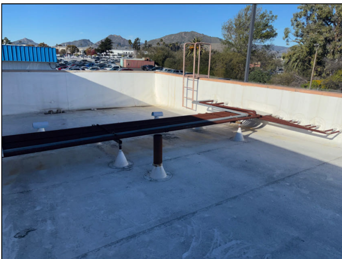
Corrosion was noted in many places at the gas lines on the roof.
