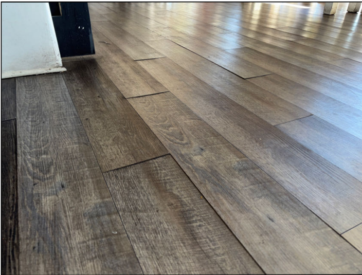
Damaged and uplifted vinyl planks were noted at many places in 12304.
