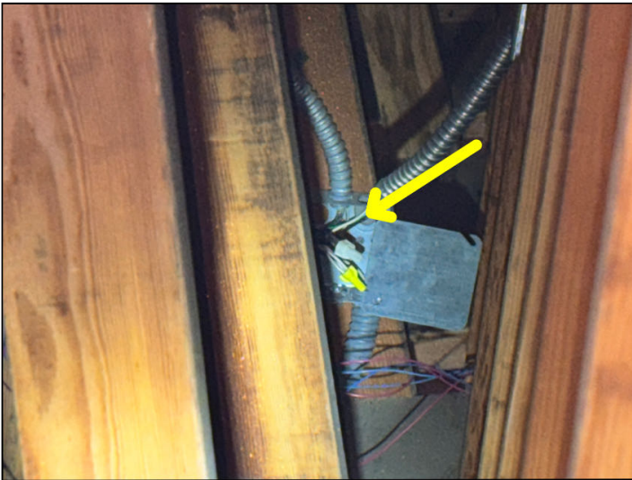
Open junction boxes were noted at various places in the stucco arch detail attic spaces.
