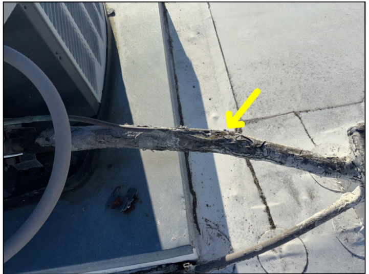
Deteriorated refrigerant line insulation and coatings were noted at the refrigerant line adjacent to the condenser over 12326.
