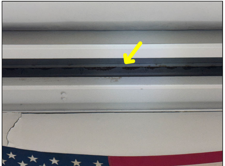
Corrosion and evidence of moisture intrusion were noted at the metal framing below the roof over the entry door of 12334.
