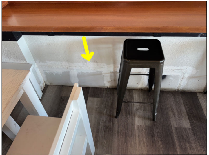
A large patch was noted at the base of the wall between 12306 and 12308.
