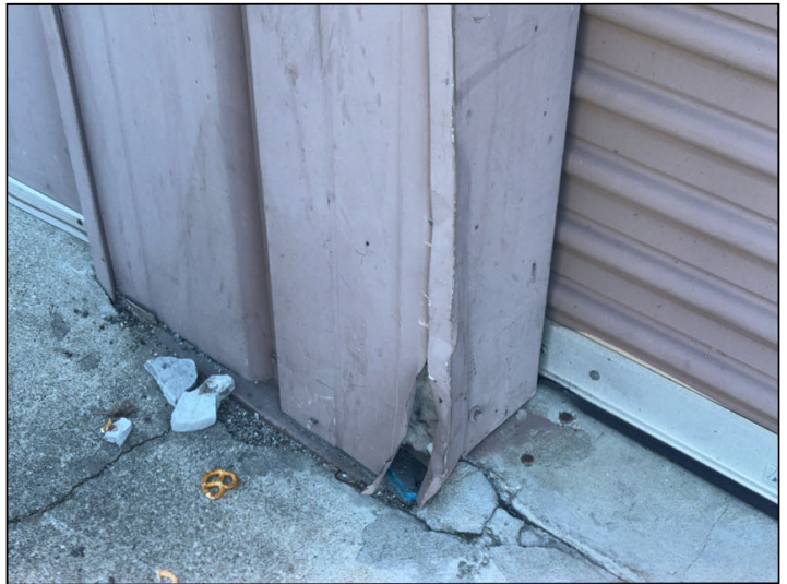
Vehicle damage was noted adjacent to the rollup door at the rear exterior of 12310
