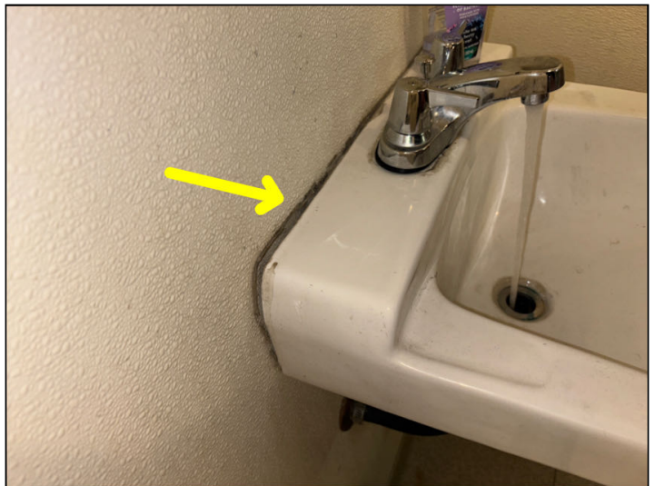
The sink is loose at the wall in the restroom at 12310.
