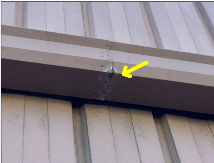
Stains and evidence of leakage were noted in many places at gutter seams.
