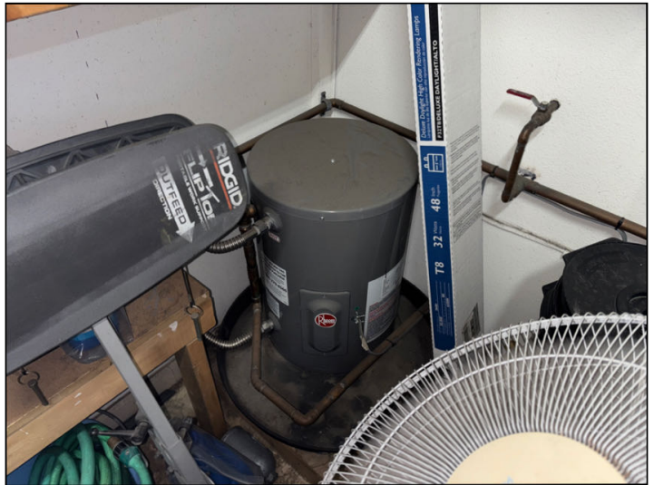
There is no seismic bracing at the water heater in 12322.
