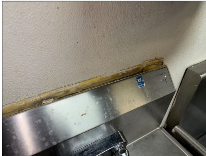
Cracked sealant was noted where a hand washing sink has separated from the wall in the kitchen of 12308.
