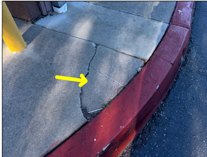
Damaged concrete was noted adjacent to the rear exterior of 12338.
