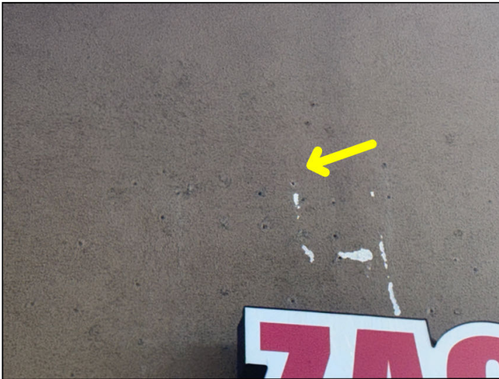
Cosmetic damage was noted in many places where fasteners have been removed adjacent to business signs.
