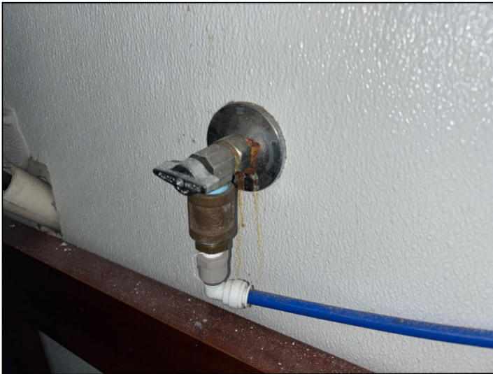
Stains and evidence of leakage were noted at a supply valve in the rear interior of 12300 adjacent to the water softener.
