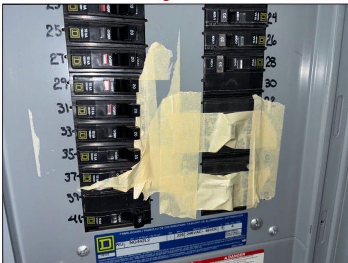
Various breakers are taped in the off position at the rear interior of 12300.
