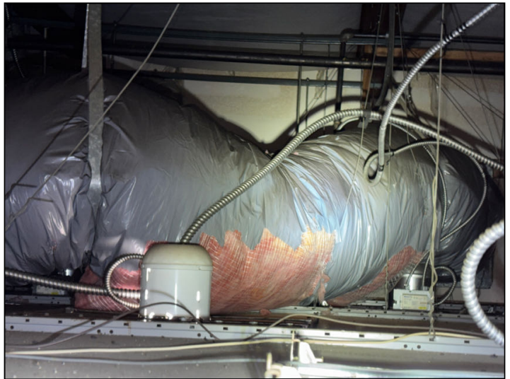
Older deteriorated gray ducting was noted in the attic over 12304.
