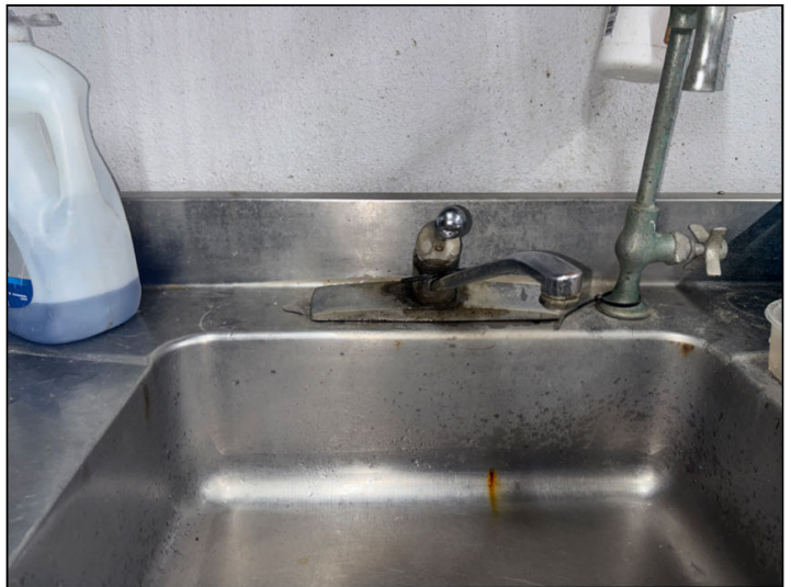
A loose sink faucet was noted at the rear sink in 12330. The sink has cold water supply only.
