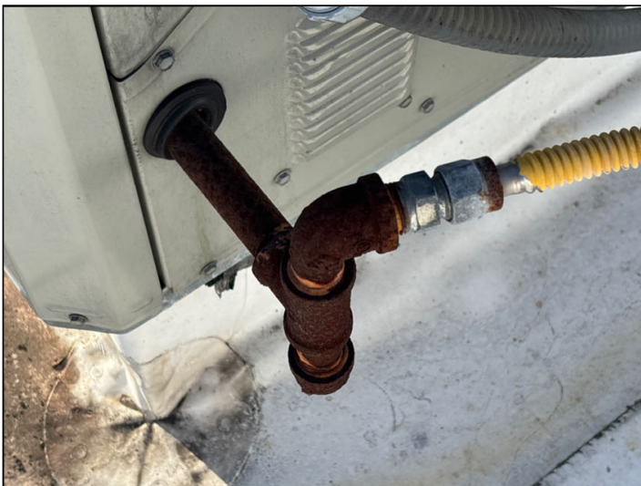
Rusted gas pipes were noted adjacent to various heating and cooling units on the roof.
