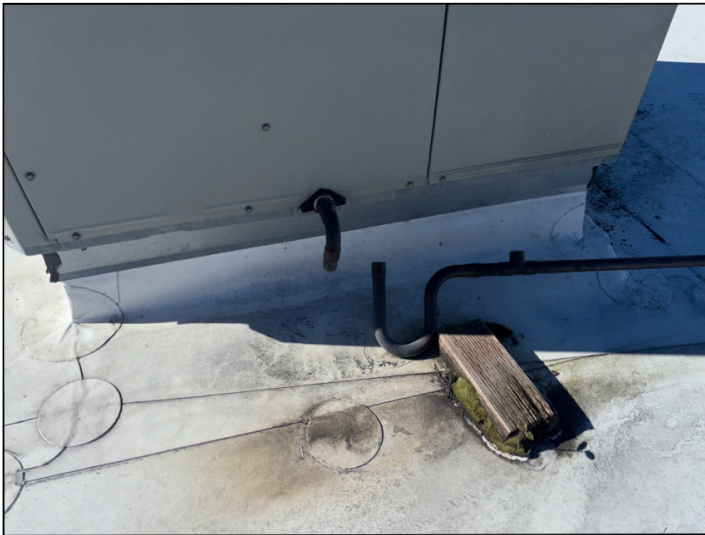
The condensate drain line for the package unit on the roof of 12310 is disconnected.
