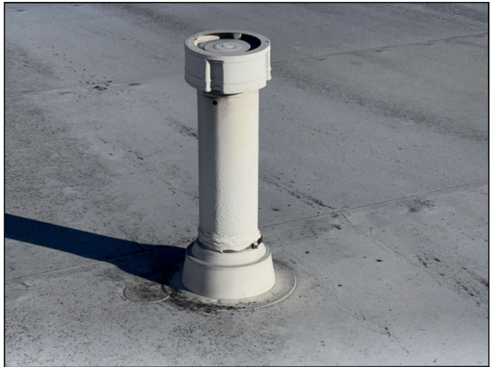
There are no double flashings at the vent pipes on the roof.
