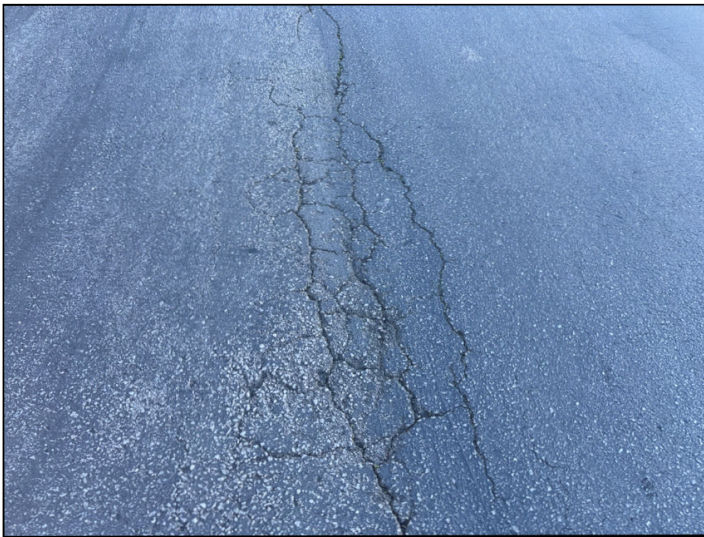
Cracked and fragmented asphalt was noted in many places at the driveway and parking areas.
