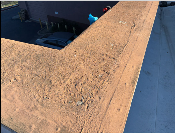
Peeling paint and deteriorated stucco was noted in many places at the horizontal surfaces of the parapet walls.
