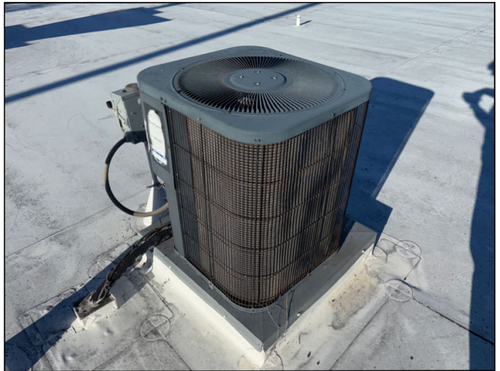
There is a split system condenser on the roof of 12300.
