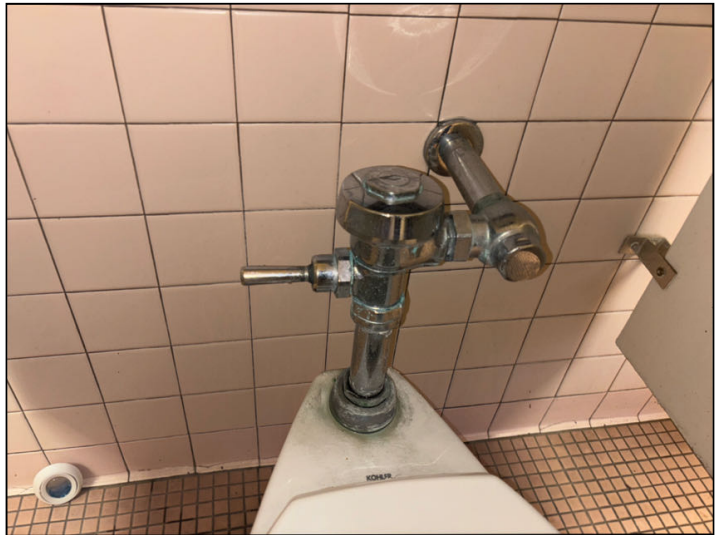
Mineral deposits and evidence of leakage were noted in many places at the common restroom toilets.
