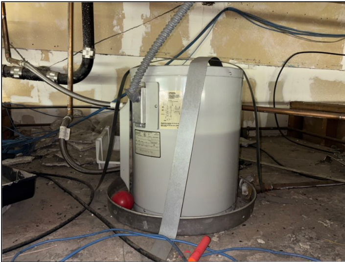
Inadequate seismic bracing was noted at the water heater in 12310.
