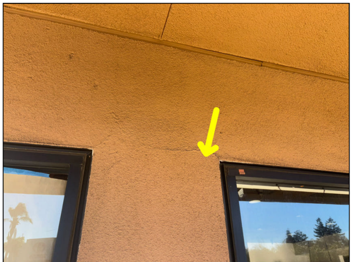
Cracks and patching were noted in many places at the exterior walls.
