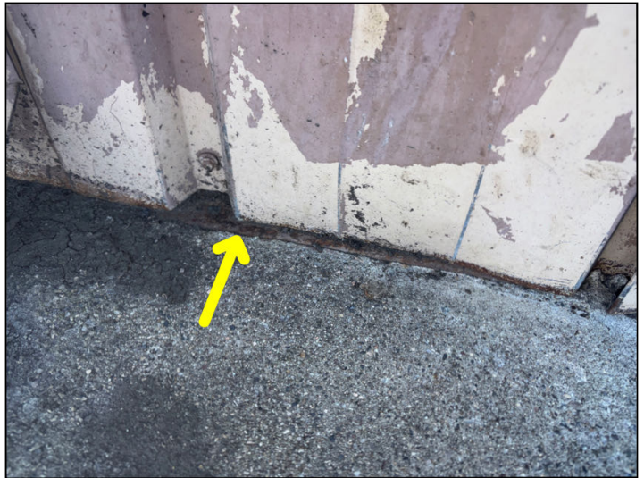
The bottom plate for the exterior metal siding is imbedded in paving and has corroded in many places.
