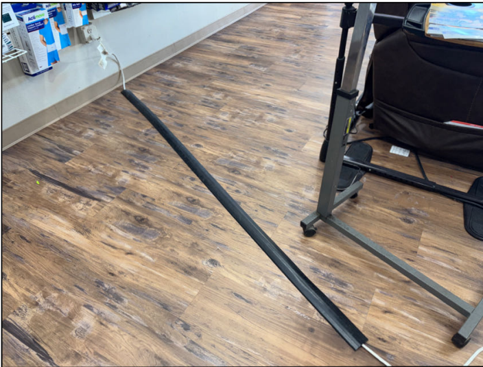
Temporary extension cords have been permanently installed at the sale room of 12310.
