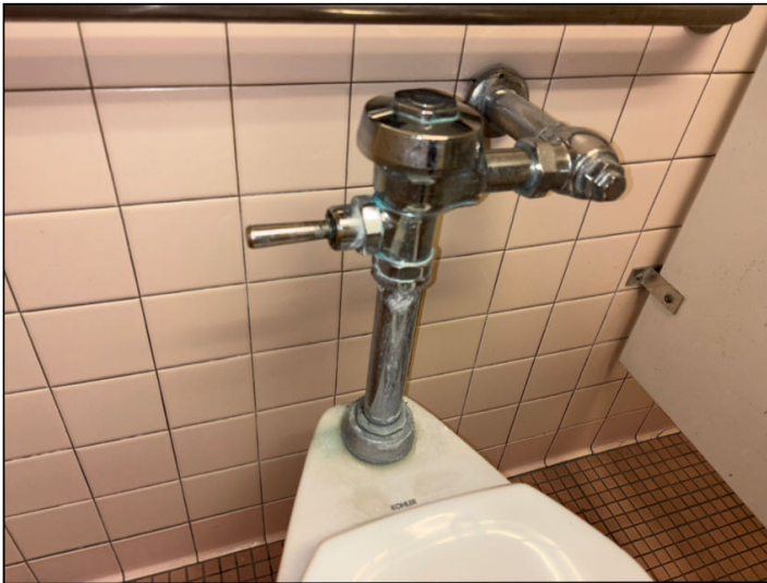
Mineral deposits and evidence of leakage were noted in many places at the common restroom toilets.
