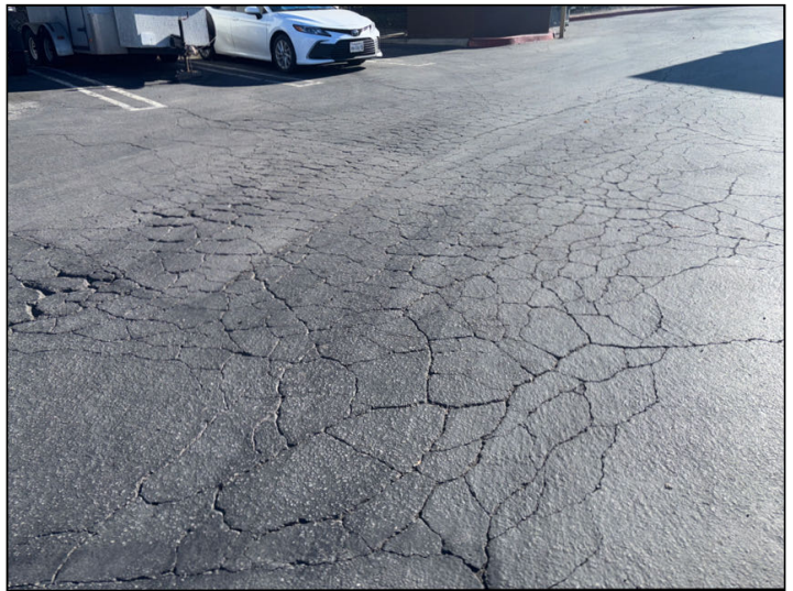
Cracked and fragmented asphalt was noted in many places at the driveway and parking areas.
