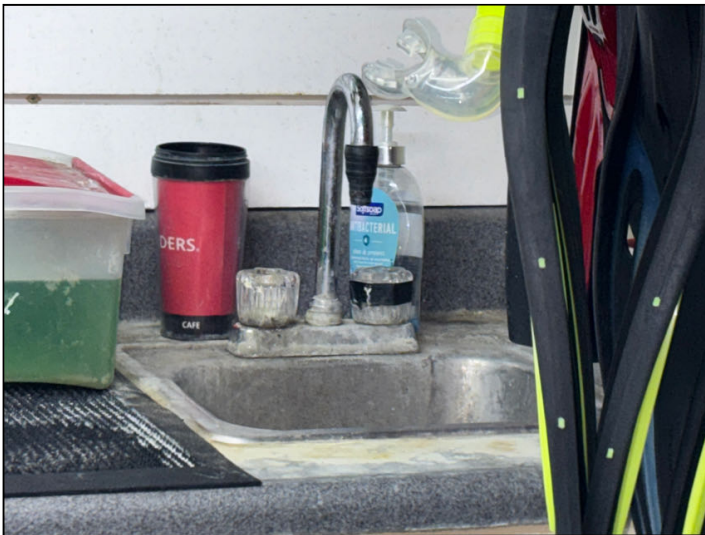
Mineral deposits were noted throughout the worker sink in 12322.
