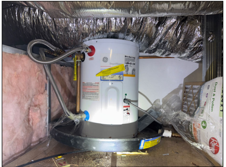
There is no seismic bracing at the water heater in 12326. Recommend installing blocking between the water heater and the wall.
