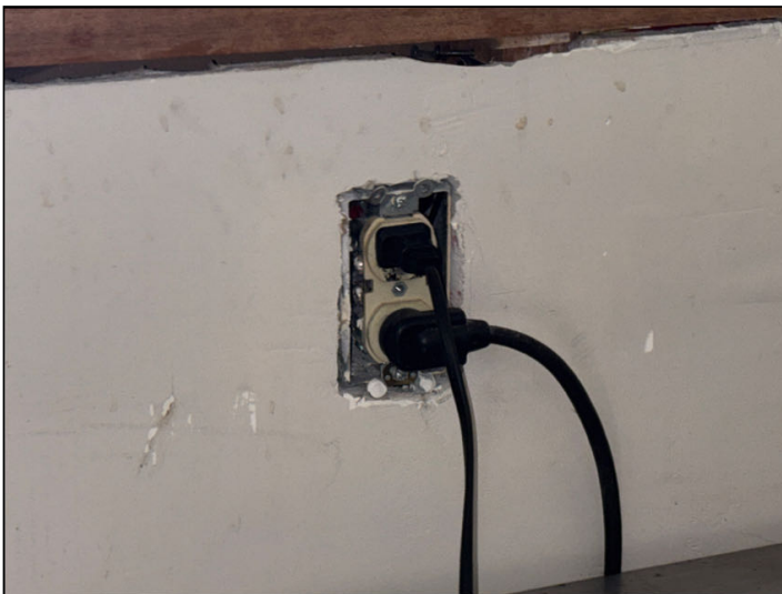
The missing receptacle cover was noted at the wet bar area of unit 12306.
