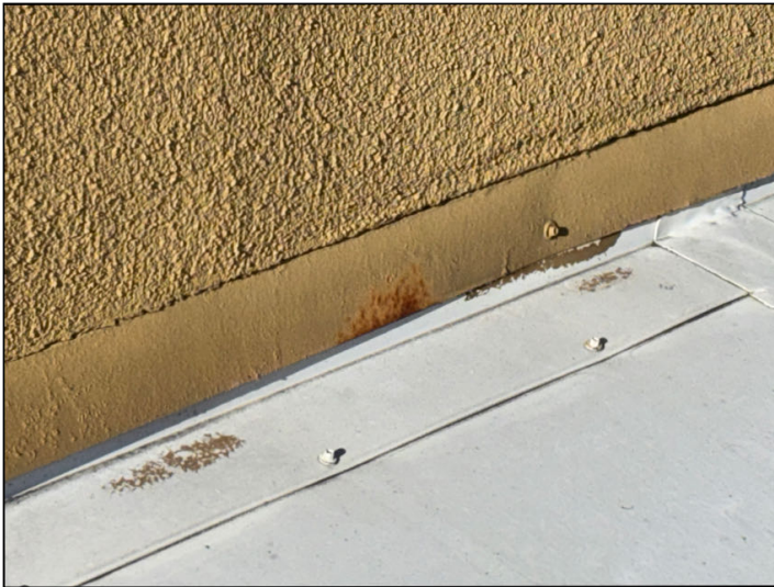
Corroded flashings were noted in various places on the roofs.
