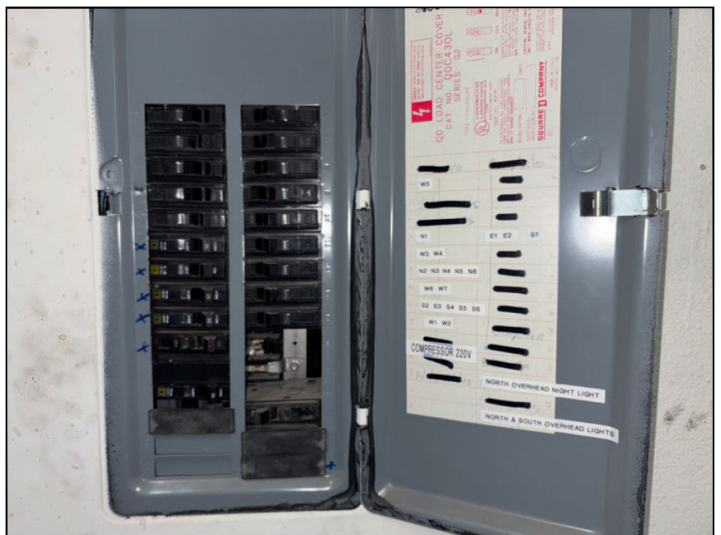
Incomplete breaker identification labeling was noted at the subpanel in 12322.
