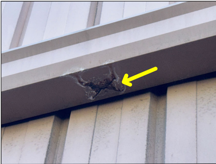
Corrosion was noted at the gutter in various places at the rear of 12320 and 12322.
