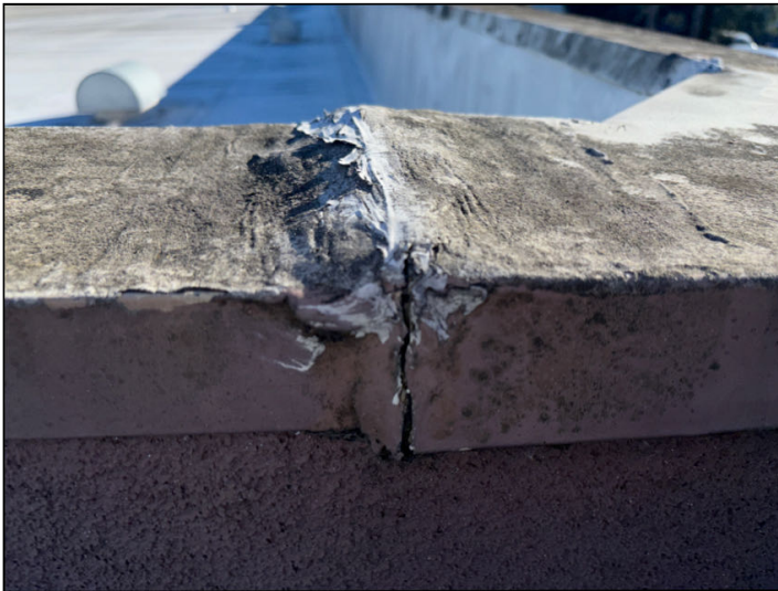
Cracked sealants and added sealants were noted in many places at the parapet cap flashings on the upper portion of the roof.
