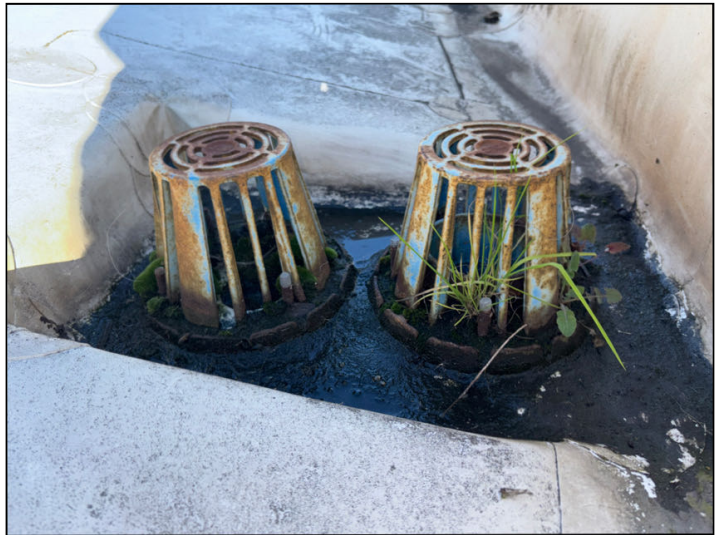
Recommend removing tree debris from the roof drains to help maintain proper drainage.
