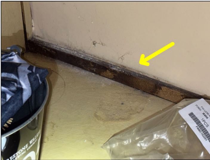
Moisture stains and evidence of past leakage were noted below the bar sink in 12306.
