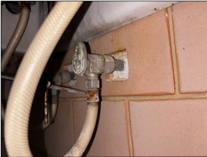
Corrosion was noted at the supply valves and adjacent connectors in the restroom of 12306.
