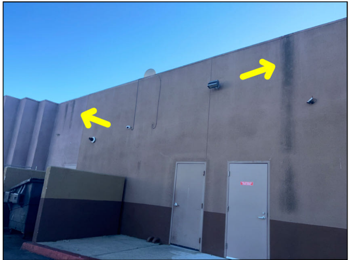
Stains were noted in various places at the rear exterior wall adjacent to 12300.
