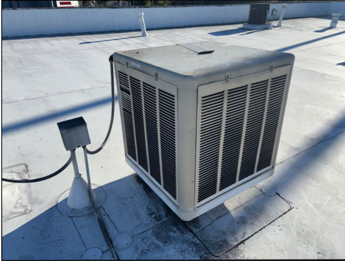
There is an evaporative cooler on the roof of 12304.
