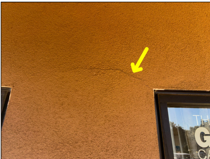
Cracks and patching were noted in many places at the exterior walls.
