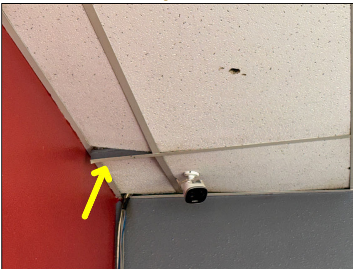
Damaged and displaced ceiling tiles were noted in various places at the front of 12308.
