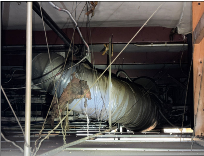
Older deteriorated gray ducting was noted in the attic over 12304.
