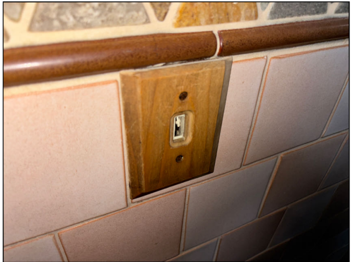
A damaged light switch was noted in the restroom of 12306.
