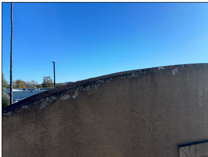
Damaged and flaking stucco color coat was noted in various places at the stucco arch detail over 12328.
