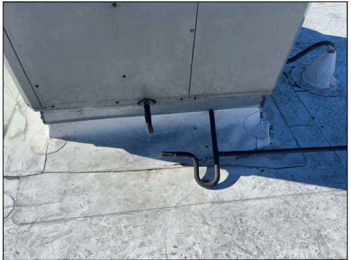
The condensate drain line for the package unit on the roof 12314 is disconnected in various places.
