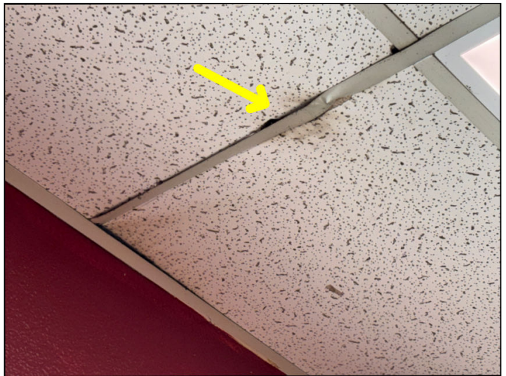
Damaged and displaced ceiling tiles were noted in various places at the front of 12308.
