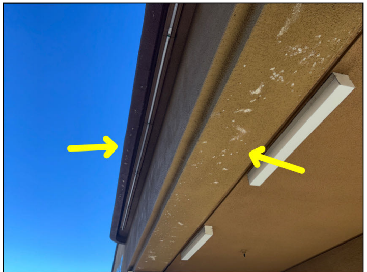
Efflorescence and evidence of leakage were noted at the underside of the stucco trim and eaves on the front of 12340. This area is directly below a flat stucco surface.
