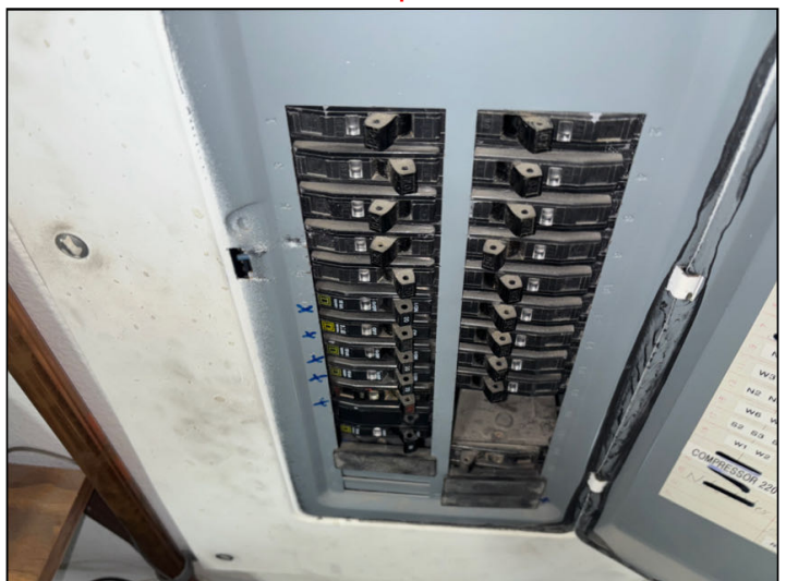
Various breakers were found in the off position at the time of inspection at the subpanel in 12322.
