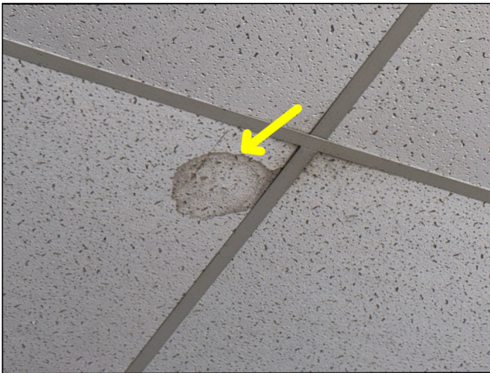
A moisture stain and evidence of water intrusion were noted at a ceiling tile at the front of 12308.
