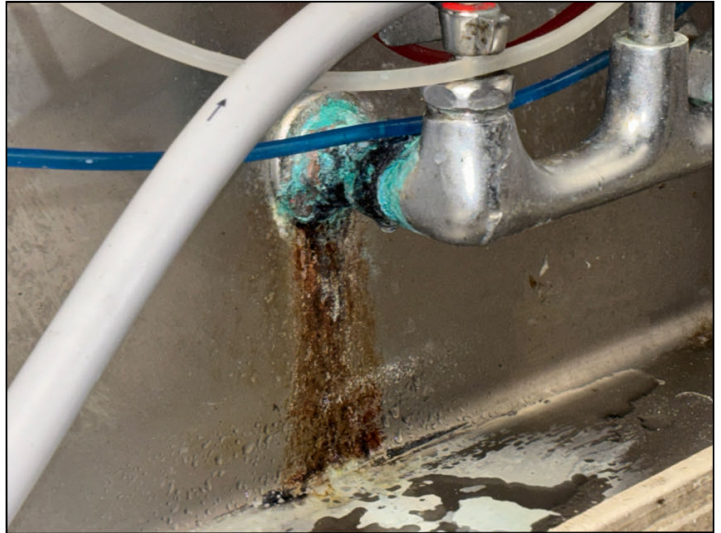
Active leakage was noted at a hot water supply pipe at a sink in 12304.
