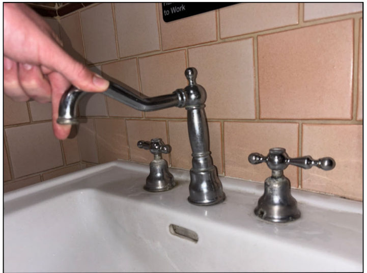
The sink faucet is loose in the restroom of 12306.
