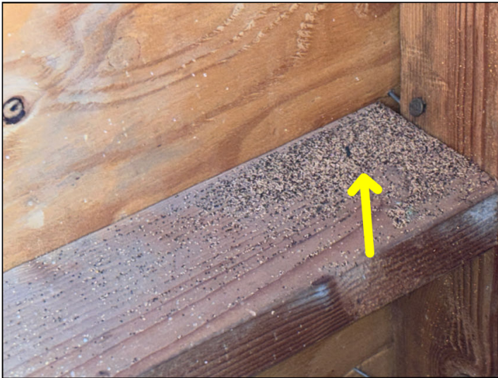
Apparent insect droppings were noted at various places in the attics of the stucco arch details on the roof.
