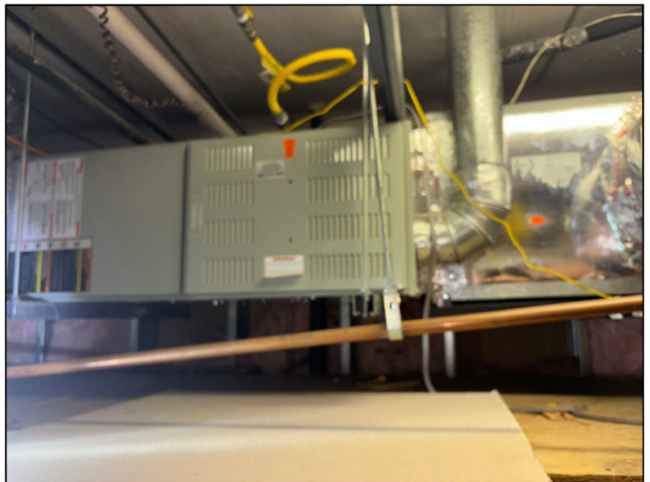
There is a split heating and cooling system in the attic over the 12326 restroom.
