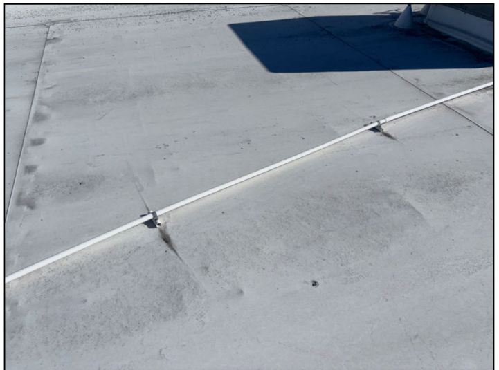
The condensate drain lines for the package units on the roof are not secured to the roof.
