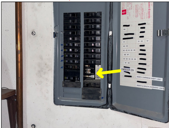
Missing filler plates were noted at the subpanel in the rear storage area of 12322.
