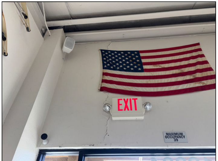
Cracked and peeling paint and evidence of water intrusion were noted at the wall over the entry door to 12334. Hidden damage may be present.
