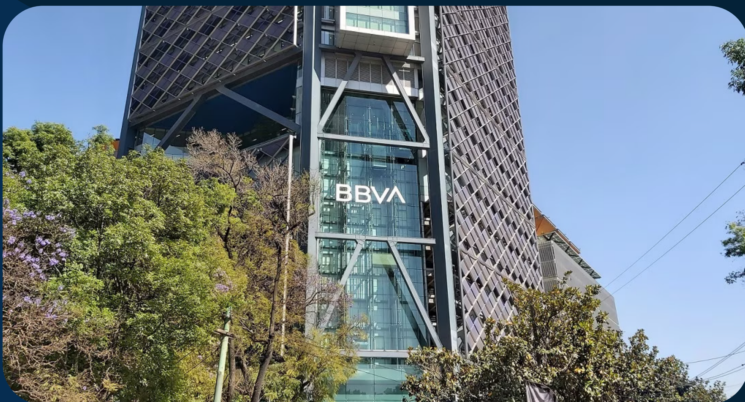
BBVA TOWER CD. DE MÉXICO, QC INSPECTION
