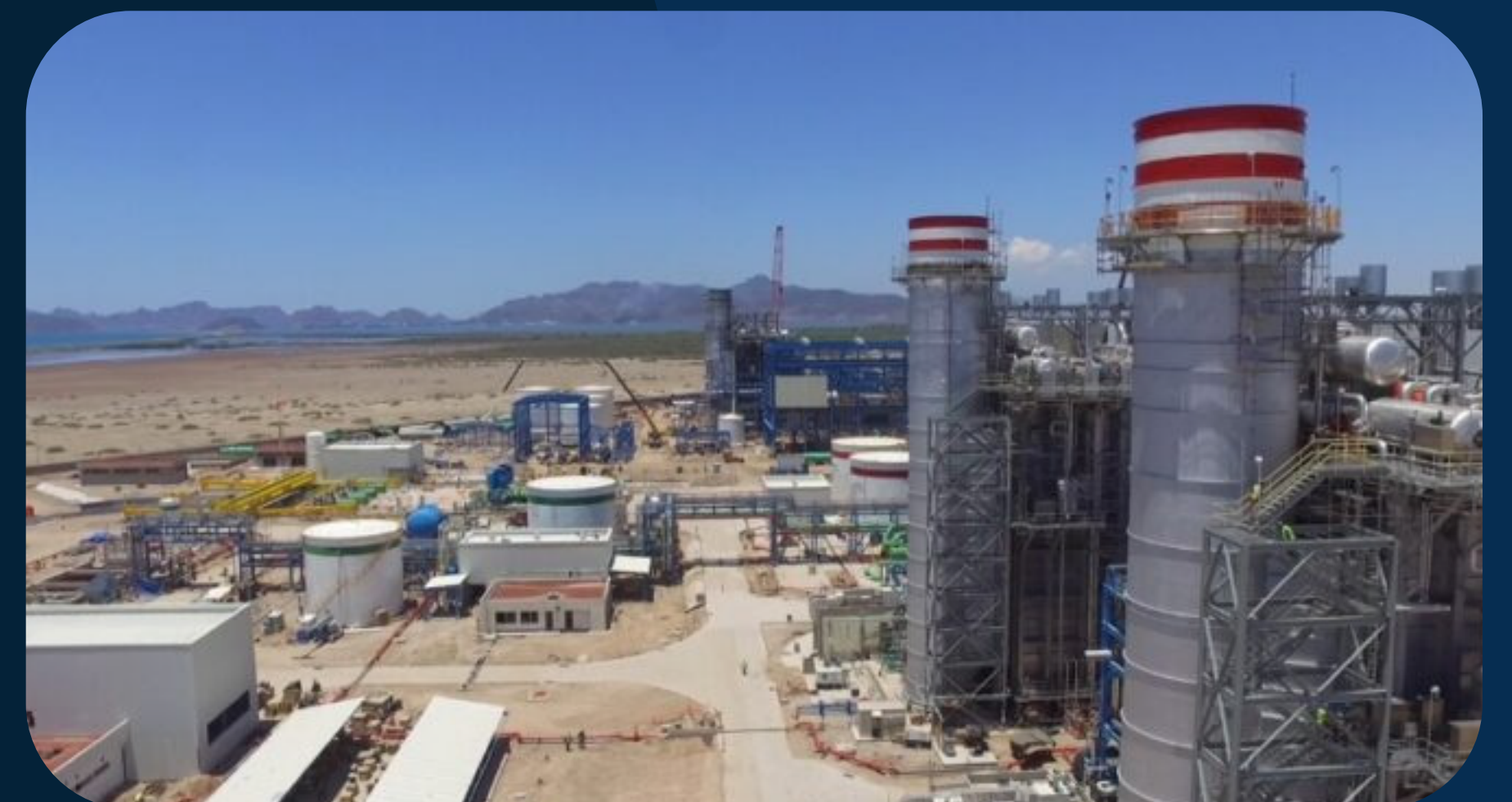
CFE COMBINED CYCLE POWER PLANTS MEXICALI Y SAN LUIS RÍO COLORADO
