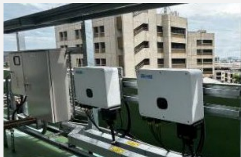
PV 103.24kWp Billion Giga-40-60K PV Inverter
