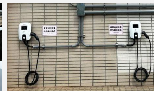
AC EV Charger 14kW Billion BH-2000 7kW AC EV Charger
