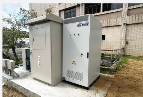
ESS 100kW/215kWh Billion Fusio One-100kW/215kWh Energy Storage System
