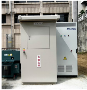
Kaohsiung PV 103.24kWp+ESS 100kW/215kWh+AC Charger 14kW+DC Charger 120kW
