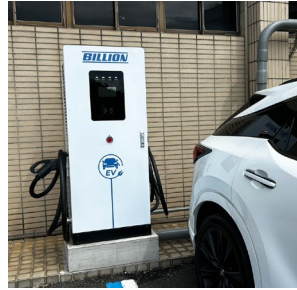
Kaohsiung PV 103.24kWp+ESS 100kW/215kWh+AC Charger 14kW+DC Charger 120kW
