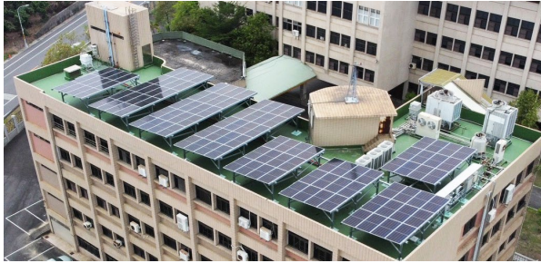
Kaohsiung PV 103.24kWp+ESS 100kW/215kWh+AC Charger 14kW+DC Charger 120kW
