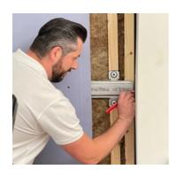
**8.** Before installing the first plasterboard layer, mark the locations of the furring channels on the surrounding walls in chalk or pencil. This will help you to locate the position of the furring channels later once the first layer of plasterboard is on and furring channels are no longer visible.
