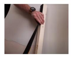
2. Build the stud frame attaching the isolation strip around the perimeter of the stud frame. This sits between the stud frame and the surrounding surfaces and has a self adhesive backing.
