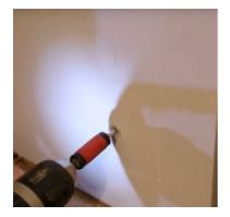
**10.** While holding the acoustic plasterboard in position use the 25mm self-drilling screws to secure the board into each ReductoClip furring channel. Screw the fixing in place until the screw head is flush with the plasterboard. A screw should be used every 200mm on each furring channel. Once the first plasterboard is in position, apply the next board butting up tightly to the previous board and continue.
