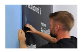
12. Install FlexiSound 5. FlexiSound is self-adhesive and requires no fixings or secondary adhesive. Stick the FlexiSound to the plasterboard covering the entire wall leaving no gaps. The FlexiSound can touch the walls and ceiling, as it is a soft material and won't aid in the transfer of sound energy. It also helps to seal the first layer of plasterboard.
