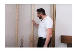
**4.** The stud frame should be built at 600mm centre widths. Use noggins if necessary for larger walls to give extra support.
