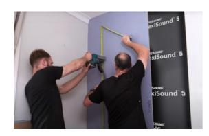
**12.** Install the second layer of 15mm acoustic plasterboard using 50mm self-drilling screws. Stagger the joins by starting at the opposite side from where you started on the first layer. This should sandwich the FlexiSound between the two layers. A screw should be used every 200mm on each furring channel. A 5mm gap should be left around the perimeter again too.
