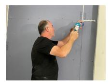
**14.** Finally remove the shims and fill the gaps around the perimeter with Acoustic Sealant.
