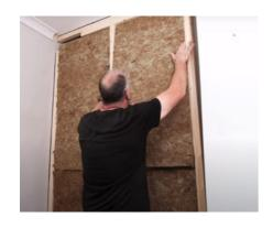
**6.** Install Acoustic Mineral Wool between studs. If the studs are installed at 600mm centres, mineral wool slabs should be slightly compressed either side and friction fit into the space between battens. No fixing required.
