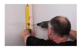
**4.** Secure the new stud frame in place with suitable fixings, screwing through the stud frame and isolation strip into the returning walls, ceiling and floor. A minimum of 10mm air gap should be left between the new stud frame and the existing stud wall. There should be no parts of the stud frames touching each other.
