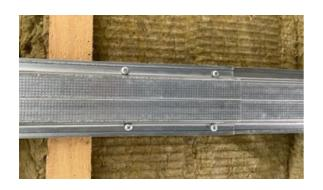
8. Snap the ReductoClip furring channel into the ReductoClip by squeezing the furring. IMPORTANT: Make sure to overlap channels by 150mm and secure with 4 self tapping screws (not supplied). Make sure overlaps occur between the clips, not on the clips. Ensure furring channels are overlapped alternatively, front to back and so on.
