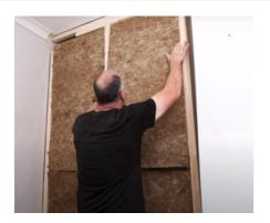
**2.** Install Acoustic Mineral Wool between studs of the existing stud frame. You should use the same thickness mineral wool as the depth of the studs.
