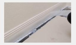
**2.** Add Perimeter Flanking Strip around the perimeter to isolate all floor layers from the walls.
