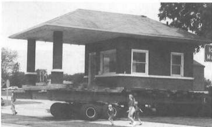
STATION BEING MOVED TO IT'S NEW HOME
