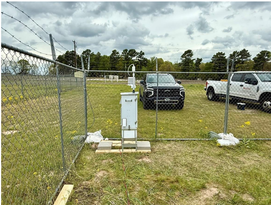
Figure 2.2. Northwest Photo of Monitoring Station
