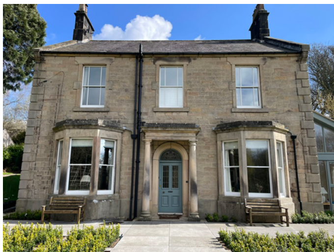
Sliding sash window replacements
