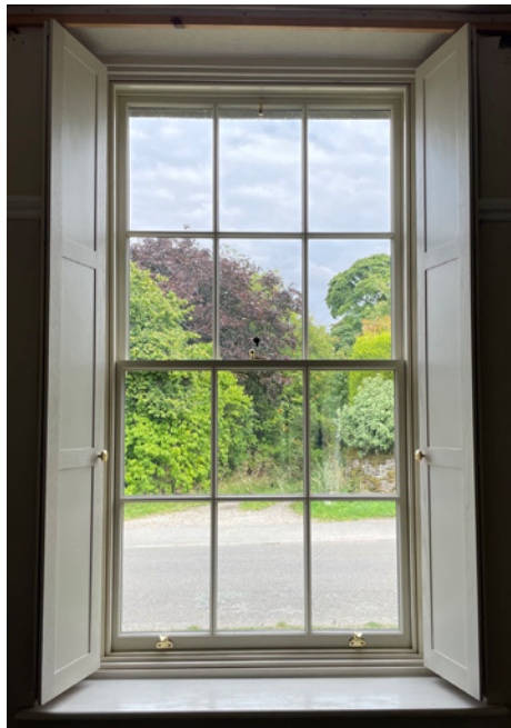
Sash window with heritage double glazing
