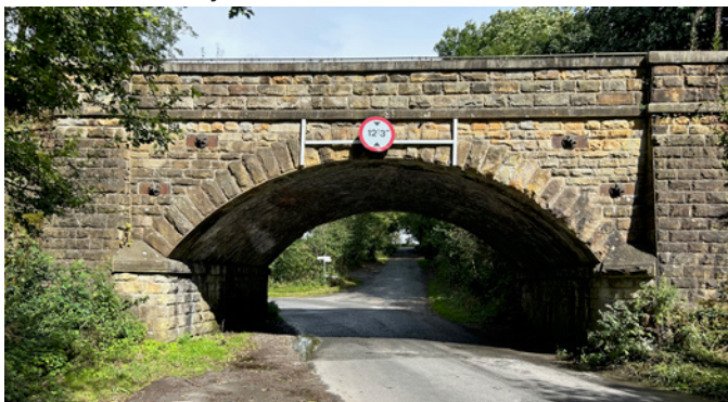
Longstone Hole Bridge
