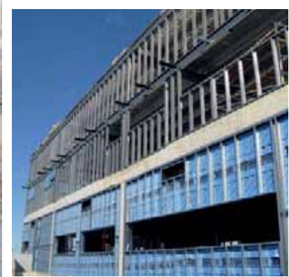
External Infill Framing Between concrete and steel structures
