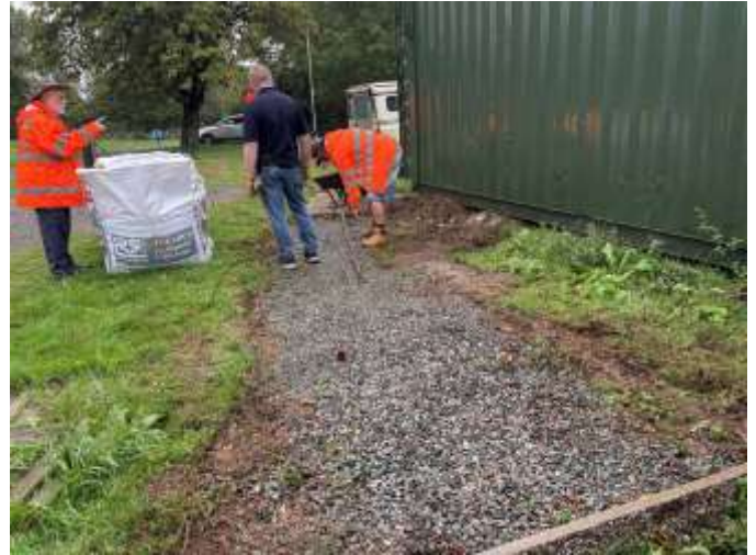
Level pegs checked and the slope re-graded
