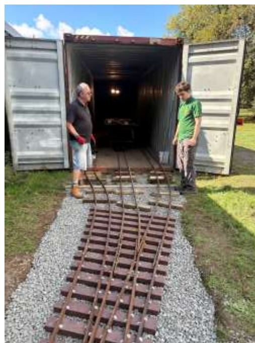
Rolf and Kai working on the bridging rails to the container
