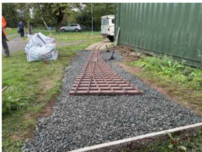
Point maneuverer into alignment
