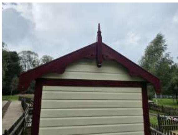
Finials as replicated from the Quorn and Woodhouse signal box.
