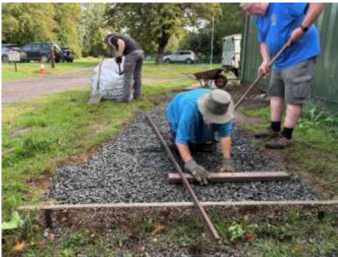
Levelling the bed - Tony making a start using our tried and tested method
