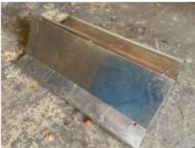
The new well roof top
