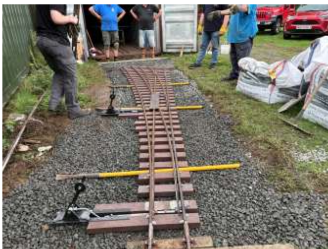
Point lifted out - weight shared between eight of us!
