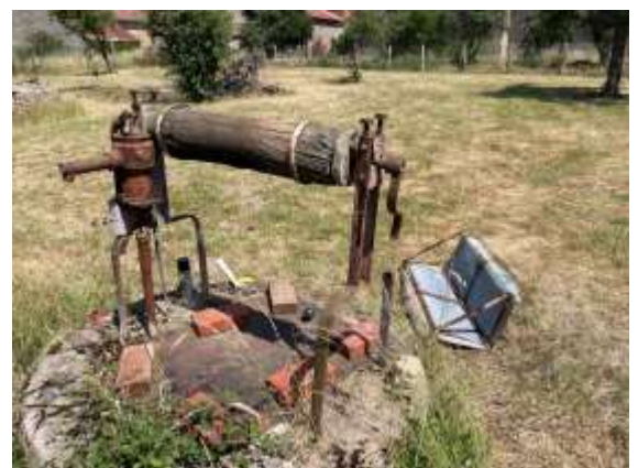
The well during dismantling during June this year
