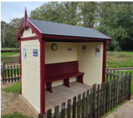
Showing the completed shelter with the 3 half circles on each fascia board and the finials.
