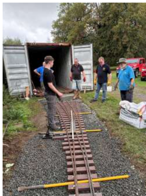
Checking the level and removing the lifting bars
