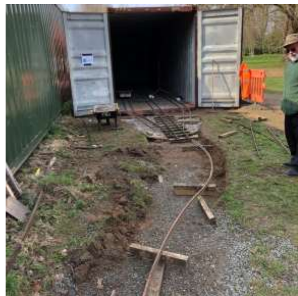
Our first attempt at the connecting rail - I think we were over enthusiastic with the rail bender!
