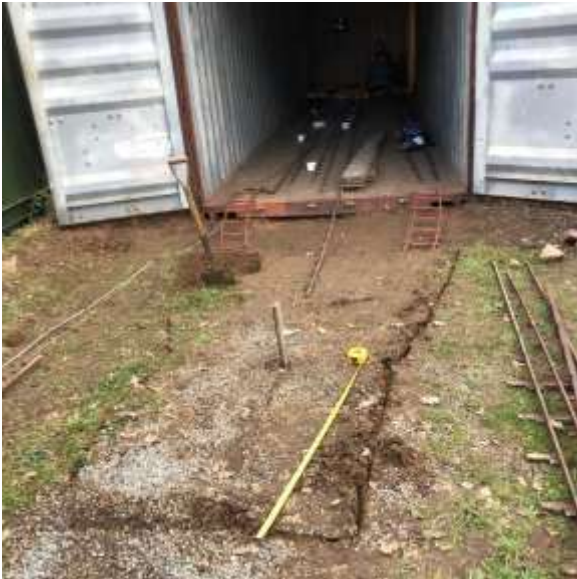
Initial excavations and rails laid to feed the new carriage container.
