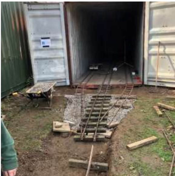
The permanent rails in position (but not fixed).
