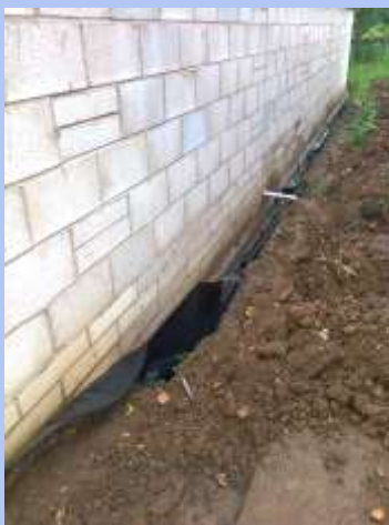
Work continues to dampproof CS3.
