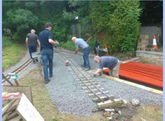
Work completed, note the traverser now has a coat of oxide paint!
