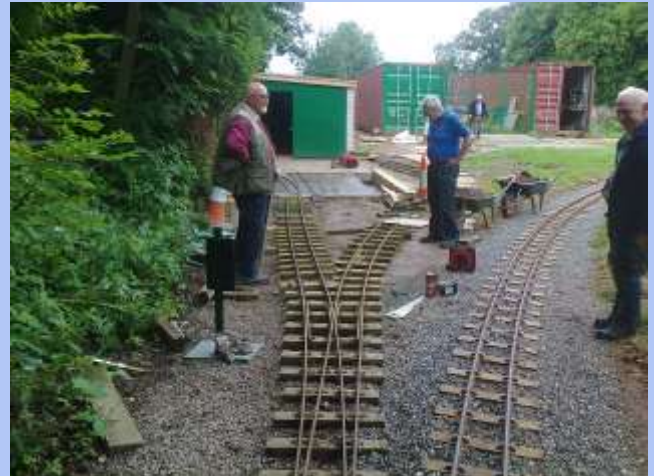
The track gang get busy sorting out the point to feed the traverser and workshop.
