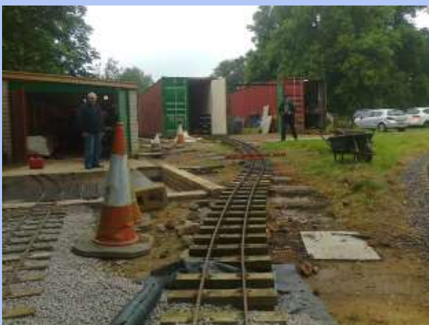
Work progressing on the point ant two lines.
