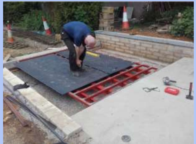
Aubyn busy attaching chequer plate to the traverser
