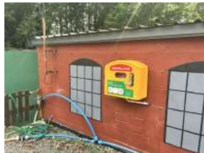
The cabinet on the side of Carriage shed 2.
