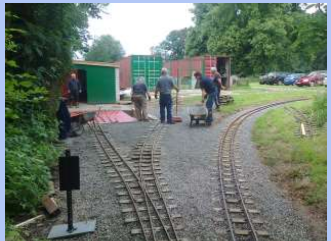
Work progressing continued...
