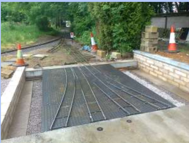
Chequer plate fixed and rails in place
