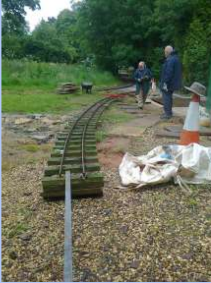
Work progressing continued...
