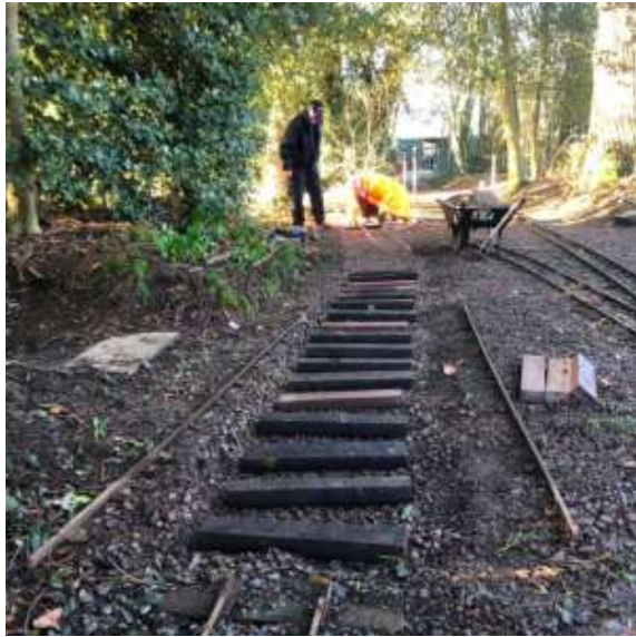
Sleepers in place to protect the levelled bed.
