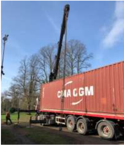
Setting up ready for the lift.
