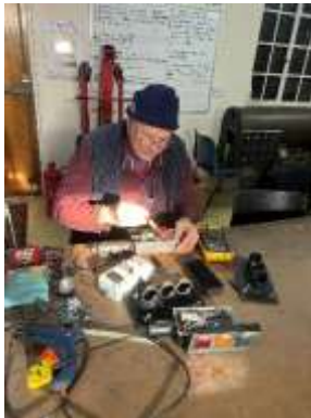
Peter checking and repairing the signals.
