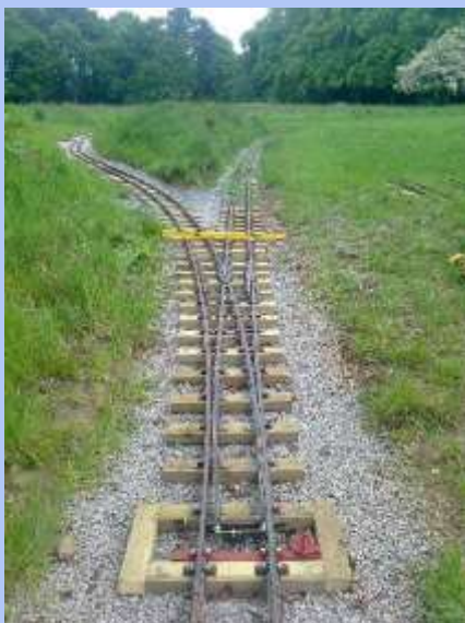
Point installed - but at this stage they were not powered.
