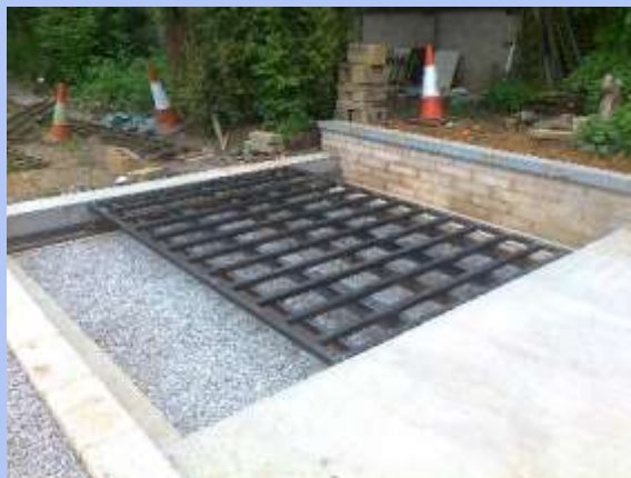
The main structure of the moving base completed.
