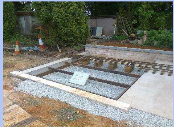
Bottom tracks in for the traverser to run on.
