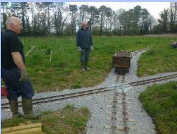
Ballast was being used on the diamond crossing on the 'short route'.
