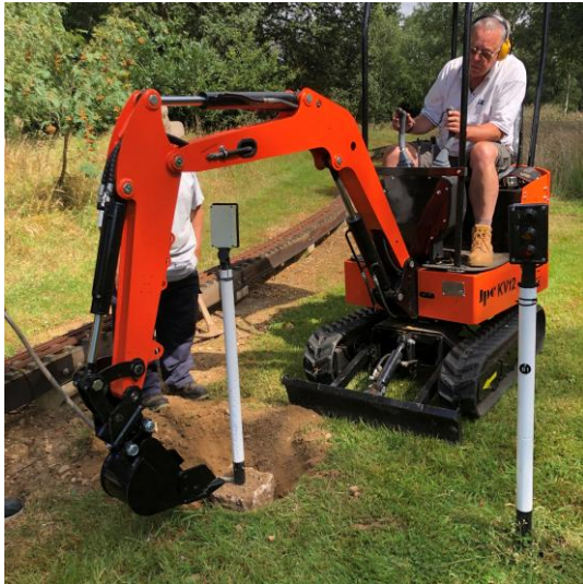
A RT signal needed to be moved, so the track gang took on the task, dug all around but needed Mini-Digger to give it a nudge.
