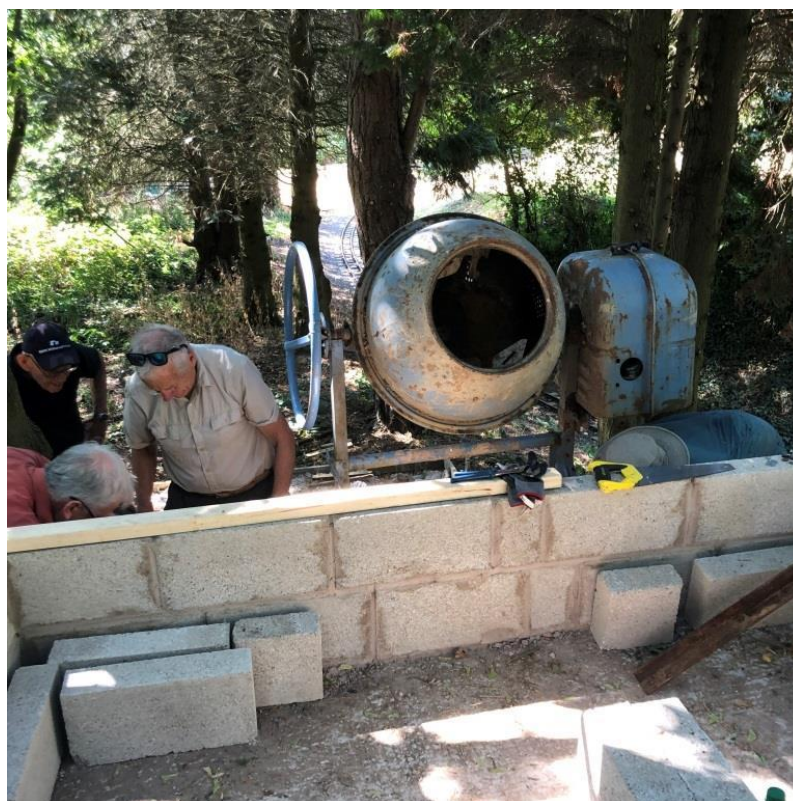
Ballast washer now in place
