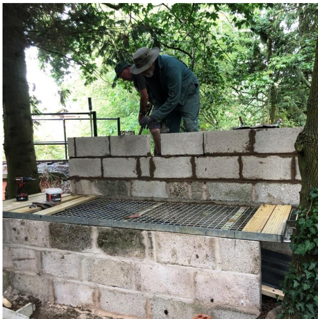
The ballast washing plant is progressing with Geoff Broad and his gang - Geoff laying blocks.
