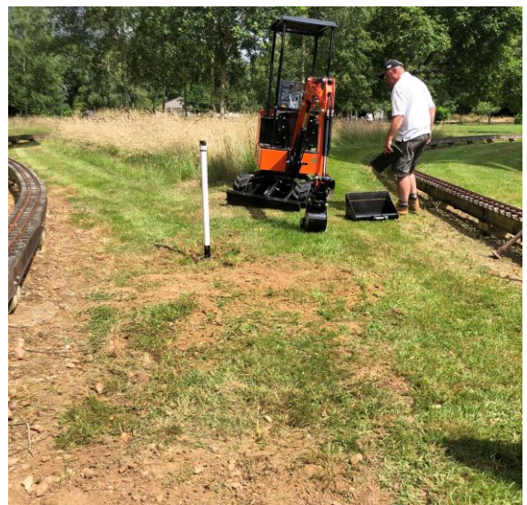
Job done and signal in its new position, the new mower can now get by!
