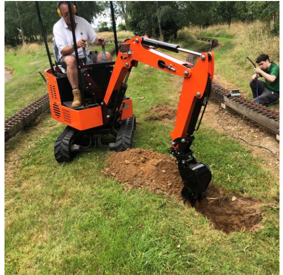
Rolf digging the hole with his Mini-Digger to 're-plant the signal'
