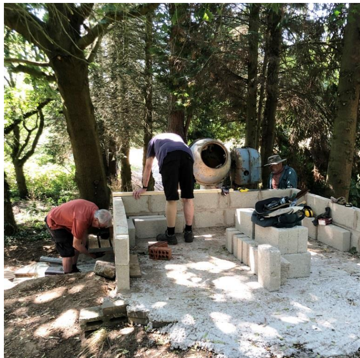
Job getting nearer completion!
