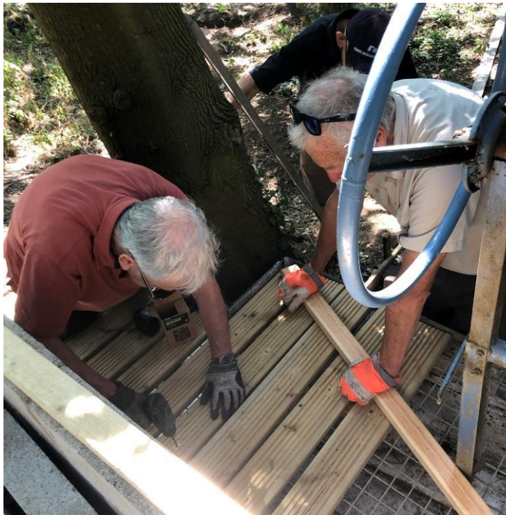
Peter Featherstone and John Powell fixing decking boards for standing on
