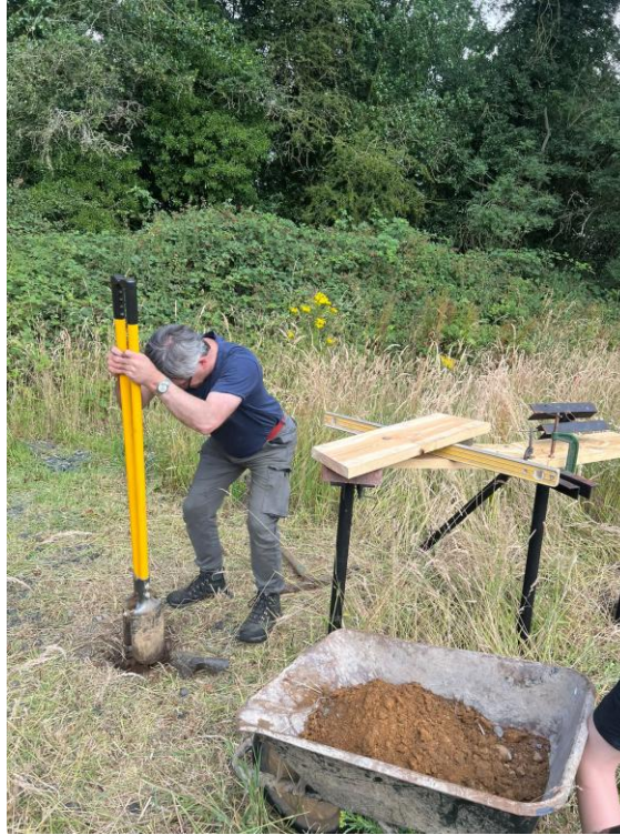
Ed dug out 2 more holes for garden rail posts.
