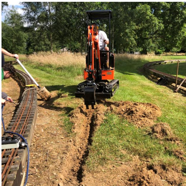
A narrow trench to re-bury the cable to the new signal position
