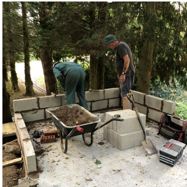
Peter Barnett helping with the mortar mix
