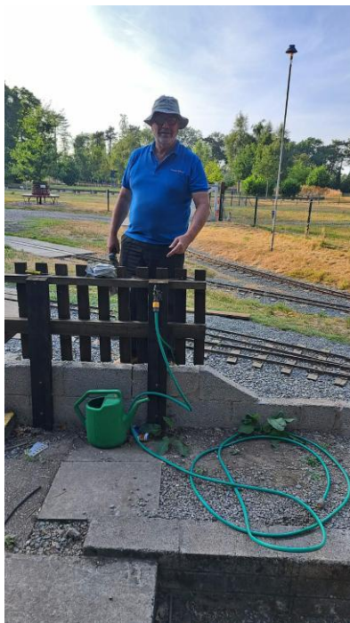
New tap installed near the shed
