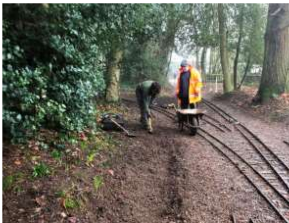
By the end of the session the formation has been dug out ready for washed ballast to go back in.
