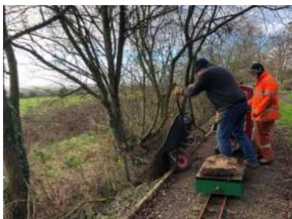
Unloading on the embankment to build this up
