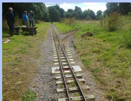
Points being put in to give us alternate routes.
