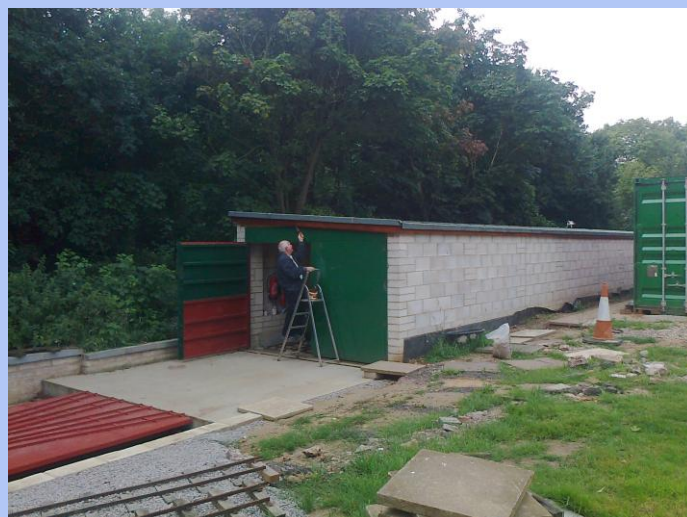
The late Brian Walton was finishing off the original roof of CS2 just 10 years ago!
