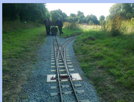
Points being put in to give us alternate routes.
