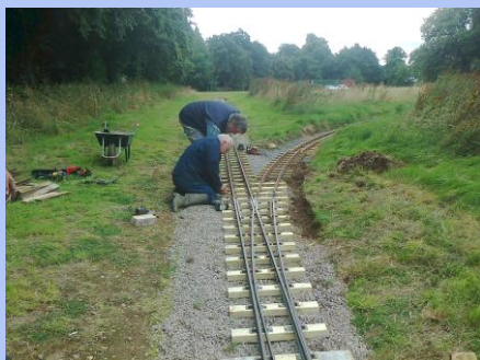
Points being put in to give us alternate routes.
