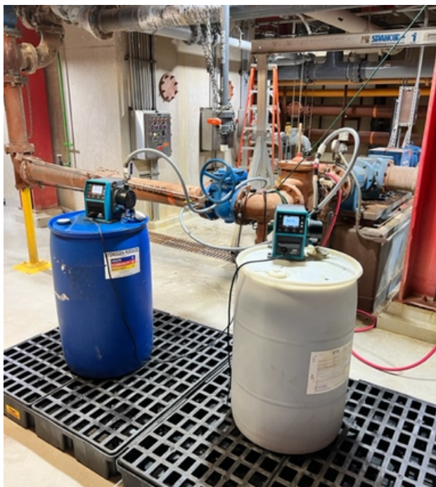
Picture 1: (Left) 50% H 2 O 2 and (Right) ETX catalyst temporary chemical injection system.
