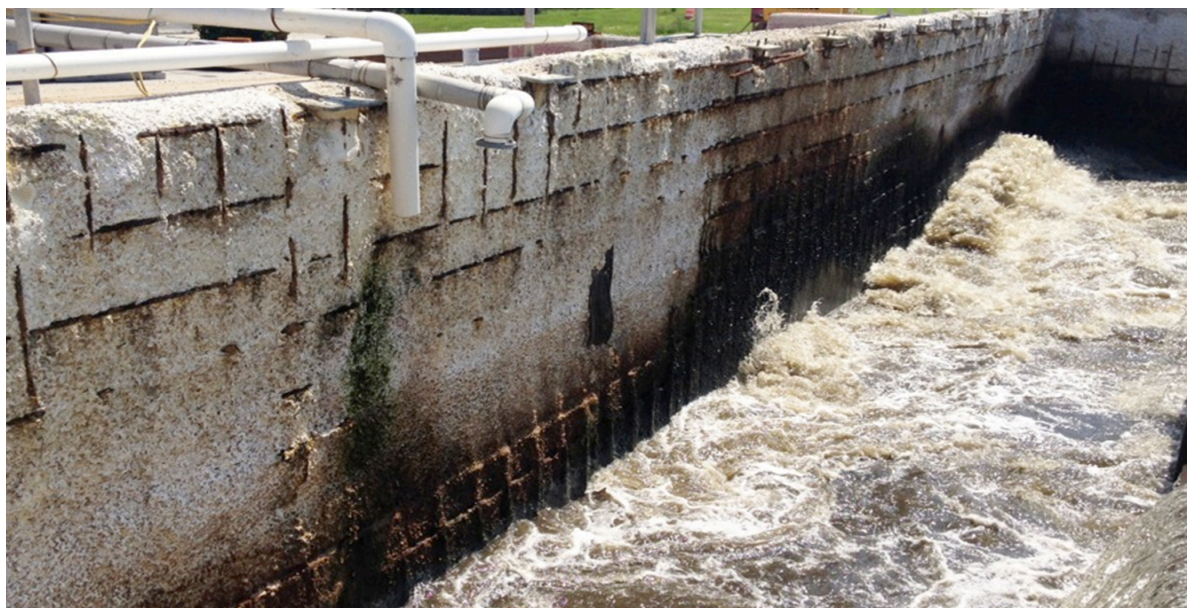
Image 3: The above image is from ~ Wastewater Treatment Plant. This location averaged 7.9 mg/L Total Sulfide, with peaks for 12.9 mg/L. At the time of this photo, the corroded facility seen above was only 7 years old, reduced to a barely functional state from H_2S Corrosion.
