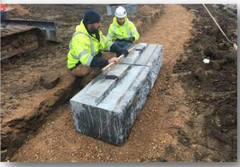
Walls should generally be built starting at the lowest elevation along the wall. However, if there are corners and/or abutting structures along the wall profile, these locations may be better places to start construction.
