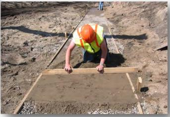
Be sure to examine and test any foundation soil that appears inadequate and may not meet the bearing requirements set forth in the engineered plans.
