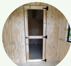
Feed Room Wall with Screen Door
