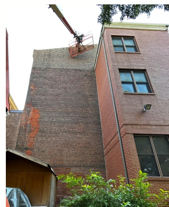
Picture left: Work has begun on repointing the terrace-facing brick wall to repair deteriorated mortar and protect the masonry from water damage.
