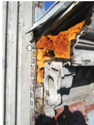
Crumbling cornice elements on the townhouse section of the GSP's building
