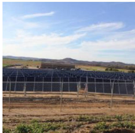
Riverland Energy Cooperative solar array
