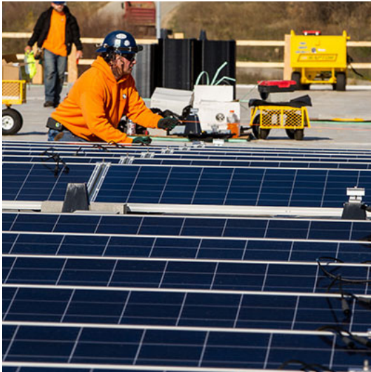
Pictured above: MGE Shared Solar under construction
