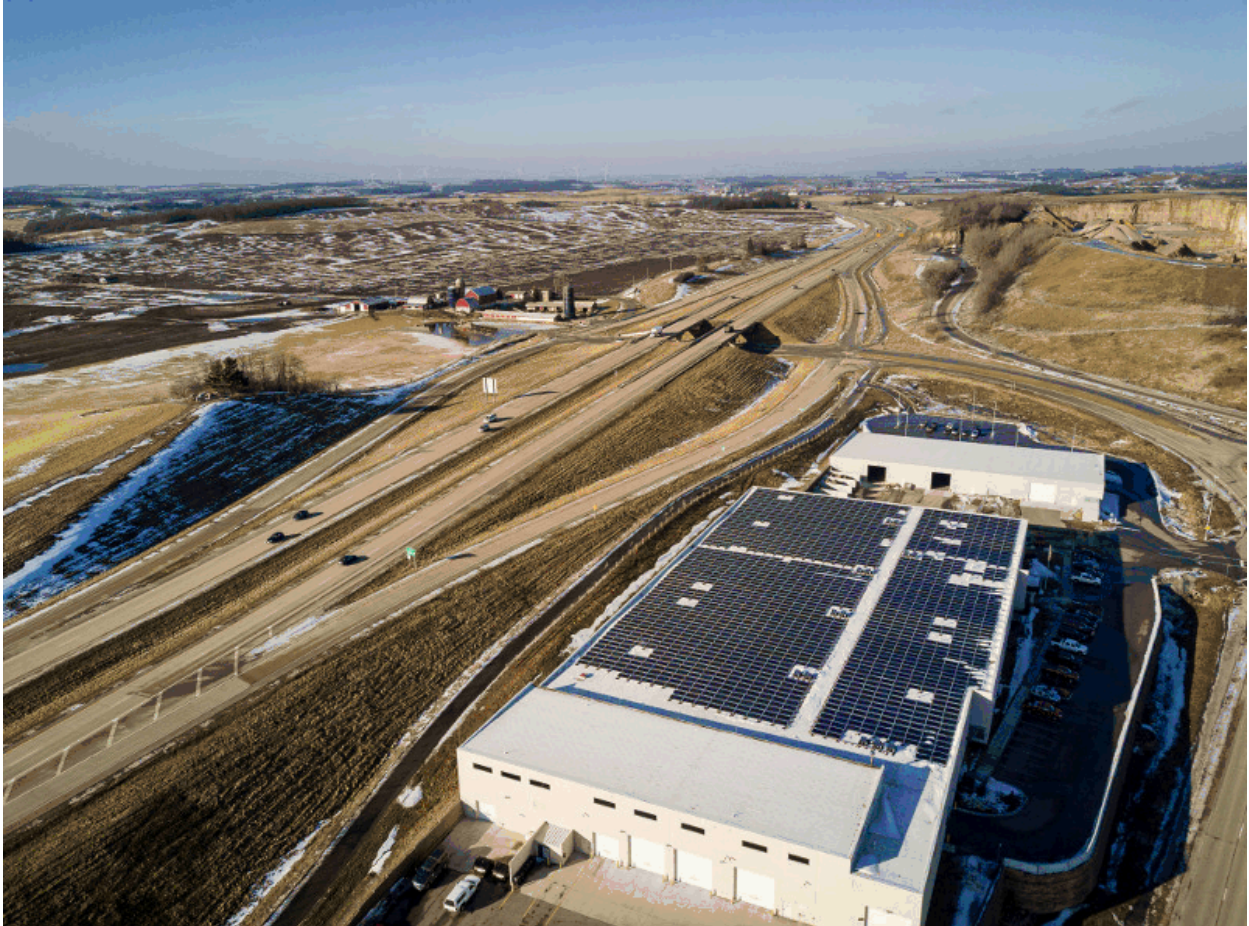
Pictured above: MGE Shared Solar on rooftop of the MOC
