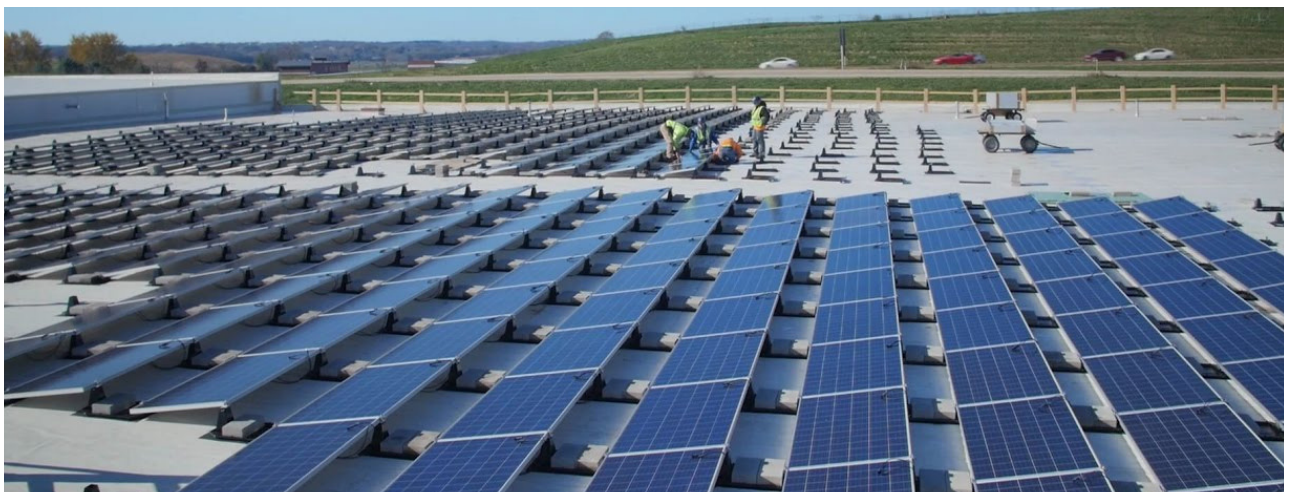
Pictured above: MGE Shared Solar under construction
