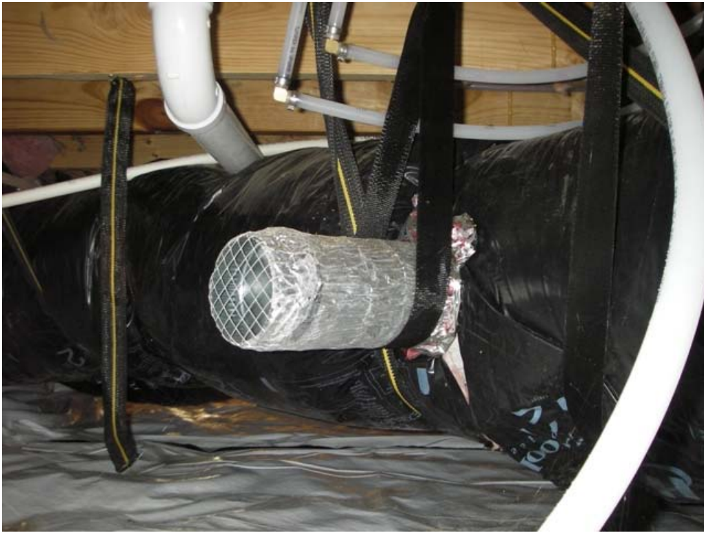
Figure 11. Baton Rouge closed crawl space drying mechanism.
