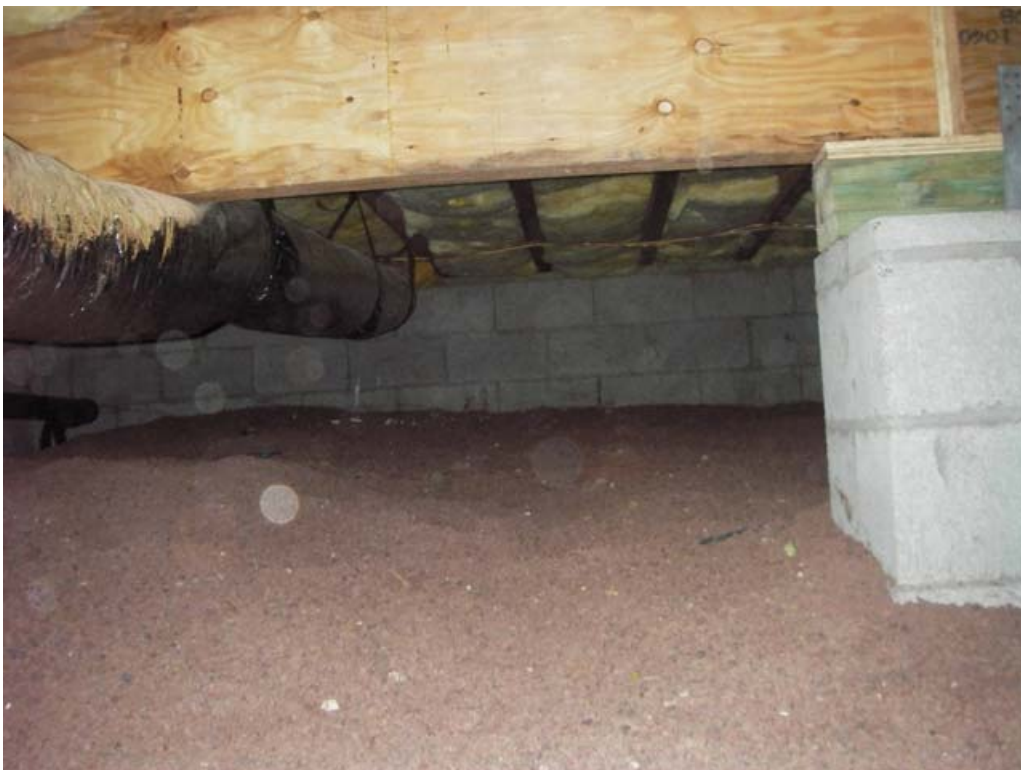
Figure 18. Flagstaff vented crawl space.
