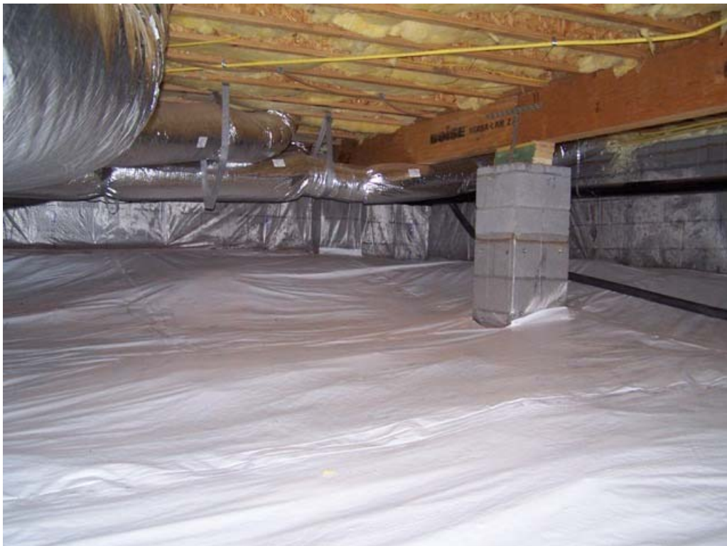
Figure 20. Flagstaff finished floor-insulated closed crawl space.
