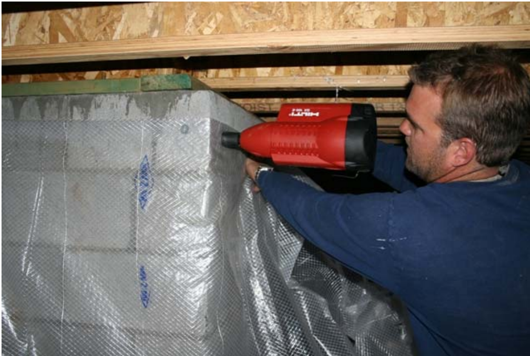
Figure 19. Flagstaff wall liner installation.
