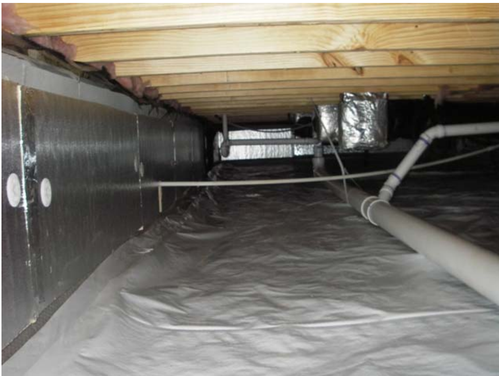
Figure 10. Baton Rouge finished wall-insulated closed crawl space.
