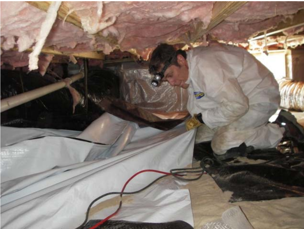
Figure 8. Baton Rouge liner system installation.
