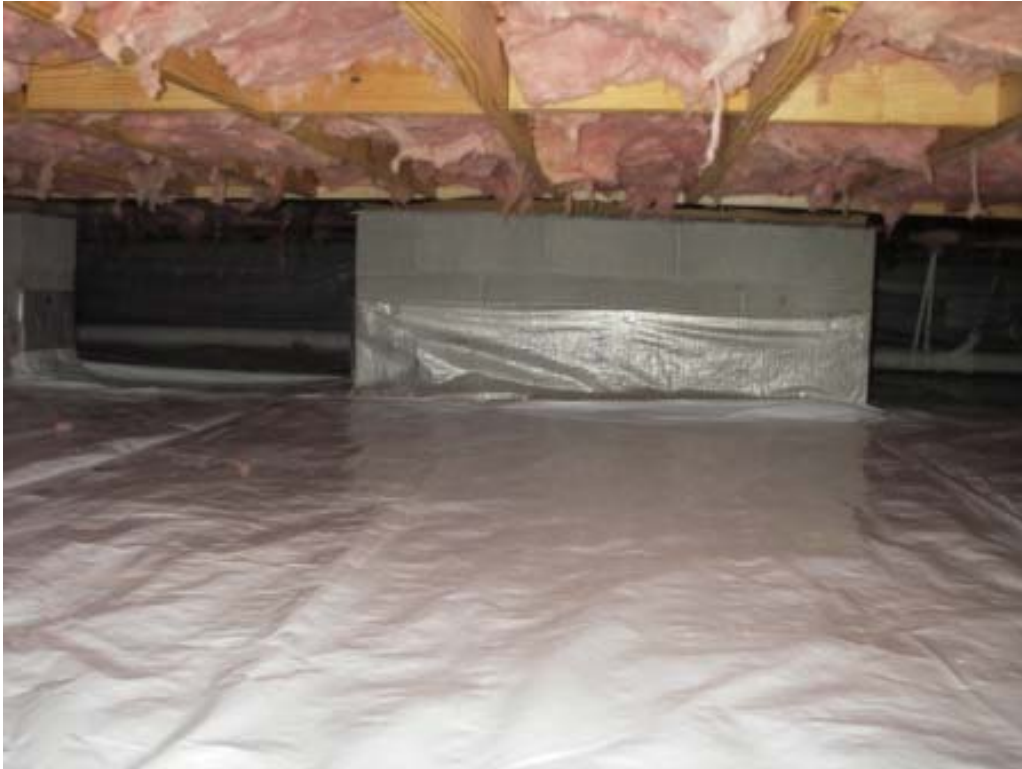
Figure 9. Baton Rouge finished floor-insulated closed crawl space.
