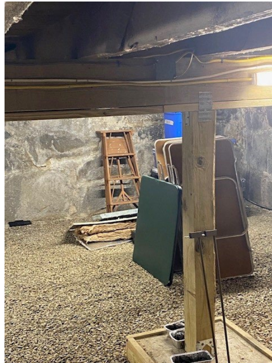
Figure #2. – ABM Library Sagging Basement Beam
