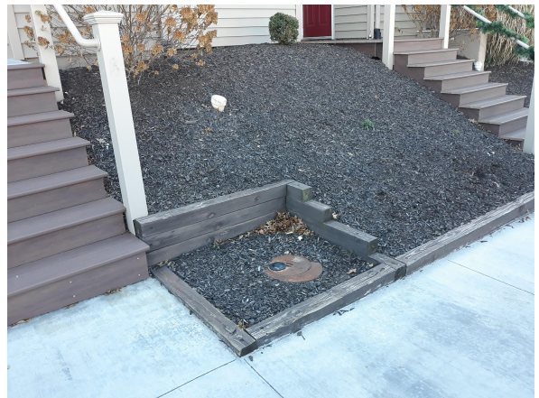
Timber/wood retaining wall
