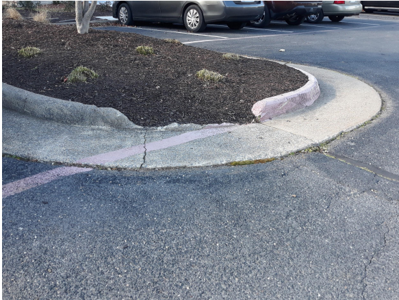
Damaged curbing
