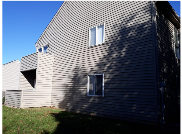
Side of building
