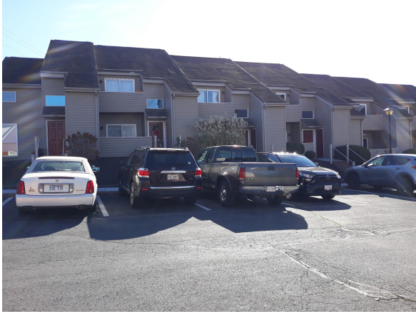
Front of building
