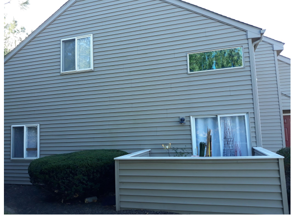
Right side of building
