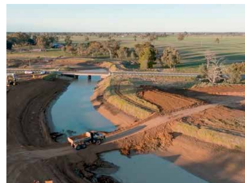
Extensive channel remediation works underway.
