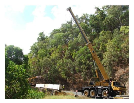
The Grove was no longer required and the 20T Franna was re-positioned to lift the front end of the bridge girder. It was attached to the 36T set of 2-legged chains with a 2.5m radius where the crane was good for 13.9T. The truck reversed under the girder and it was reattached.
