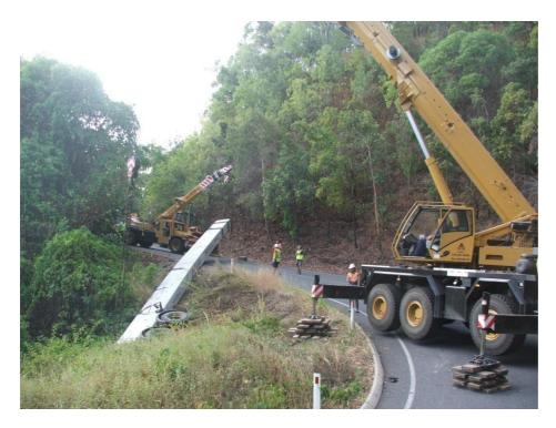
One option to lighten the load was to disconnect the dolly from the girder but after consultation between the dogger, crane driver and client it was decided the risk was too high to send someone into the gully to disconnect the girder from the dolly.
