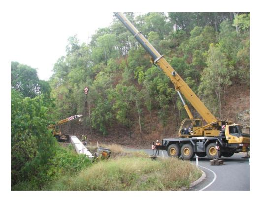
The estimated weight applied to lift the lower end of the girder and dolly by the Grove was 4.5-5T at a radius of 13m as the upper part of the girder was acting as a counter weight. The machine was good for 8.2T at this point.
