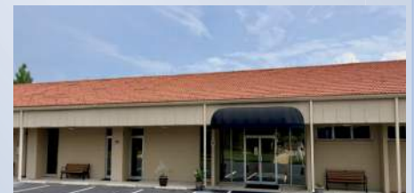
Education Bldg. sealed, sided & new gutters
