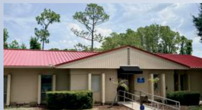
New metal roof and siding
