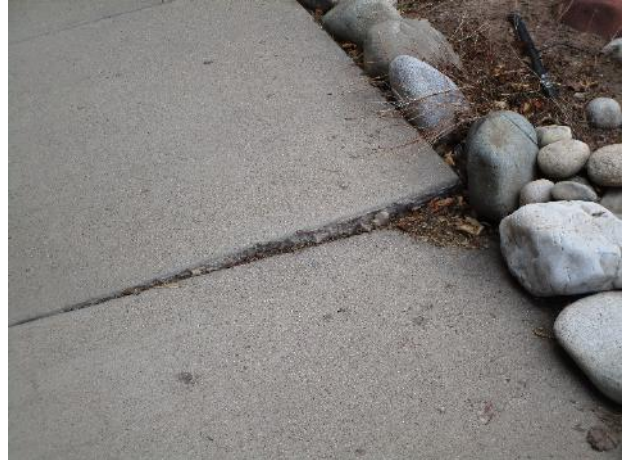
Concrete settlement at Building 255-258
