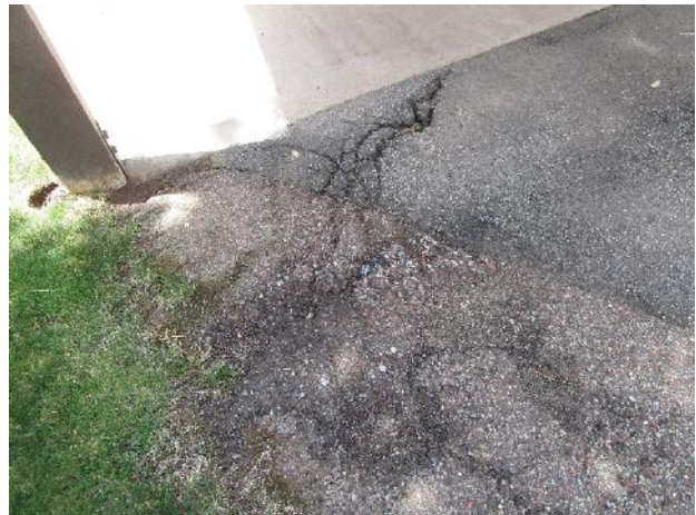
Pavement cracks and deterioration at Building 119-125
