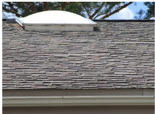
Shingle lift and sheathing deflection at Building 115-118
