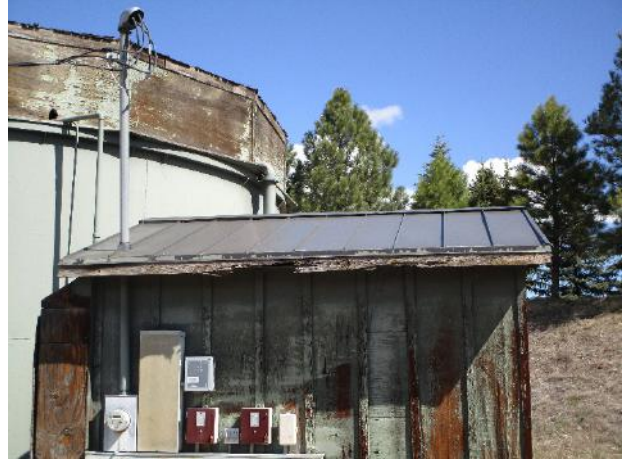
Siding finish deterioration and damage
