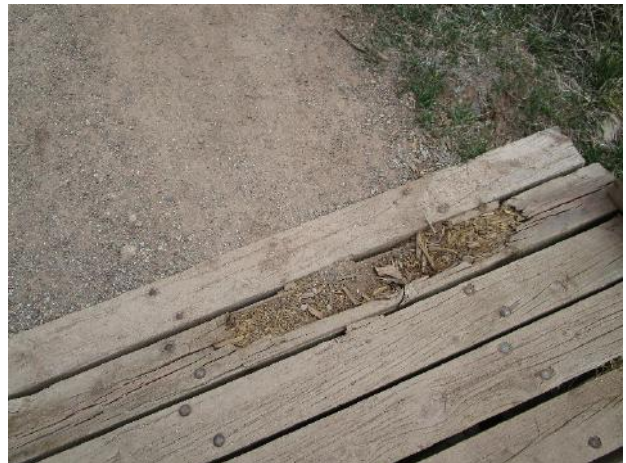
Wood rot and split deck boards
