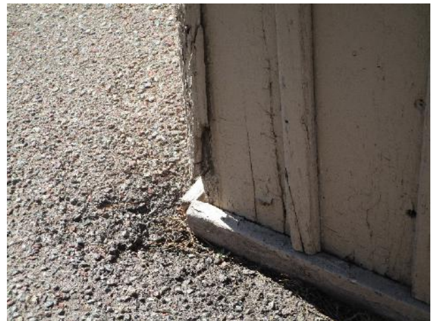
Siding damage and finish deterioration at the Golf Shop
