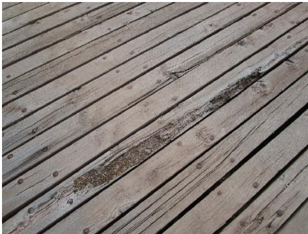
Wood rot and split deck boards
