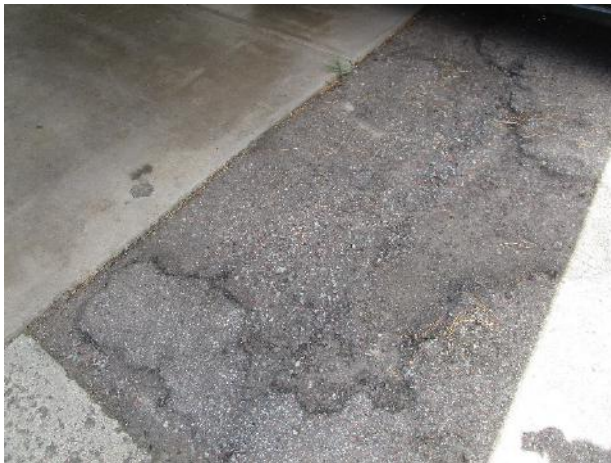
Pavement deterioration at Building 119-125
