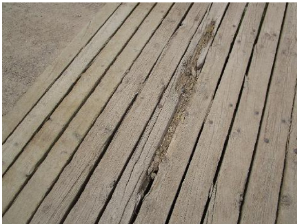
Wood rot and split deck boards
