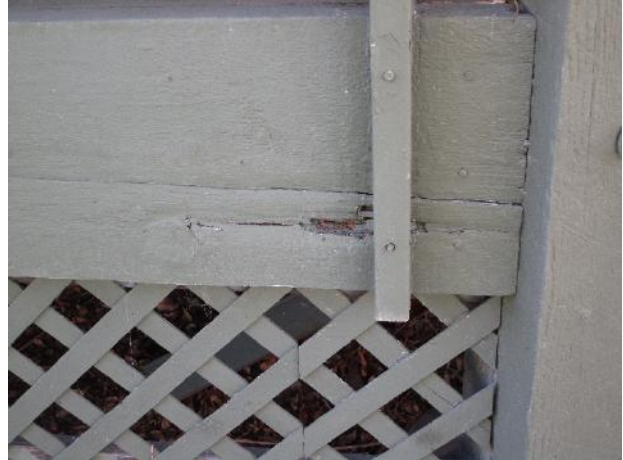
Deck frame split wood and wood rot
