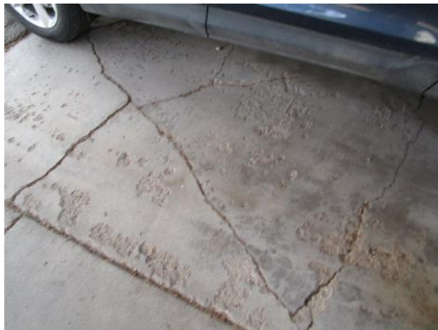
Concrete cracks and concrete spall at Building 103-113
