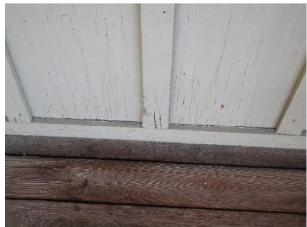
Siding damage and finish deterioration at the Office Building
