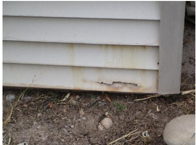
Siding damage at Building 283-286
