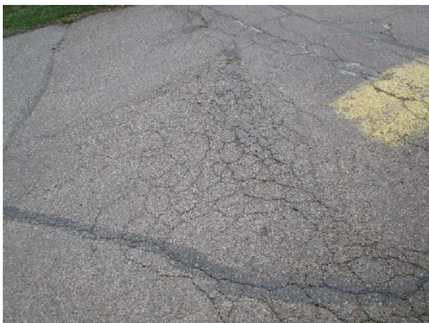
Pavement cracks at Stagecoach Lane
