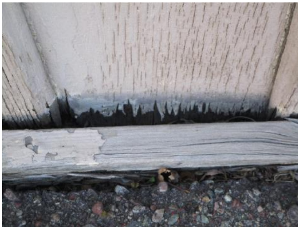
Siding damage and finish deterioration at the Golf Shop
