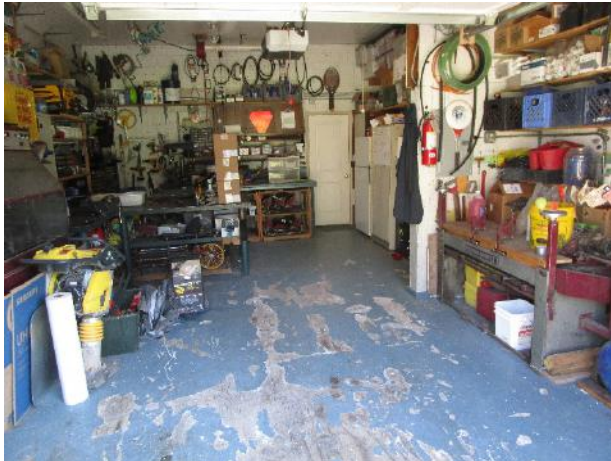
Golf shop common interior; Floor finish deterioration
