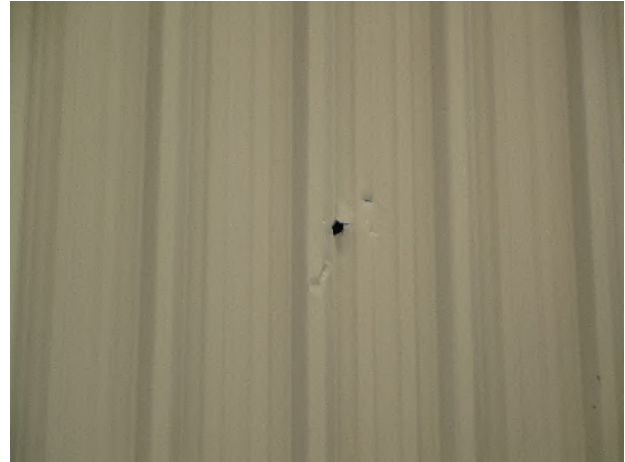
Siding damage
