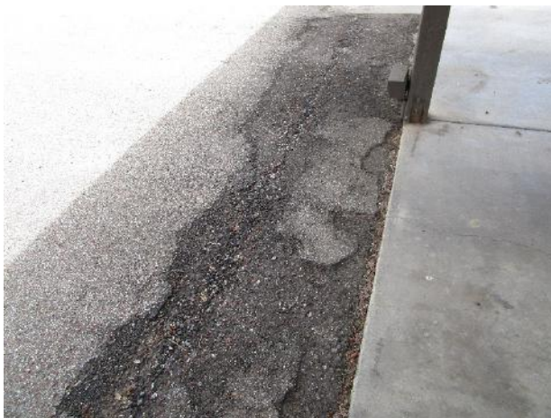
Pavement deterioration at Building 135-138
