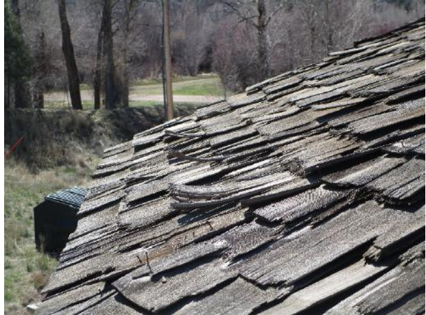
Damaged and curled shingles
