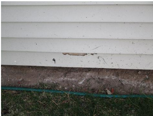
Siding damage at Building 115-118
