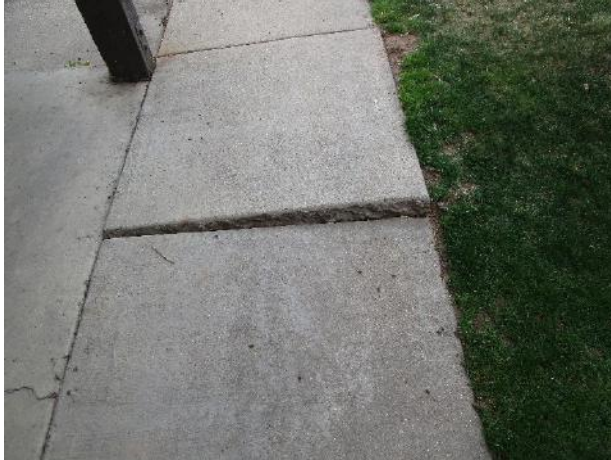
Concrete settlement at Building 275-281
