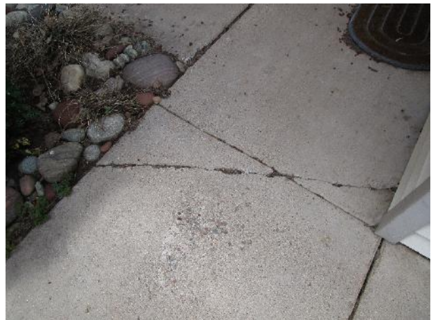
Concrete cracks and concrete spall at Building 135-138
