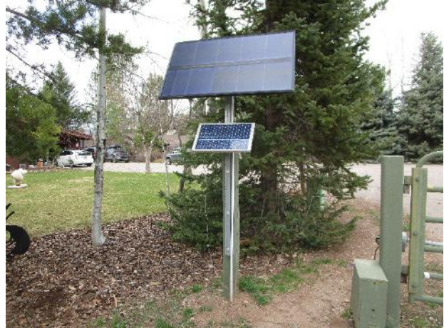
Gate operator and solar panel
