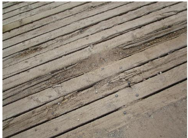
Wood rot and split deck boards
