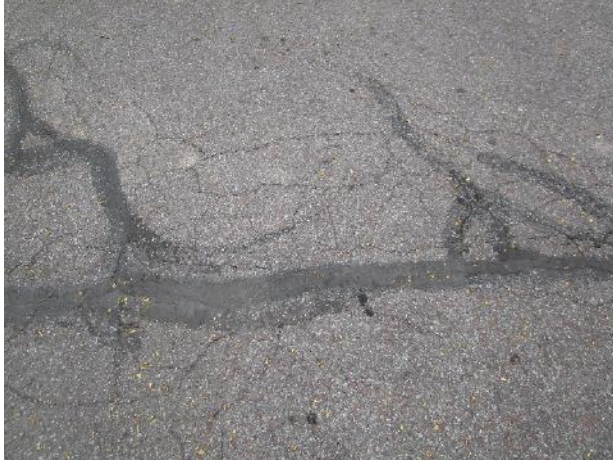
Pavement cracks at Stagecoach Drive
