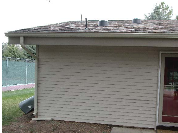
Gutter and downspout assembly
