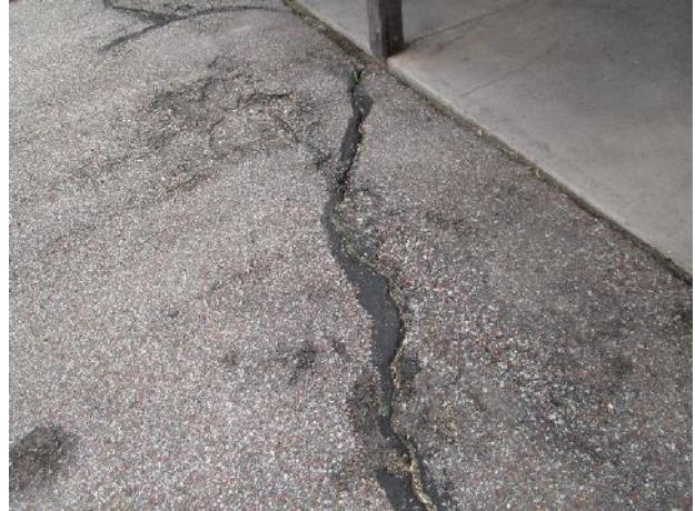
Pavement cracks at Building 271-274
