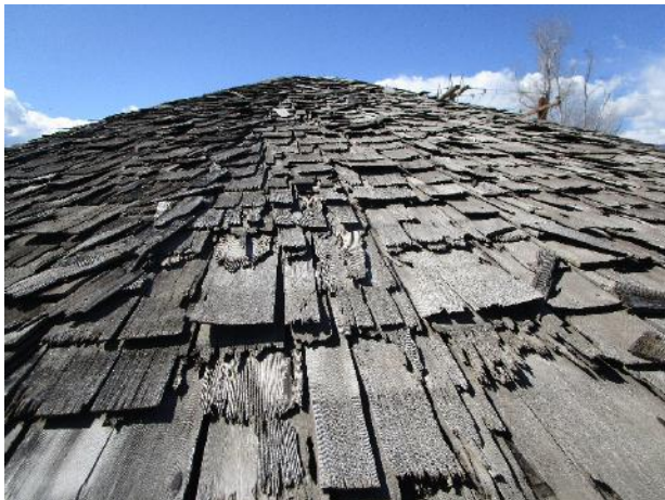
Damaged and curled shingles
