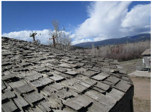
Damaged and curled shingles
