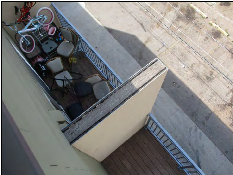
128: Missing wall flashing at balcony wall (Immediate Repair)
