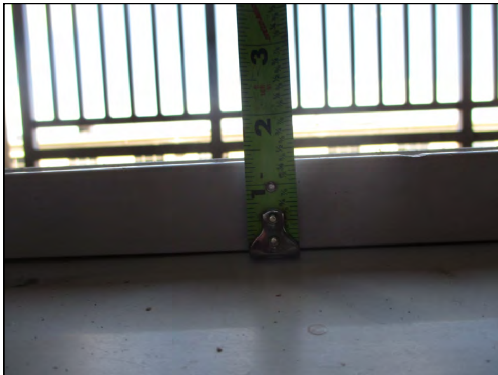
142: Reconfigure thresholds at patio sliding glass doors (Immediate Repair)
