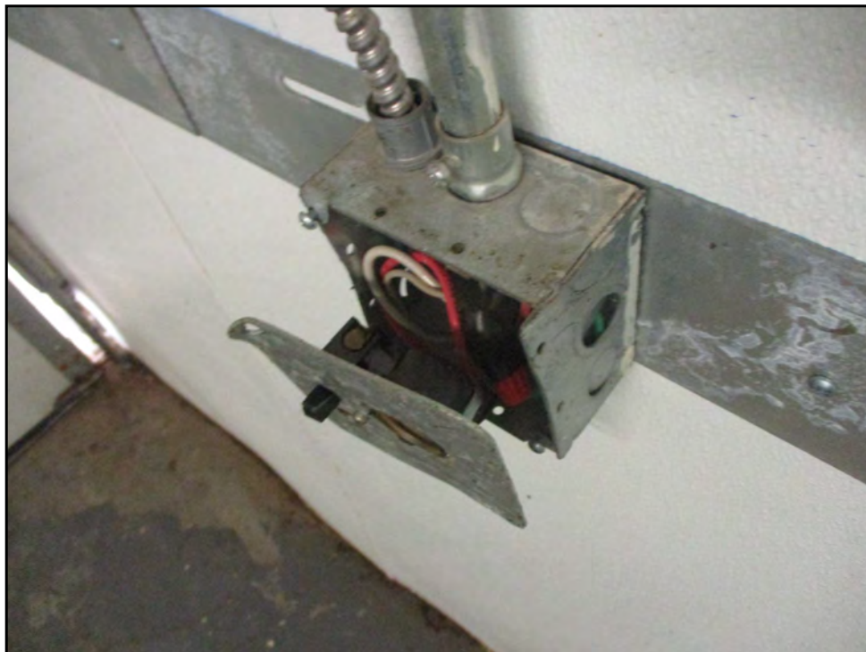
132: Exposed wiring at junction box within trash room (Immediate Repair)
