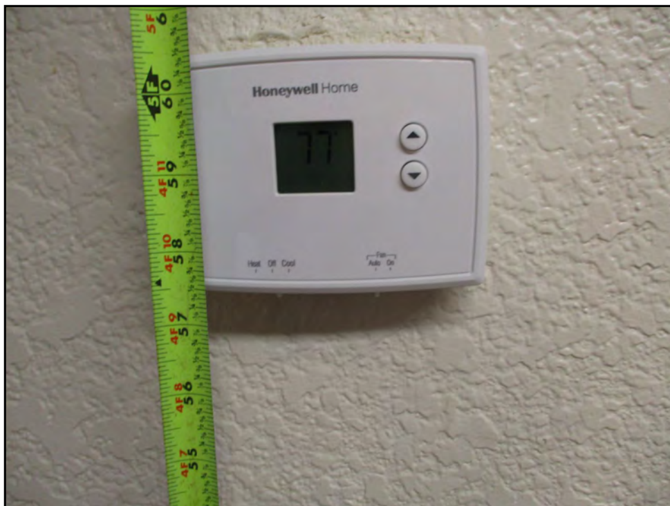
148: Lower thermostats (Immediate Repair)
