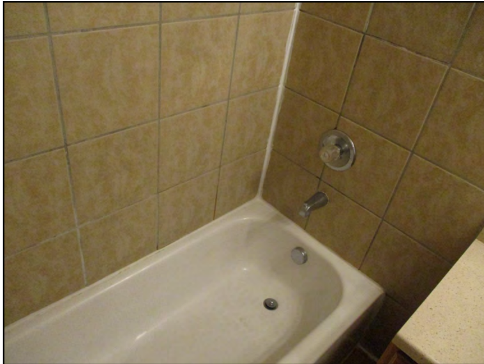
115: Interior dwelling unit
