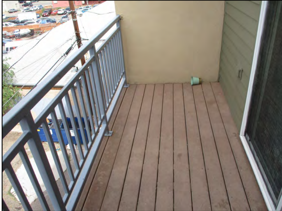
113: Interior dwelling unit
