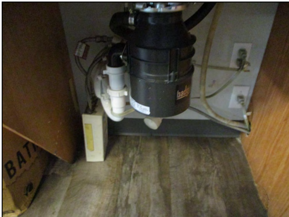
152: Install scald and abrasion protection at common kitchen sink (Immediate Repair)
