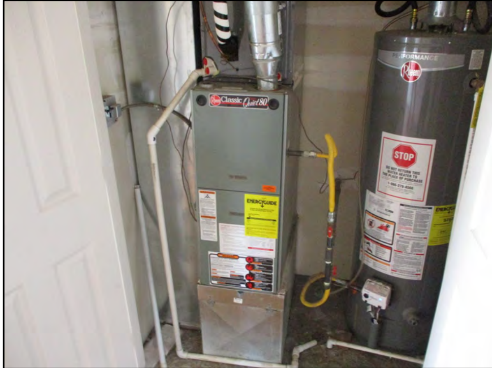
109: Interior dwelling unit
