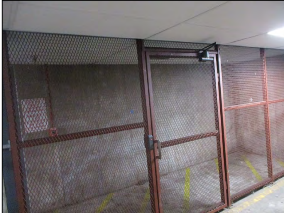
47: Secured stairwell entrance at parking garage
