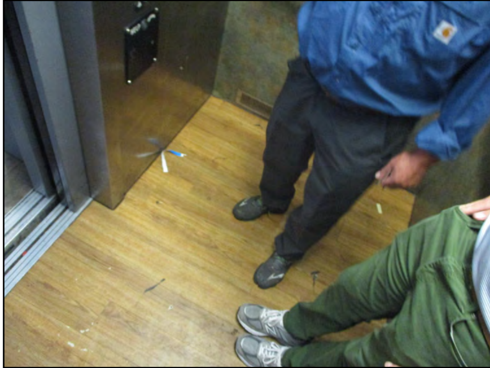
137: Refurbish elevator cab interior (Immediate Repair)
