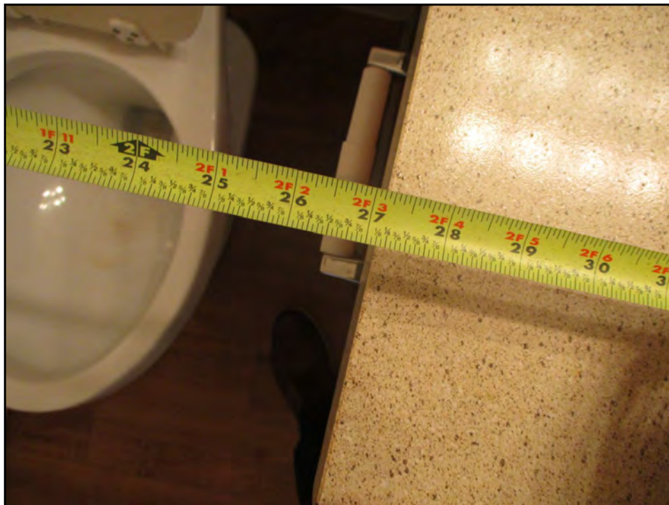
170: Less than 33-inches between wall and vanity at toilet in select floorplan types (Immediate Repair)
