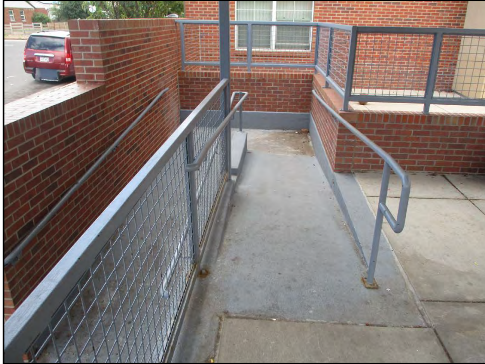
7: Ramp at primary pedestrian entrance
