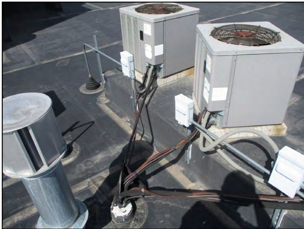
136: Replace A/C line set insulation (Immediate Repair)
