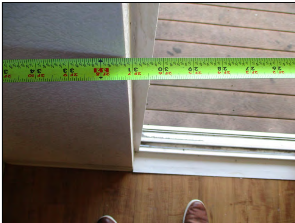
144: Sliding glass door opening less than 32-inches (Immediate Repair)
