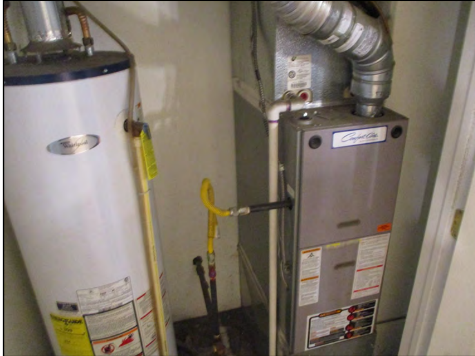
61: Interior dwelling unit
