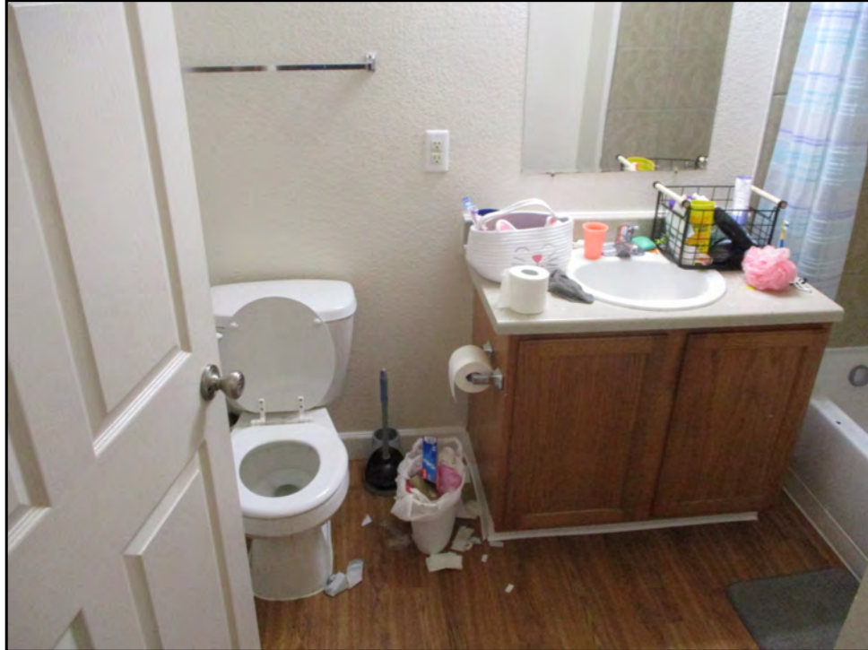
139: Replace bathroom vanity cabinets (Immediate Repair)
