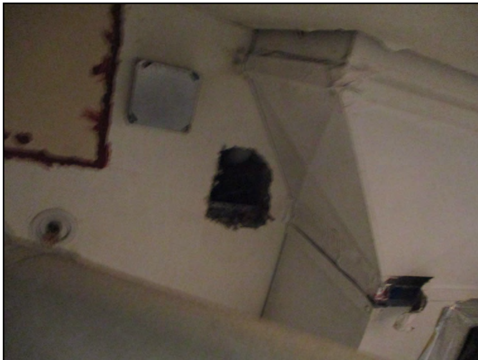
172: Unsealed thru-wall penetrations at unit mechanical closets (Immediate Repair)
