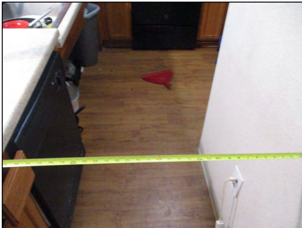
160: Missing compliant maneuvering space within galley kitchens in Type J floorplans (Immediate Repair)
