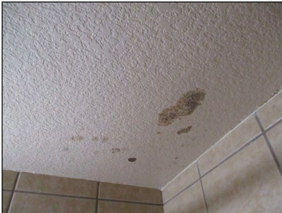
138: Water damage at bathroom ceiling Unit 101 (Immediate Repair)
