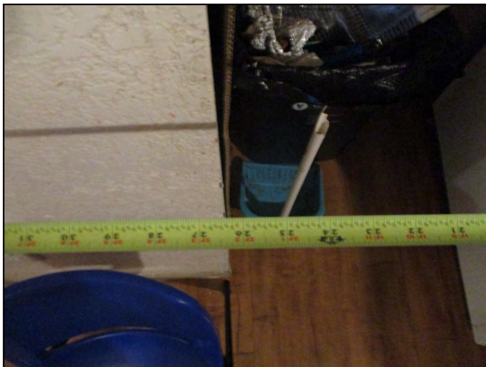
168: Missing compliant approach to refrigerator within Type C units (Immediate Repair)
