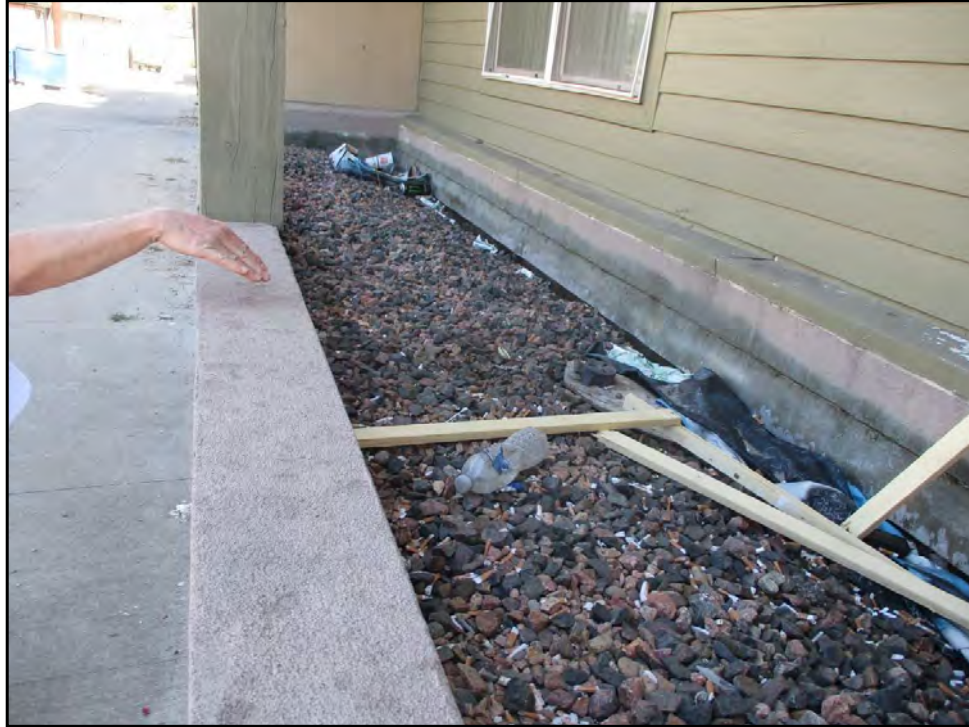
135: Address water penetration around planter boxes (Immediate Repair)
