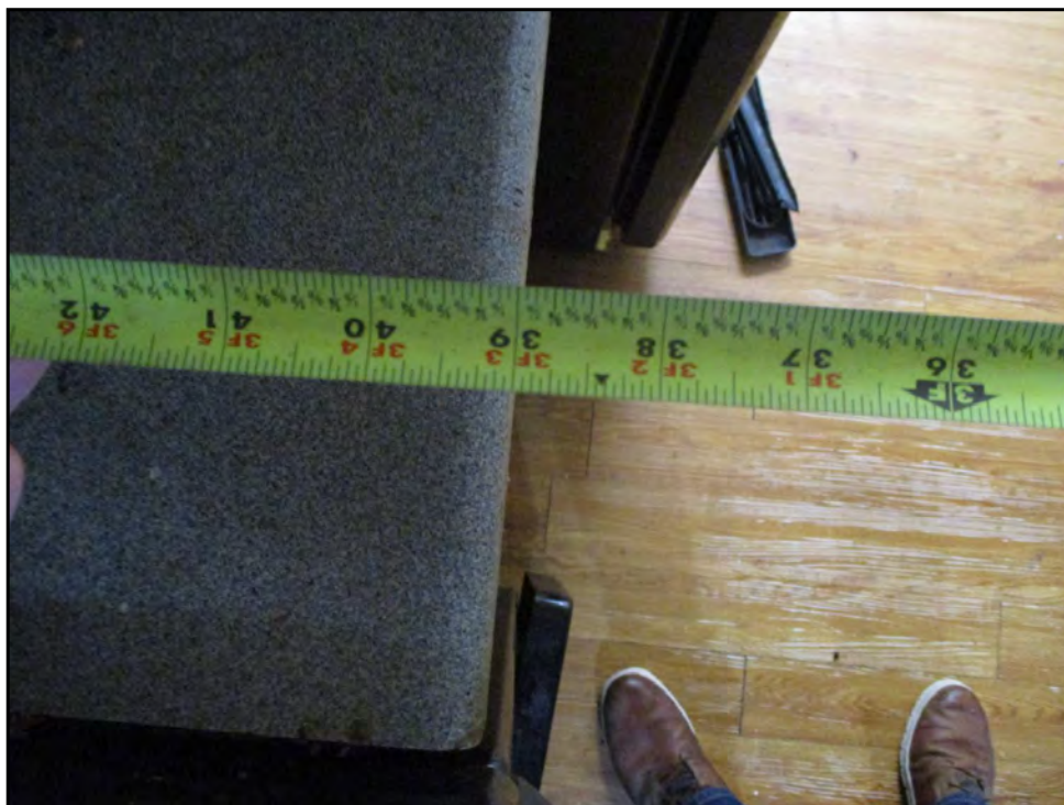
164: Missing compliant maneuvering space within galley kitchens in Type K units (Immediate Repair)
