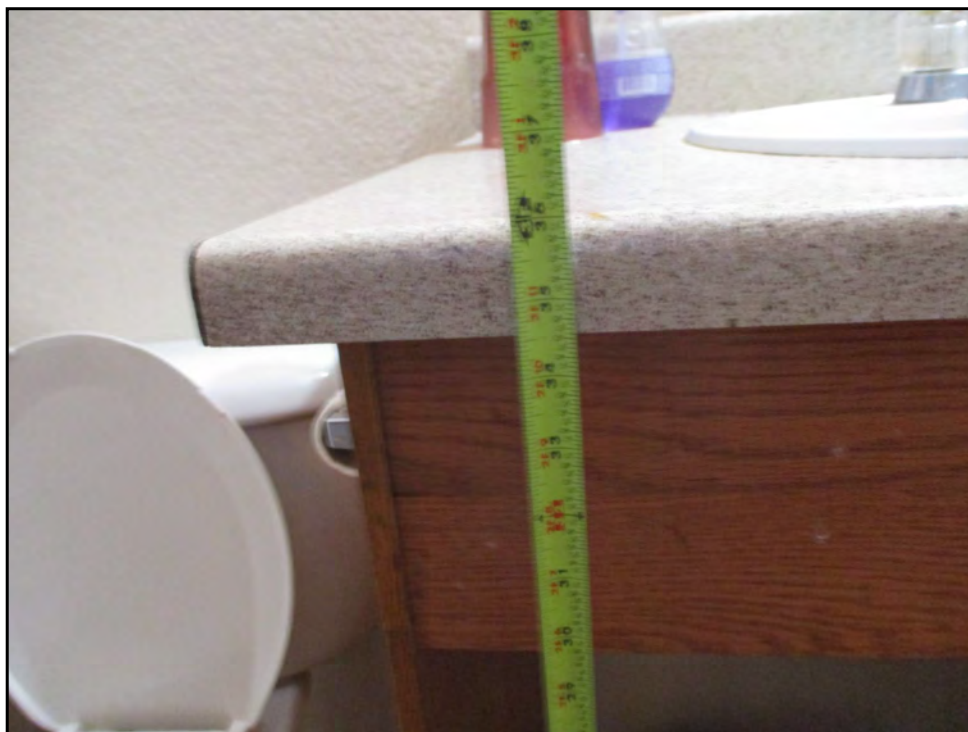
162: Bathroom sink higher than 34-inches in HC unit 101 (Immediate Repair)
