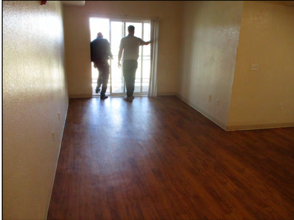
77: Interior dwelling unit
