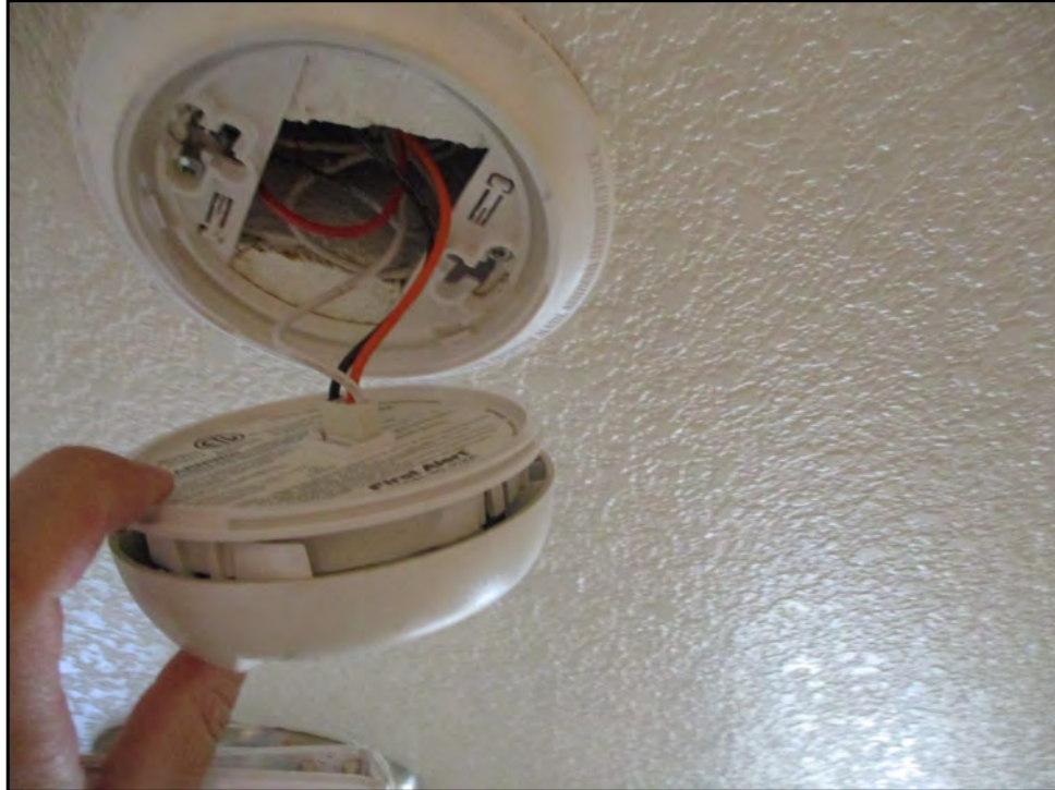
63: Interior dwelling unit
