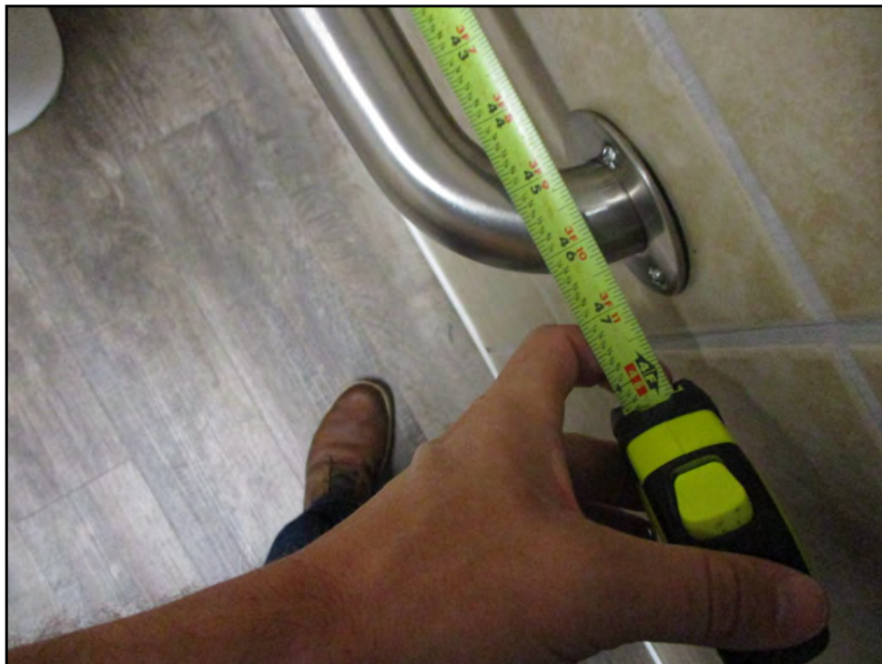
150: Non-compliant toilet grab bar at common restroom (Immediate Repair)
