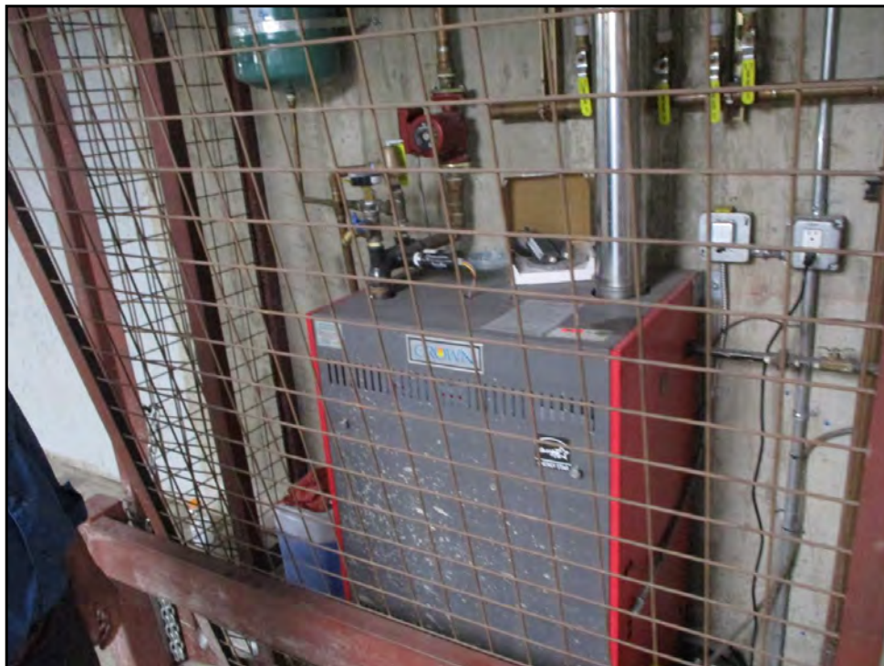
50: Boiler for fire sprinkler system
