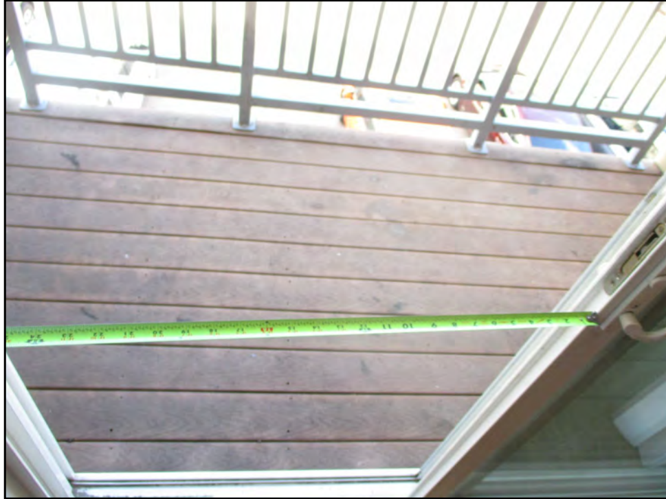
87: Interior dwelling unit
