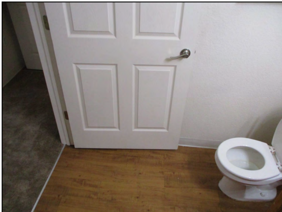
154: Reverse door swing in master bath unit type G (Immediate Repair)
