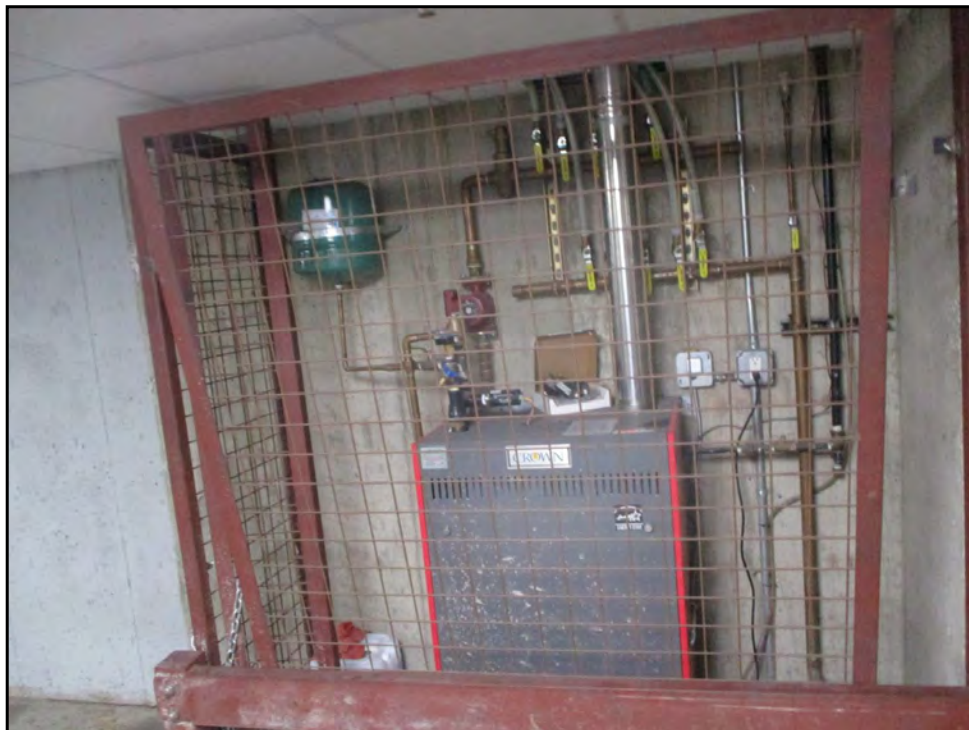
120: Damaged security screen around sprinkler boiler (Immediate Repair)
