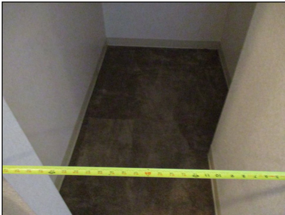
156: Master closet in Type J less than 32-inch wide openings (Immediate Repair)
