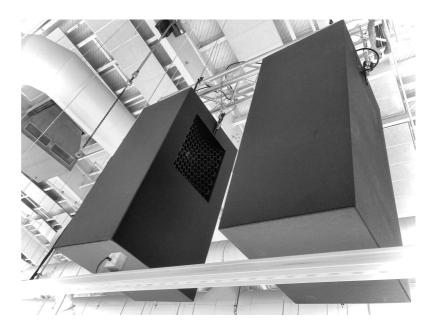
Dual XQ48 subwoofer flown array pictured from below in an arena system. Multiple subwoofers facing one point create a virtual single omni-directional source and even 360 degree distribution of low frequencies when placed in the center of the arena ceiling.
