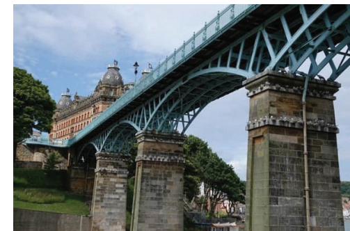
Spa Bridge - Scarborough Photo: Nick Addey
