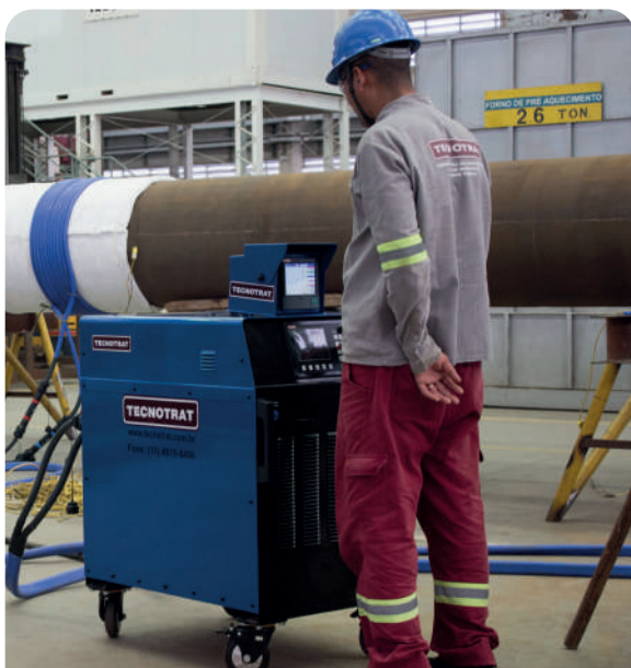
Post Weld Heat Treatment Induction Heating 30" pipe / 44 mm thickness
