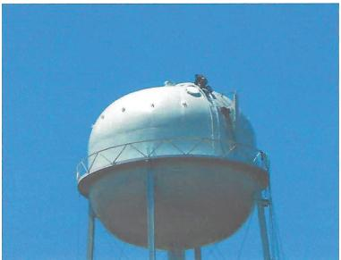
whereas irregular maintenance can greatly decrease tank life. A tank maintenance plan puts routine activities such as cleaning, painting and repair on a schedule. Best of all, the tank maintenance company knows exactly what a tank needs and when it will need it. It's important to make sure you know all the costs involved in a maintenance contract when inspections, maintenance and painting occur. A good contract includes no surprises.
