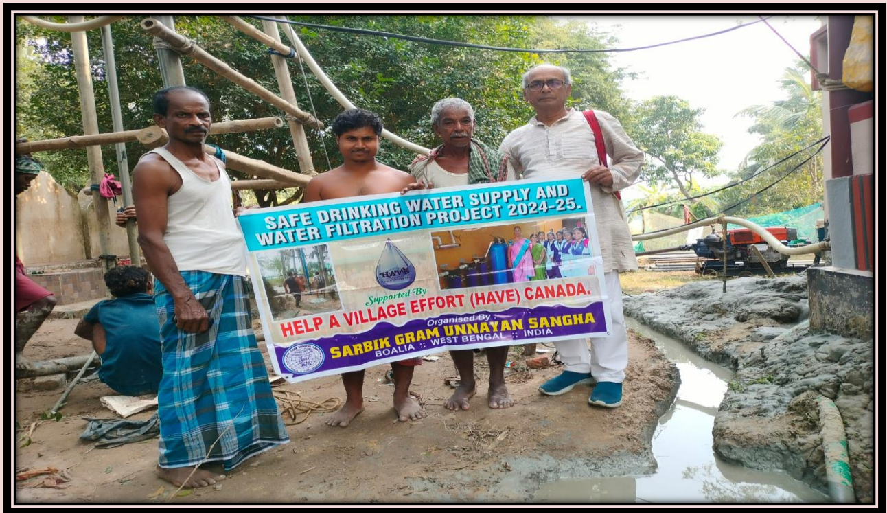
Installation of Community Water Supply Well at Jamua Sankarpur village
