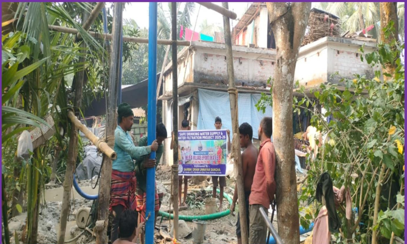
Installation of community water supply wells
